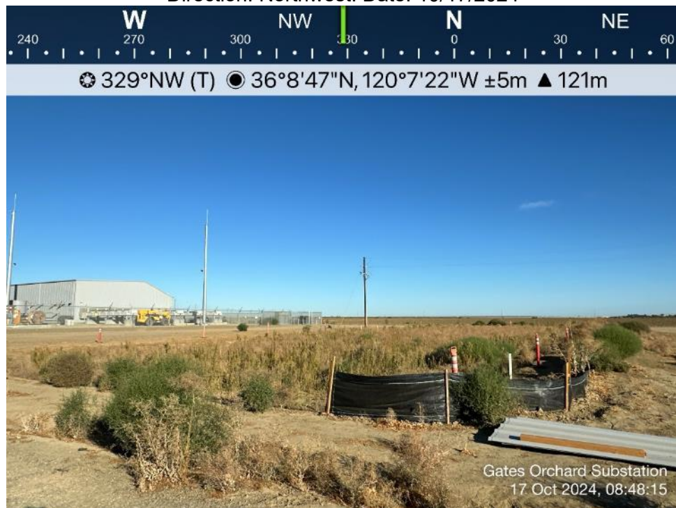
Photo 2. View of retention basin with silt fence. Direction: Northwest. Date: 10/17/2024
