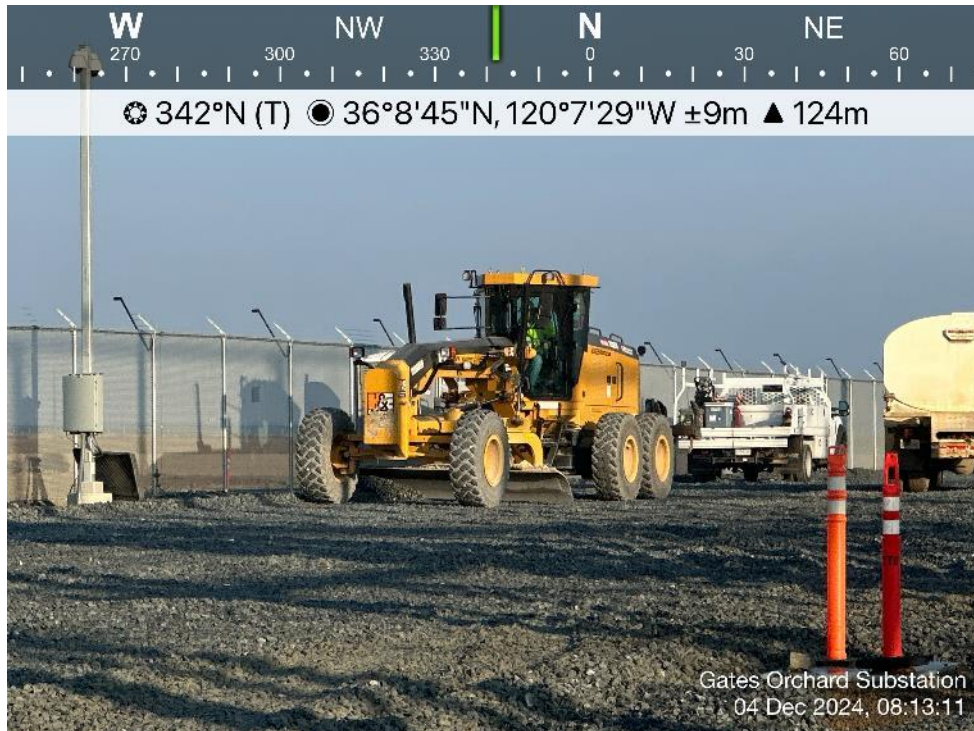
Photo 18. View of grader spreading rock inside the substation. Direction: North. Date: 12/4/2024
