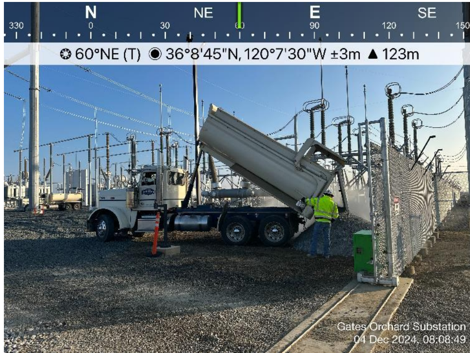
Photo 17. View of rock delivery. Direction: Northeast. Date: 12/4/2024
