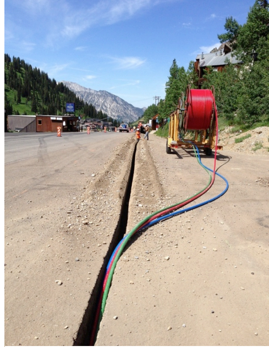
Figure 2.4-22. Saw Cut and Conduit Install
