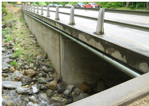
Figure 2.4-25. Completed Bridge Hang
