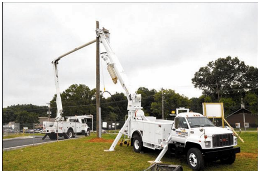
Figure 2.4-20. Installing New Pole
