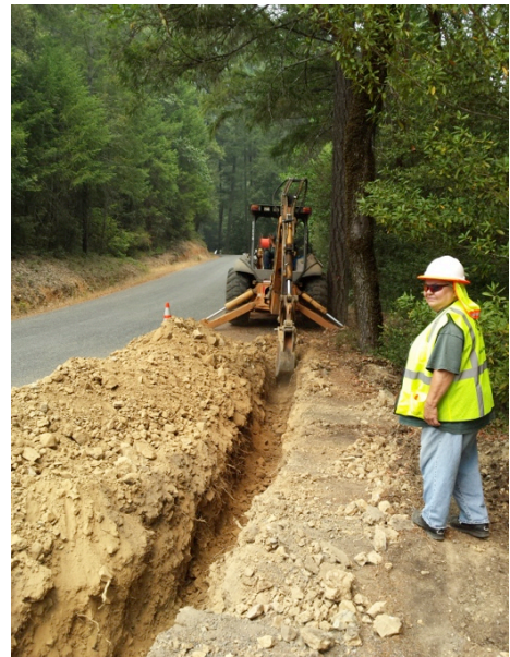
Figure 2.4-21. Roadside Trenching
