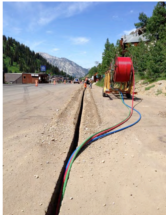
Figure 2.4-22. Saw Cut and Conduit Install
