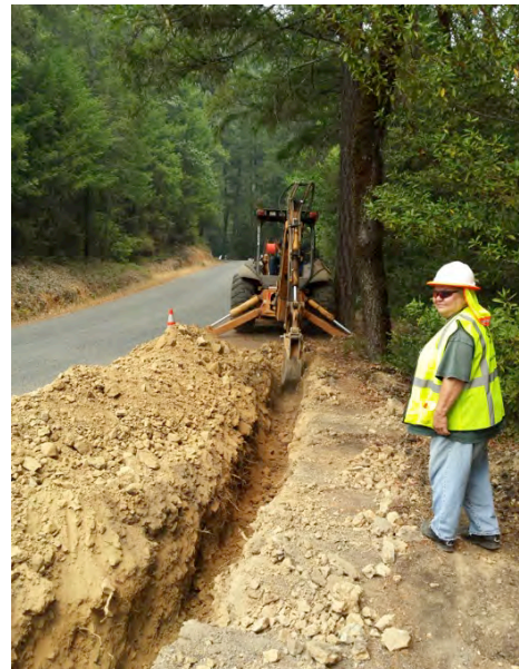
Figure 2.4-21. Roadside Trenching
