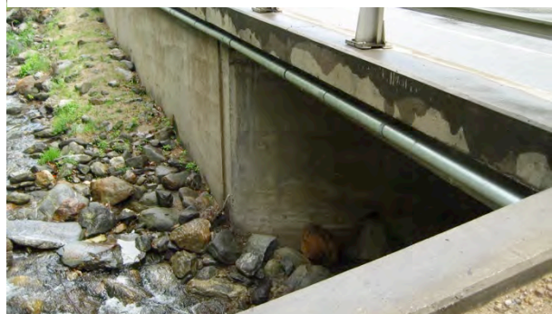
Figure 2.4-25. Completed Bridge Hang
