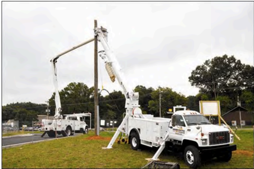
Figure 2.4-20. Installing New Pole
