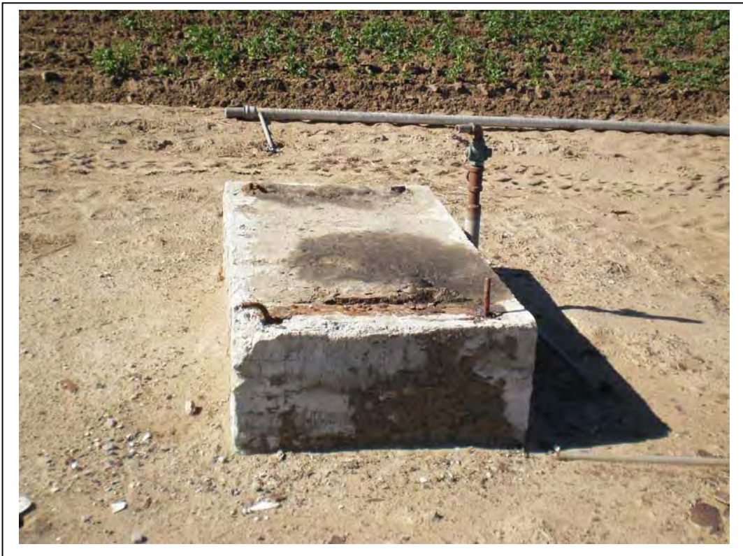
(4). Concrete Slab and Natural Gas Line
