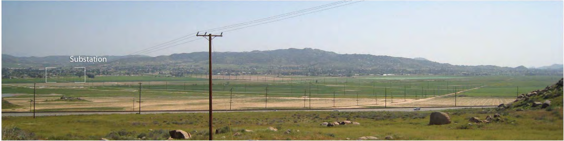
KOP 1 - Simulated View from Bernasconi Road near entrance to Lake Perris State Recreation Area, looking southeast
