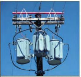
FIGURE 6.24: A pipe mounted above the conductors can be used as a nest discourager on distribution poles with insulators mounted on the crossarm. The use of triangles is cautioned against, as they may aid in the accumulation of nesting material. This design may pose an electrocution risk if exposed equipment and conductors are not covered or adequately spaced.
