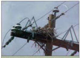
FIGURE 6.25: Red-tailed hawk nest on pole with triangle perch discouragers.
