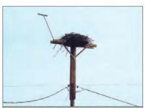
FIGURE 6.11: A nest platform built atop a pole using crossarms to extend the platform above the conductors. This design also includes an optional elevated perch to attract ospreys. The perch should be perpendicular to the prevailing wind.
