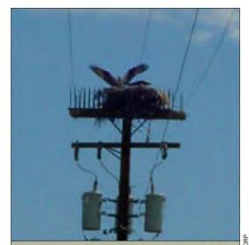
FIGURE 6.27: Osprey nest on pole with plastic spikes.
