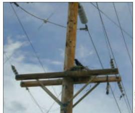
FIGURE 6.6: Common raven nest on distribution underbuild of transmission structure.
