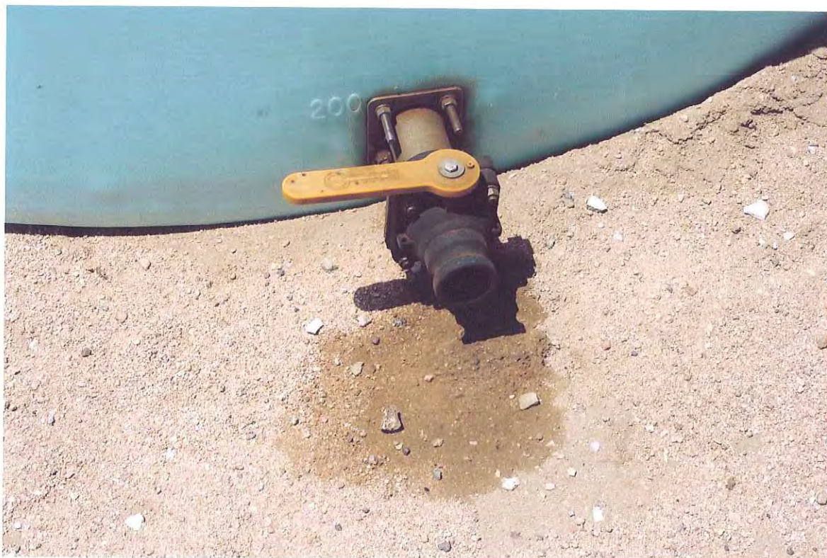
Photo #8 – Soil stain underneath valve on tank.
