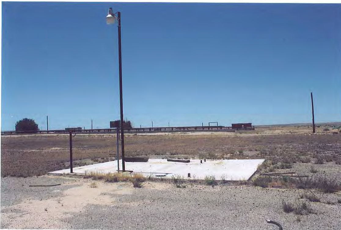
Photo #4 – APN 0490 121 42 – Concrete slab, possible location of AST's that were removed.
