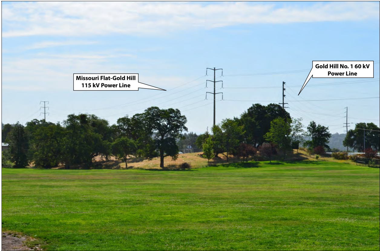
Existing View from McAuliffe Park looking southeast
