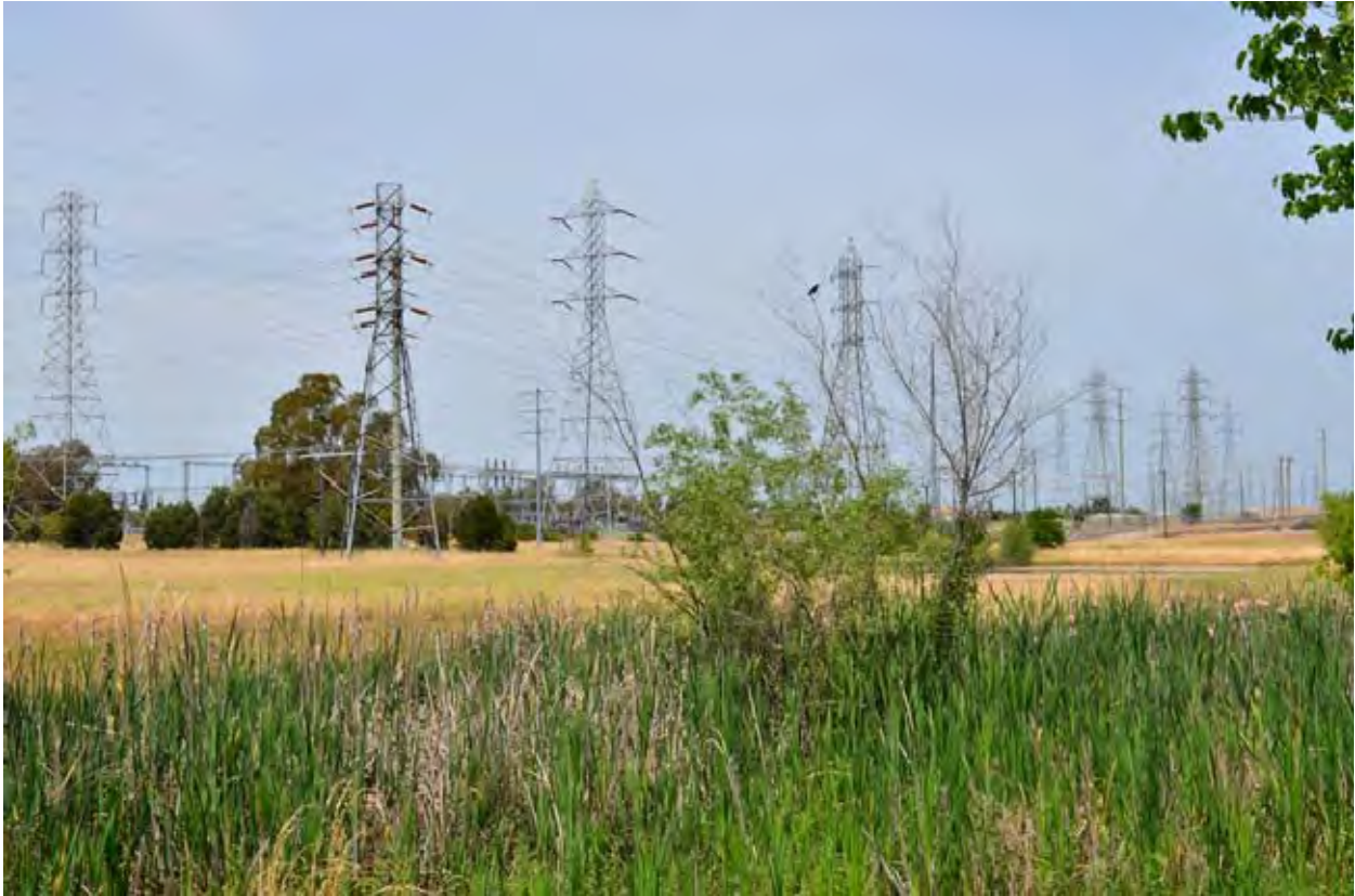
Photograph 17: View from Kemp Community Park looking northwest toward Gold Hill Substation (KOP 17). The Missouri-Flat-Gold-Hill Tower Line includes the steel lattice tower second from the right. Several other tower lines are also visible, including tower lines owned by the Sacramento Municipal Utilities District (SMUD) as well as a SMUD substation.
