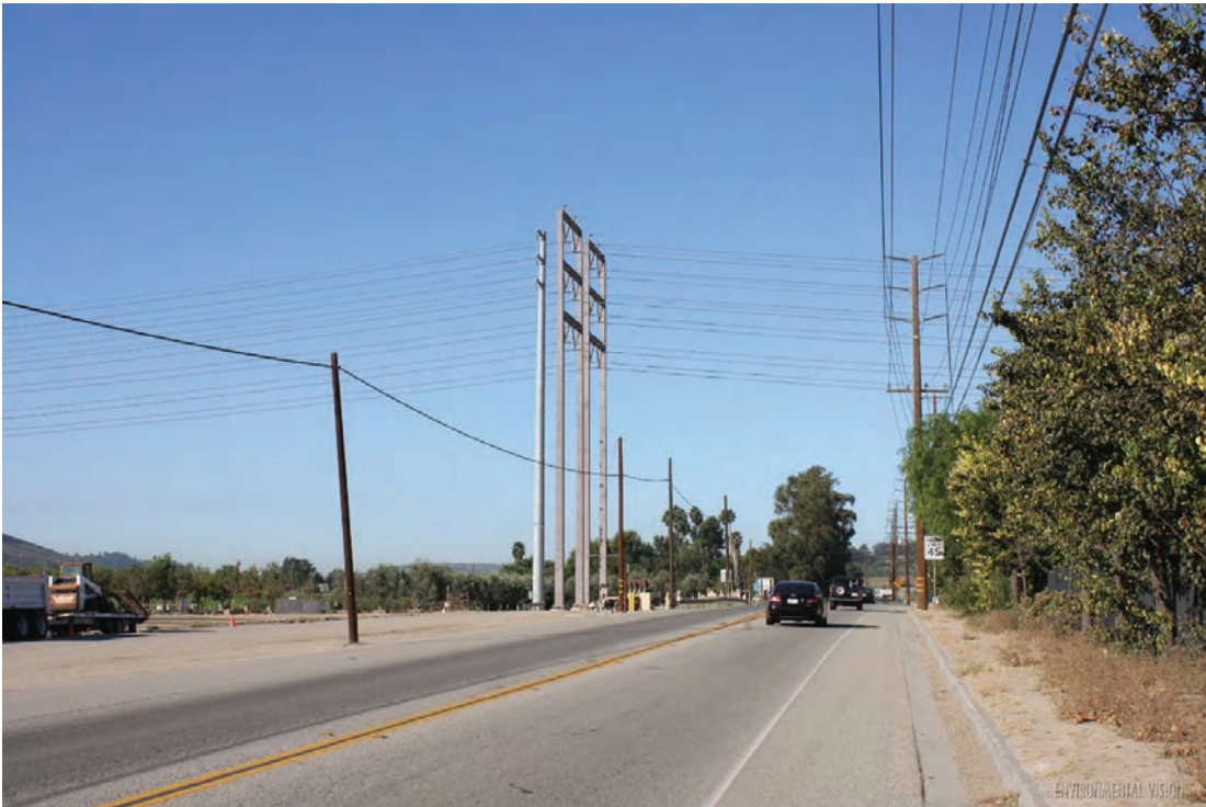
Simulated view from SR 118 looking west
