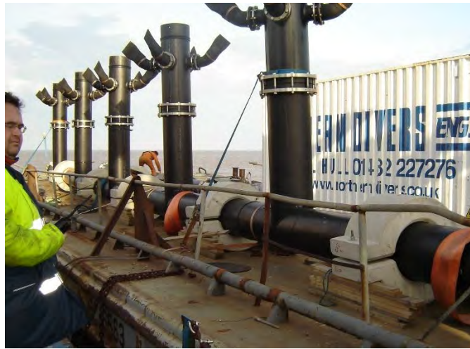
Figure 23. A brine diffuser with multiport rosettes.
