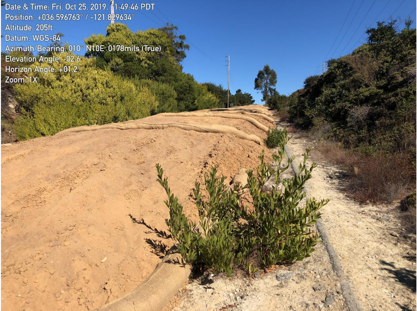
Figure 1: Soil deposition site on Mescal Street.
