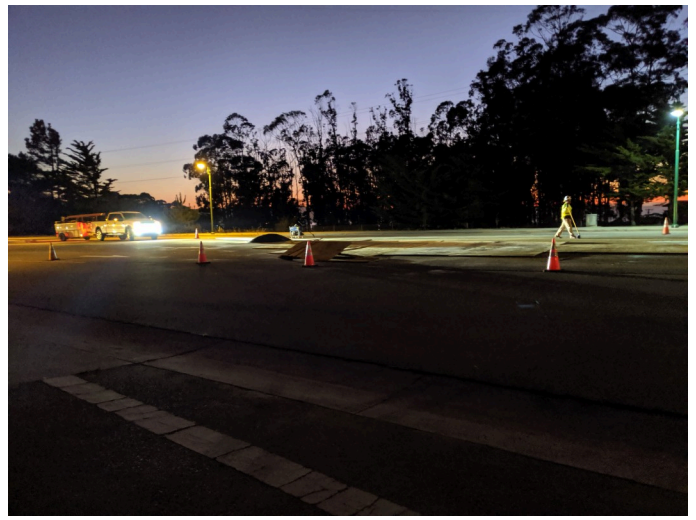
Facing SB GJM night work
