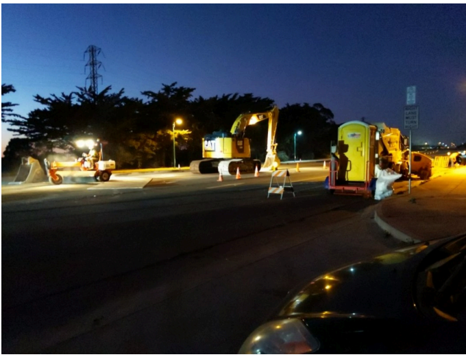
Facing NB GJM night work
