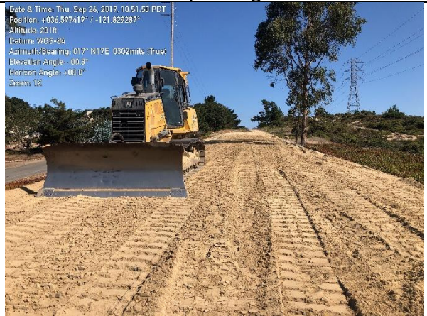
Photo 4. Offsite spoils site (between Mescal St. and General Jim Moore Blvd.)
