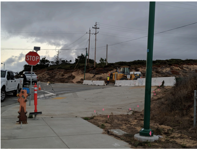
Staging Area behind the fence on Eucalyptus Rd
