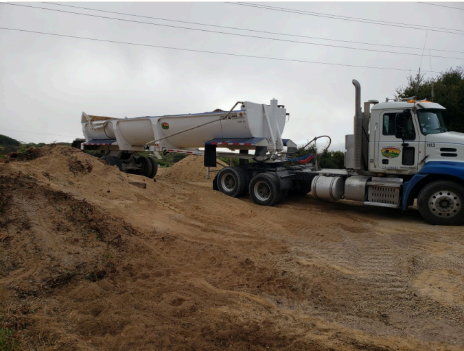
Unloading at spoils deposition site
