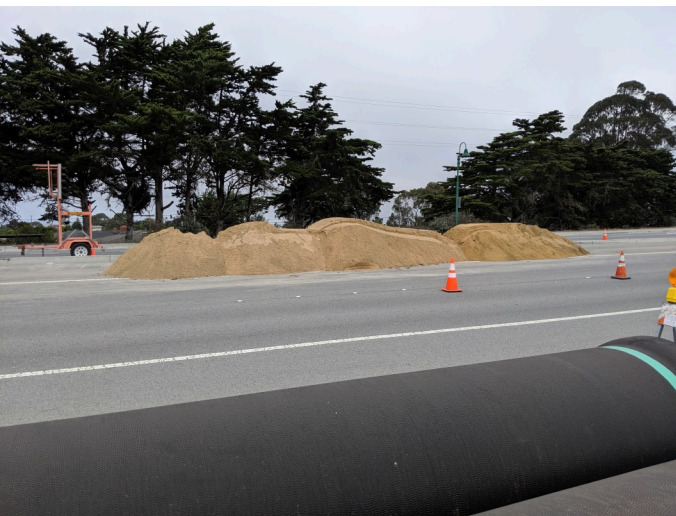
soil stockpile on alignment, facing west
