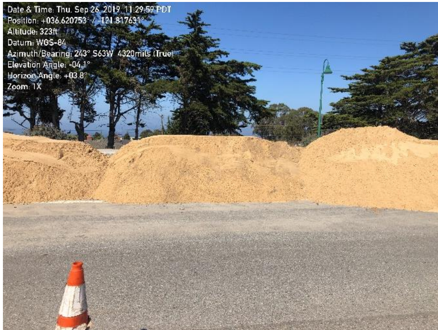
Photo 3. Temporary spoils pile
