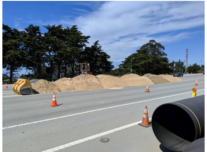
daily soil storage on site, facing NW
