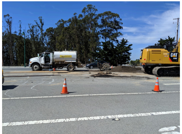
water truck on site for dust control, facing west
