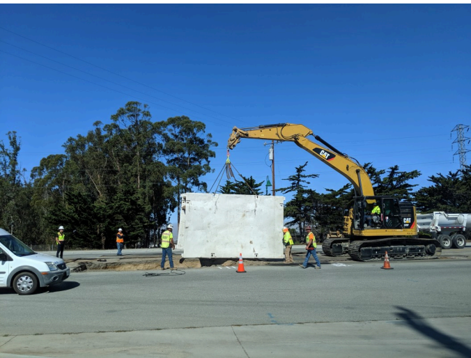
side view of vault, facing west
