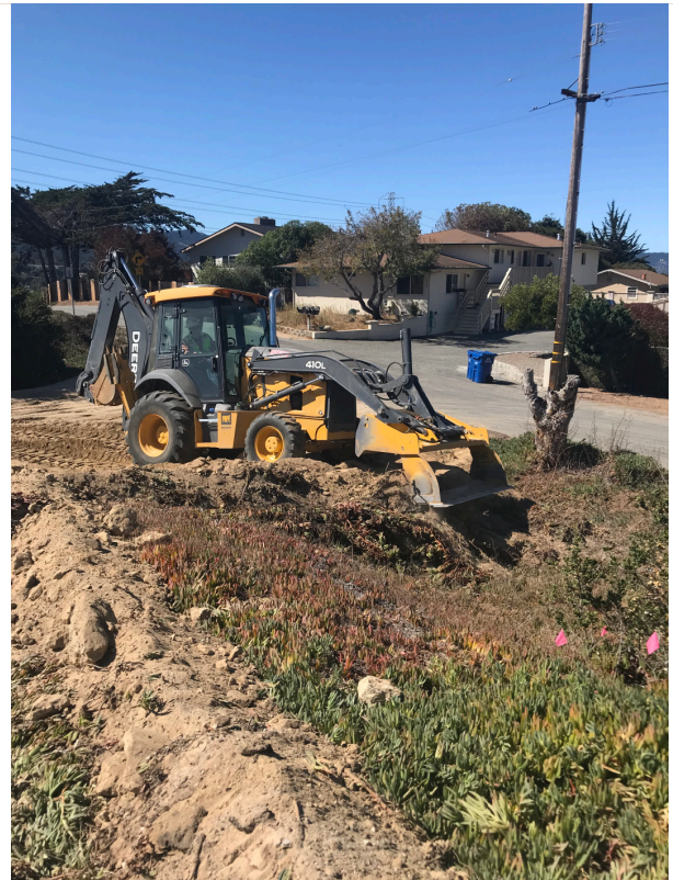
Garney operator cleaning up entrance to soil deposition area facing southwest
