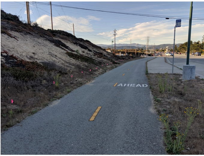
intact exclusionary flagging on site, facing south
