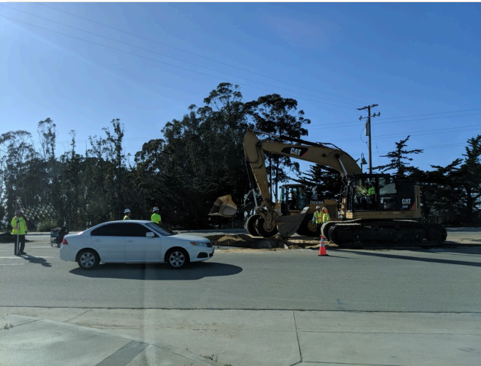
filling of trench, facing west
