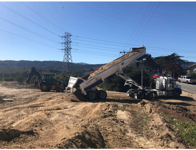
soil being deposited from pipeline construction facing south
