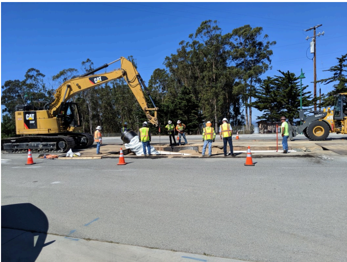
installing section of pipeline, facing west
