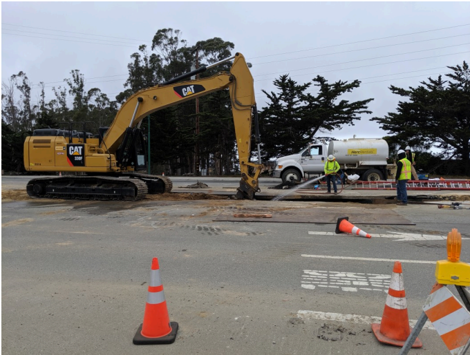
ground compaction and dust mitigation, facing west
