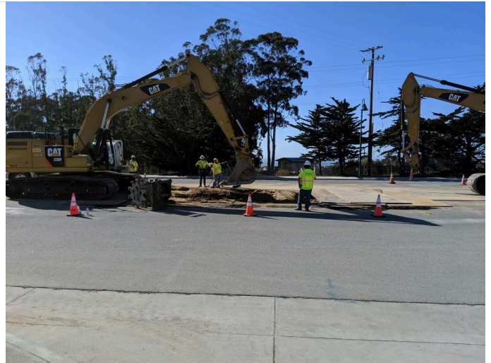
ground compaction following pipeline installation, facing west
