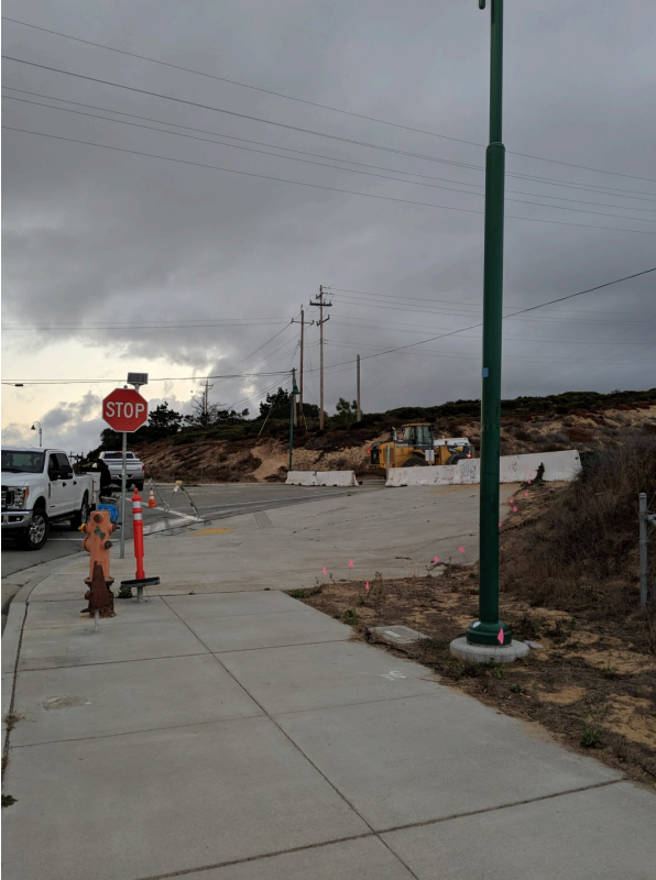
Staging Area behind the fence on Eucalyptus Rd
