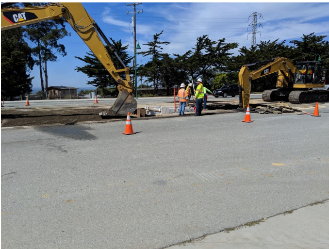
compaction of pipeline alignment, facing NW
