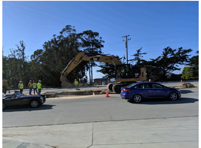
setting up trench vault, facing west
