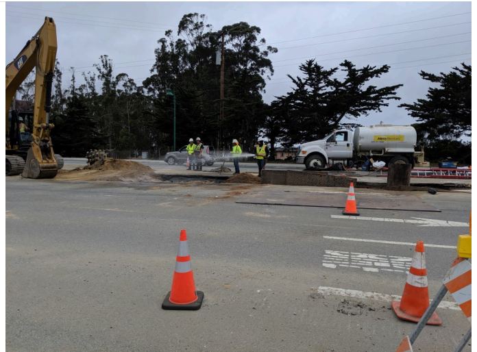
ongoing dust mitigation, facing SW
