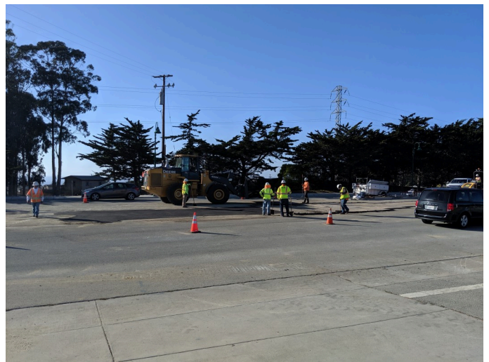
paving over trench line, facing West
