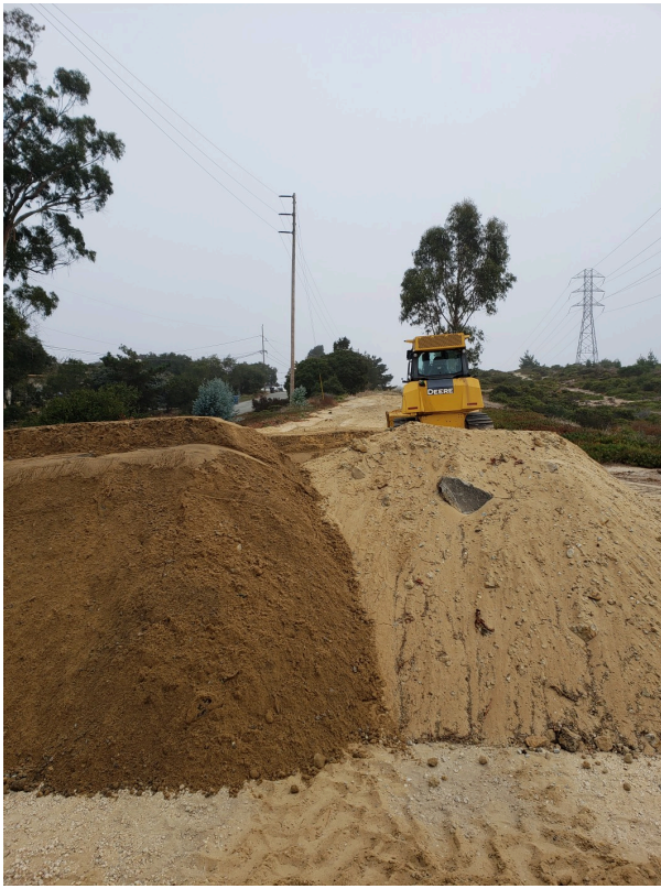
Spoils deposition site.
