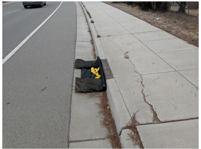
silt protection around storm drain, facing south
