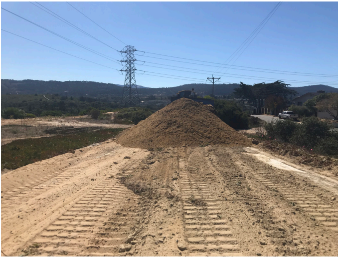
soil pile at soil deposition site facing south
