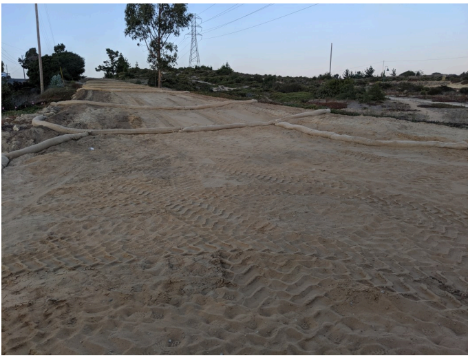
straw wattle installation, facing N
