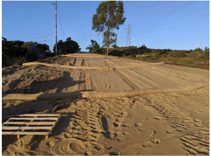
Straw Wattle installation, fscing N
