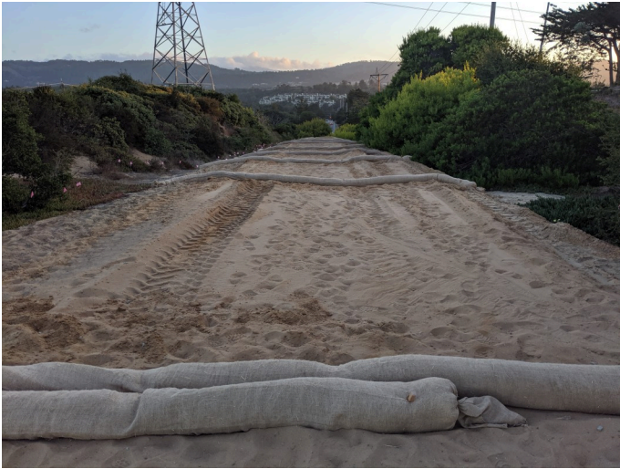
Straw wattle installation, facing S
