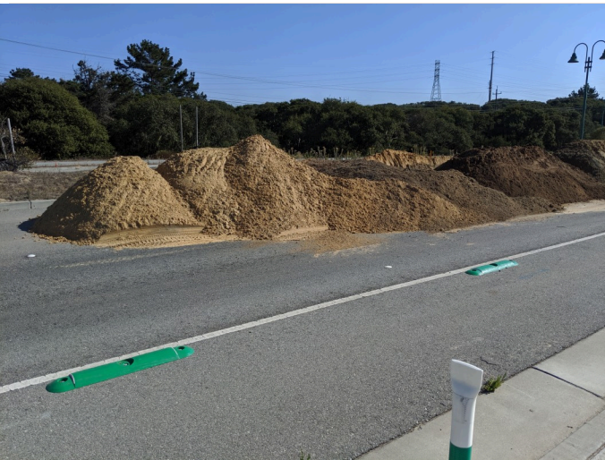
temporary soil storage on general Jim Moore, facing SW
