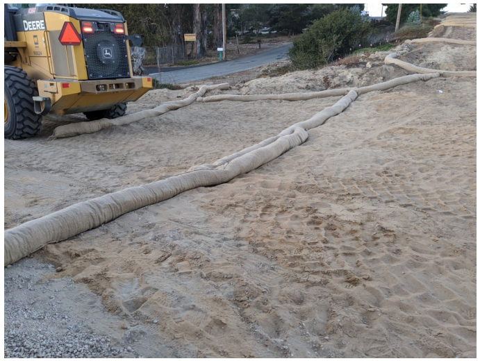
Straw wattle installation, facing W
