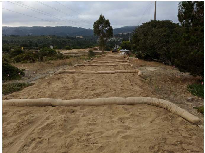
straw wattle erosion control, facing S
