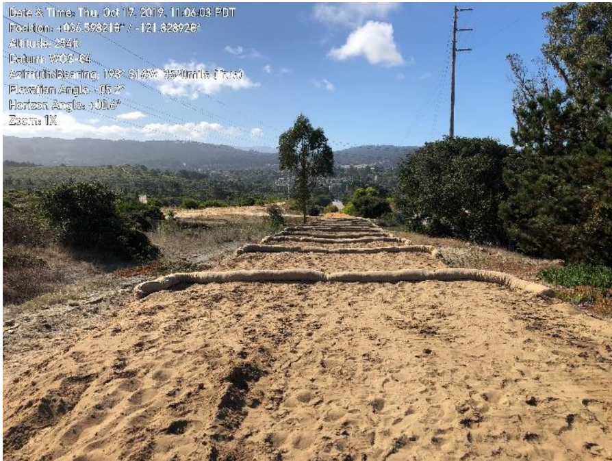
Photo 4. Erosion BMPs at offsite spoils site (Mescal Street)
