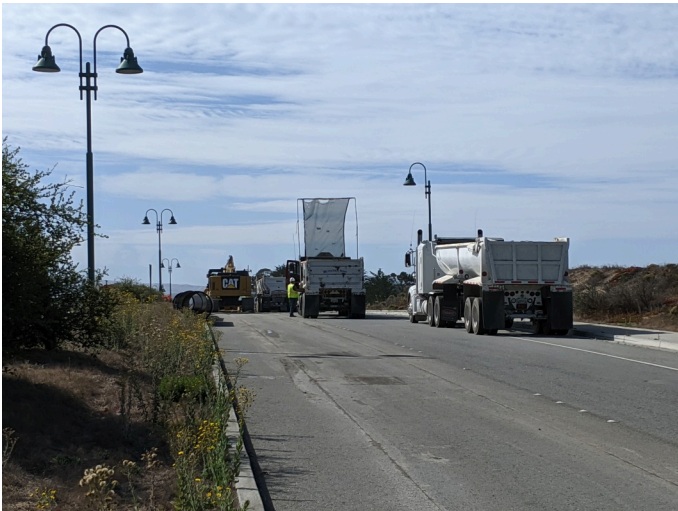
dust mitigation over soil transport truck, facing S
