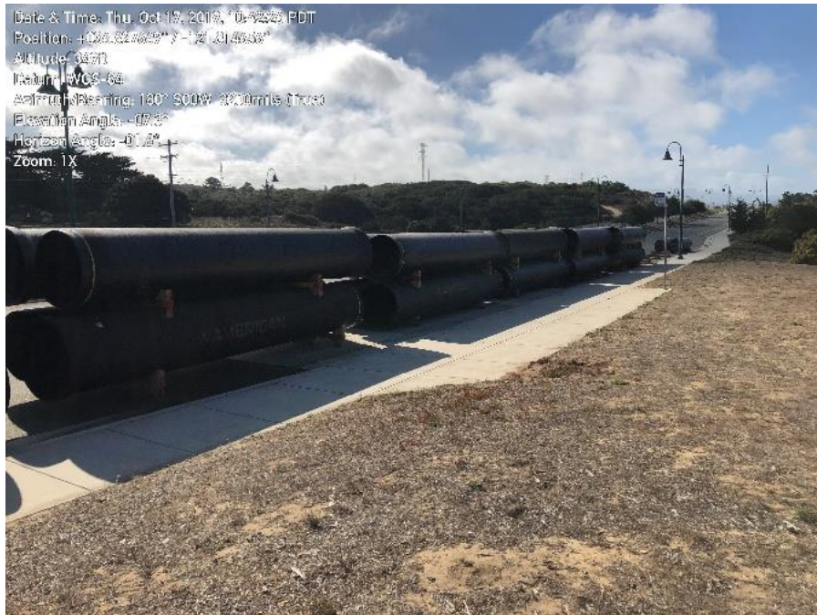
Photo 2. Materials staging on southbound side of General Jim Moore Blvd.
