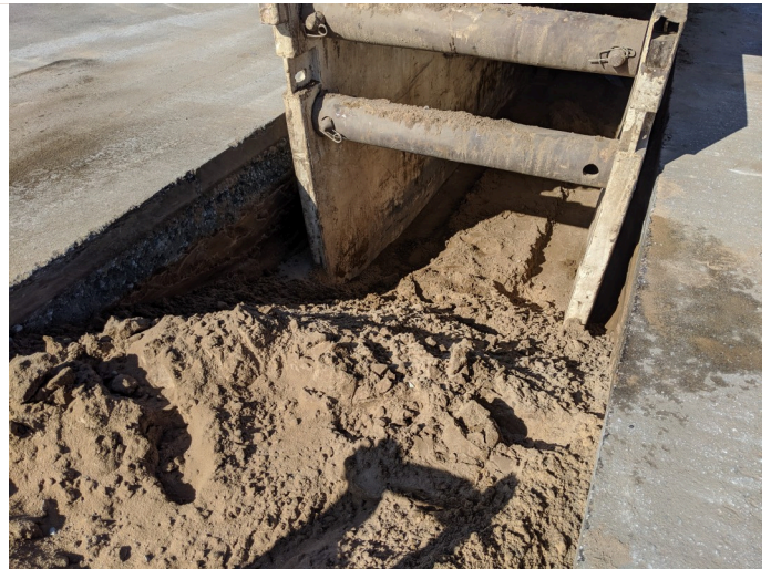
escape ramp out of pipeline trench, facing NW
