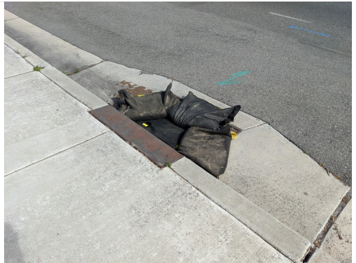
erosion control over storm drain along Gen Jim Moore
