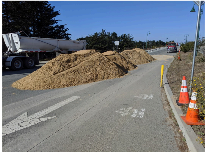
active soil stockpile on general Jim Moore, facing NW
