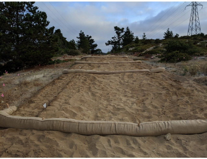
straw wattle erosion control at soil depot, facing N
