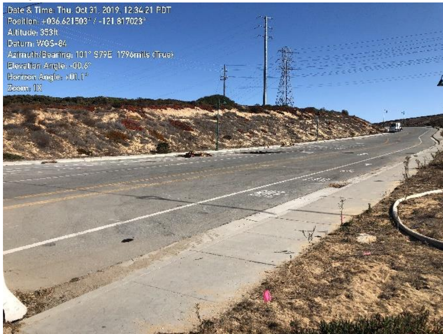
Photo 4. Cleanup of extra temporary staging area on Eucalyptus Road nearly complete.
