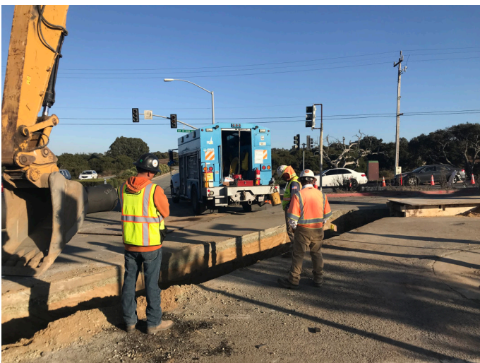
PGE fixing the broken gas line prior to installing plates
