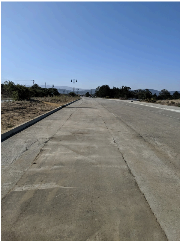
GJM cleaned and opened for traffic
