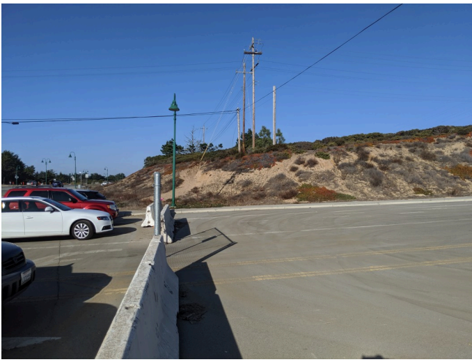
cleared staging area at Eucalyptus ave, facing W
