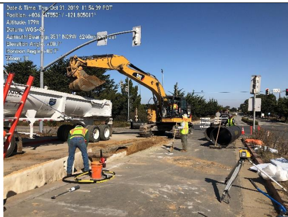
Photo 2. Trench excavation on Lightfighter Dr. and General Jim Moore Blvd. intersection.
