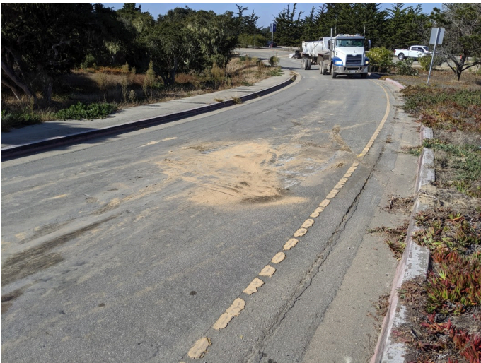
diesel leak area post-cleanup, facing NW
