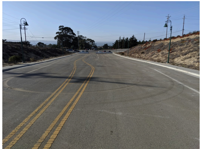
cleared staging area at Eucalyptus ave, facing S
