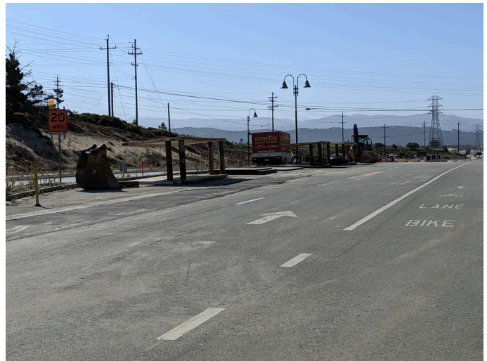
GJM cleaned and opened for traffic
