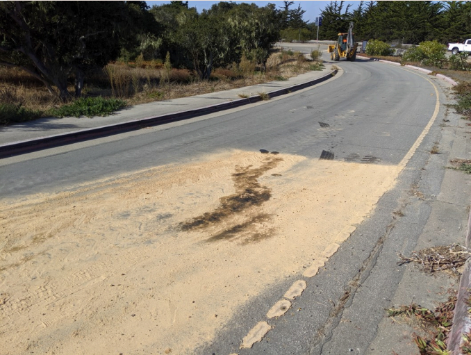
minor diesel fuel leak within roadway, sand applied and to be collected and stored, facing NW
