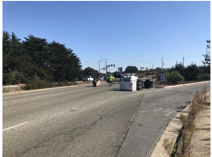
asphalt cutting along Lightfighter
