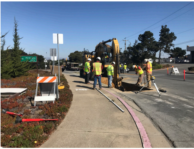
pipeline excavation along General Jim Moore
