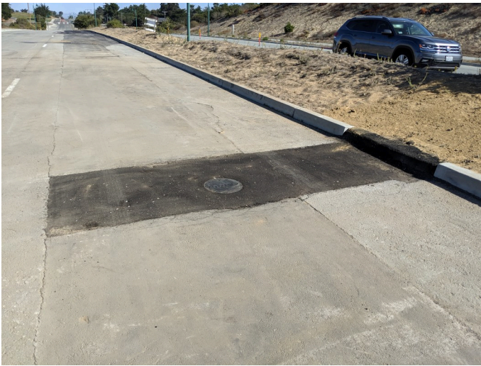
Patchwork for Air valve installation. Temporary curb was made with asphalt.
