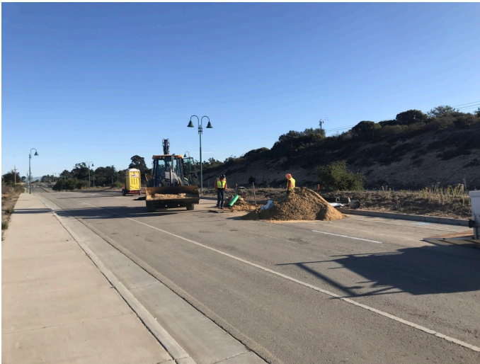
air valve installation along General Jim Moore
