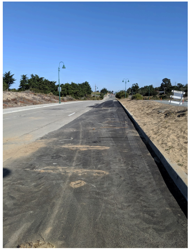
GJM cleaned and opened for traffic
