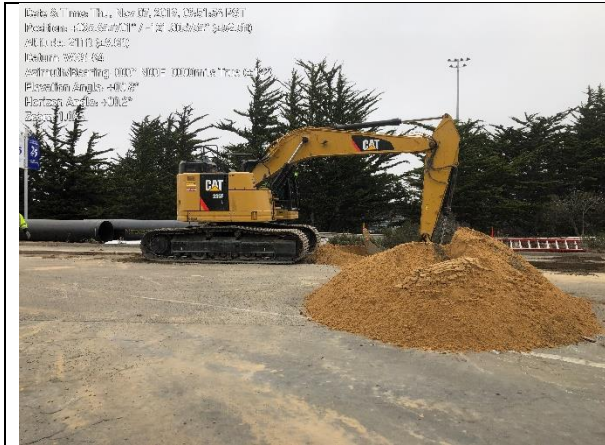
Photo 1. Trench excavation on Lightfighter Drive
