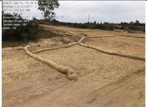
Photo 4. Straw wattle in place at Mescal spoils site
