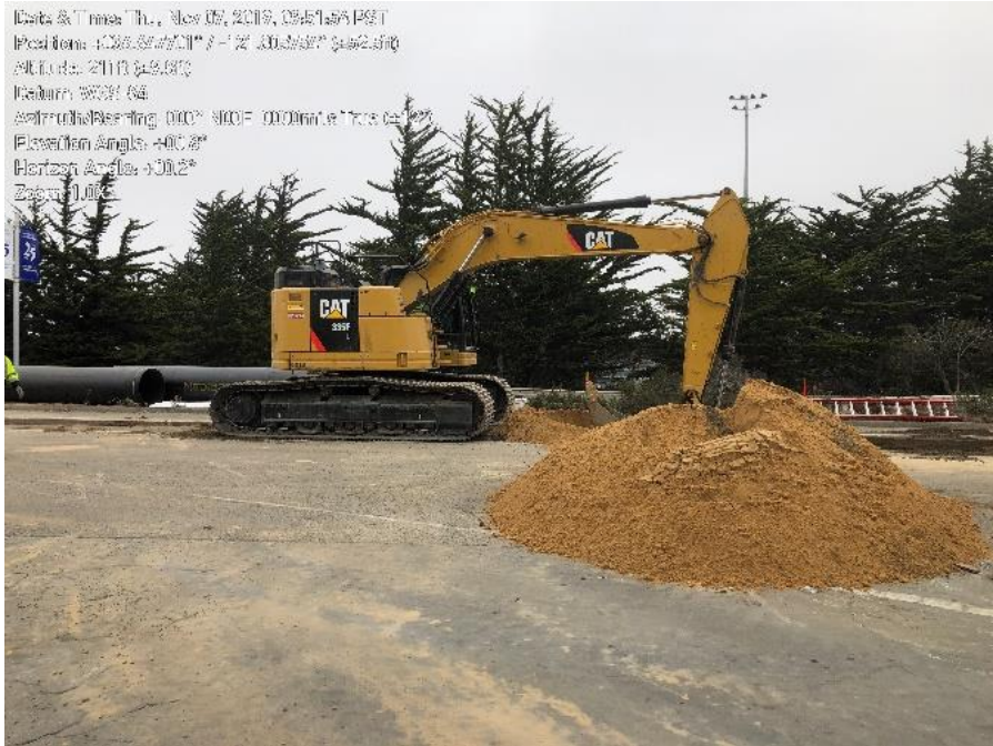
Photo 1. Trench excavation on Lightfighter Drive
