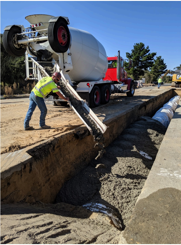
Start of slurry backfill at STA 7+69
