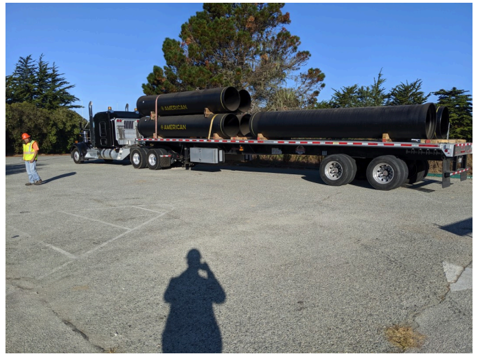
temporary staging of pipeline on transport trucks, facing N
