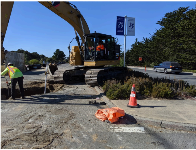
excavator parked on cleared vegetated median during excavation activities, facing W
