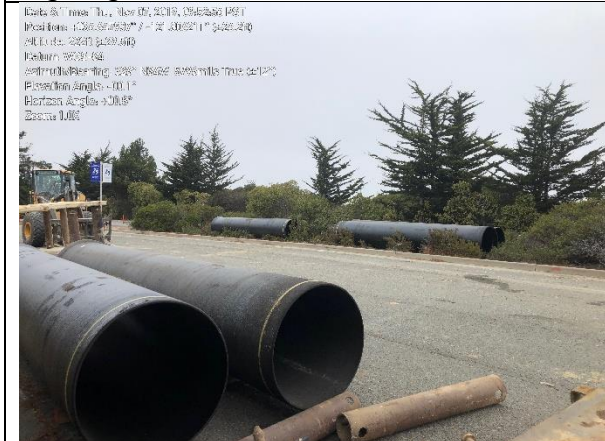
Photo 3. Pipes being staged in median on Lightfighter Drive
