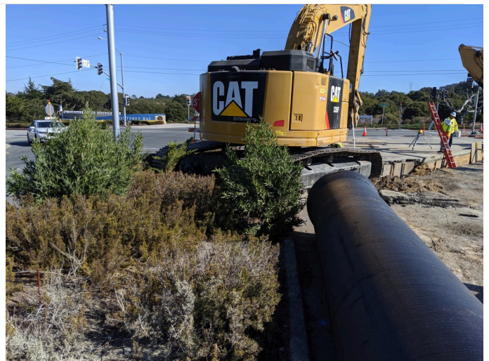
excavator parked on cleared vegetated median during excavation activities, facing N
