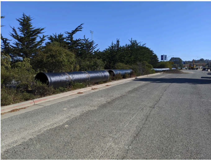
pipeline storage in surveyed and cleared median, facing E
