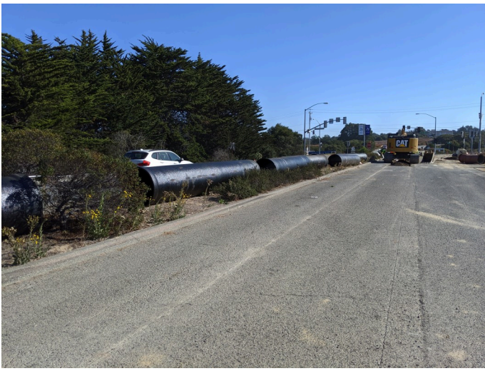
pipeline storage in surveyed and cleared median, facing E
