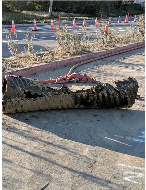
Old stormwater drain was placed
