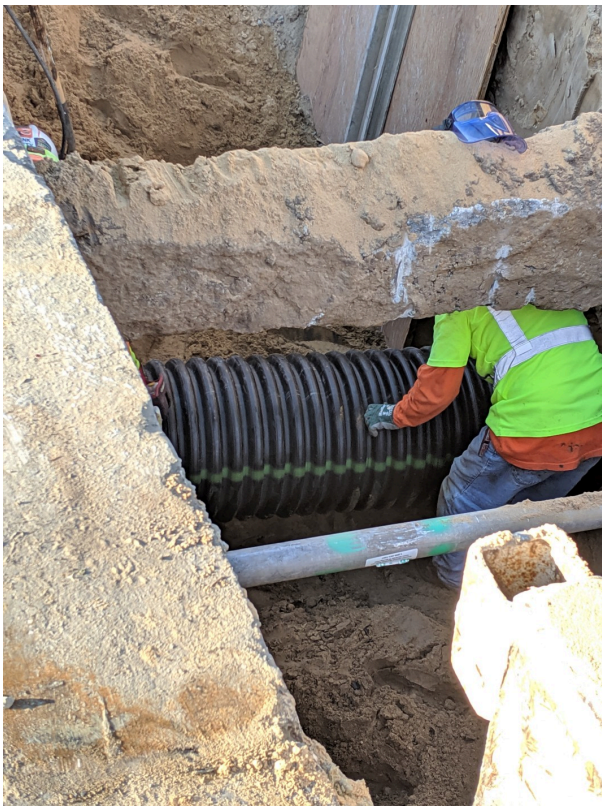
New stormwater drain
