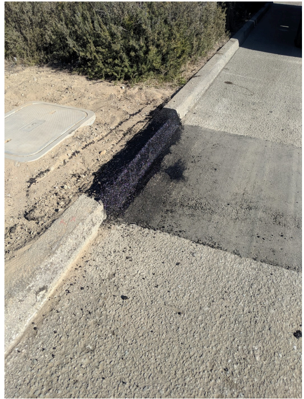
Dike was replaced in front of thr blow valve on Lightfighter
