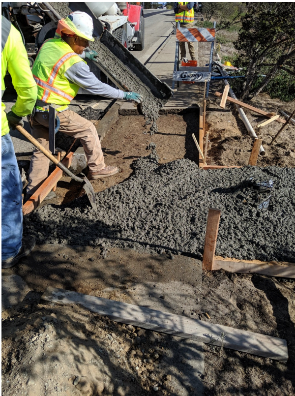
Concrete pouring for sidewalk and air valve by Lightfighter and 2nd.
