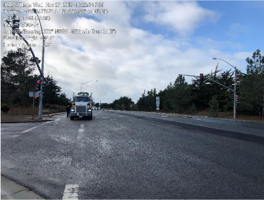
Photo 1. Demobilization of equipment on Lightfighter Drive
