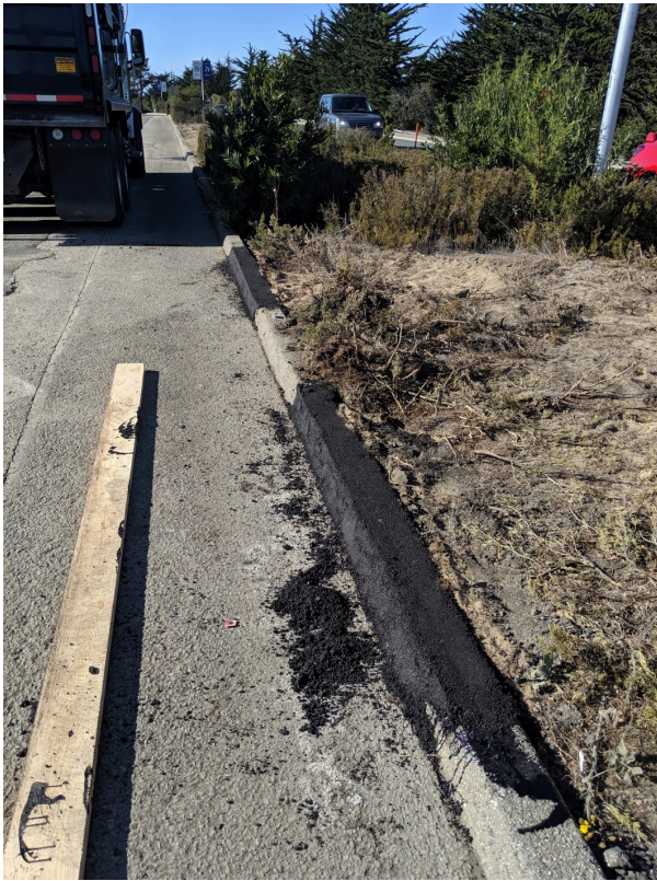
Dike was repaired at the intersection of Lightfighter and GJM
