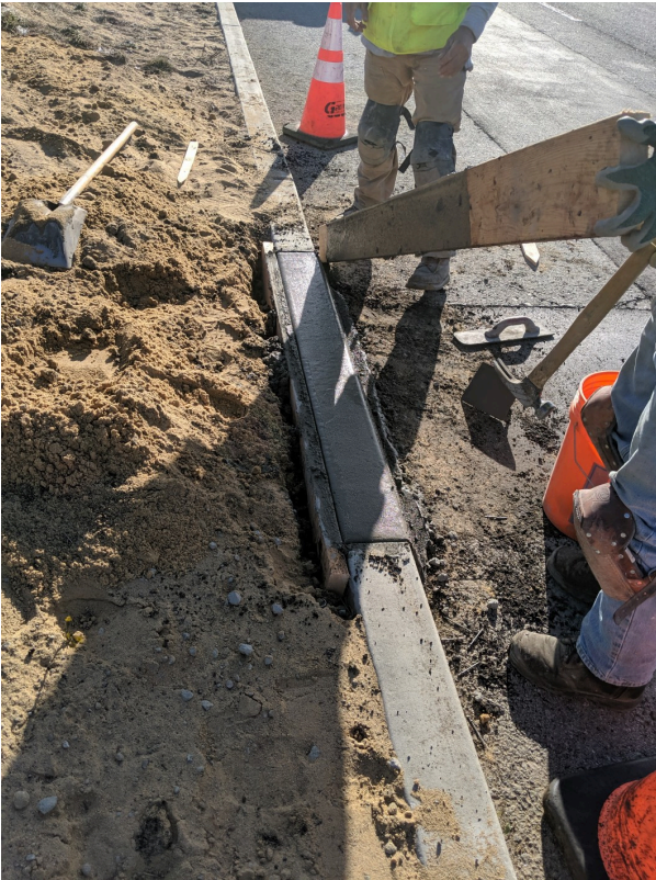
Curb replaced on GJM
