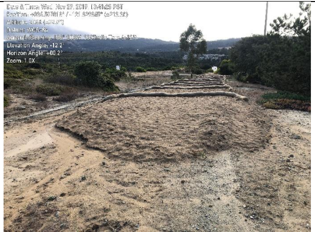
Photo 2. Offsite spoils deposition area off Mescal Street
