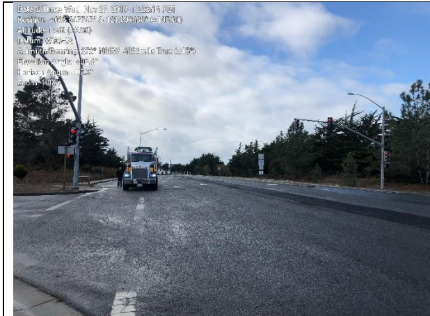
Photo 1. Demobilization of equipment on Lightfighter Drive
