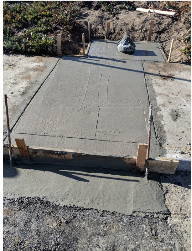
Concrete for air valve across the fire station on GJM.
