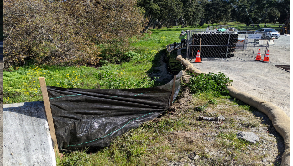
Photo 2. Installation of silt fencing around staging area. (2-19-2020).
