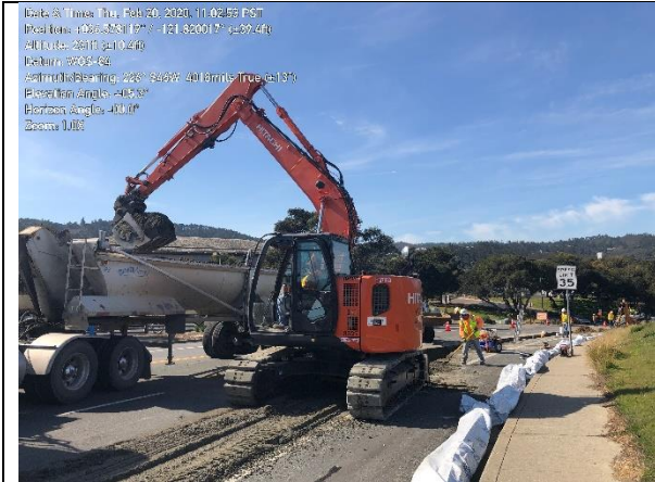
Photo 1. MPE excavation of pipeline trench
