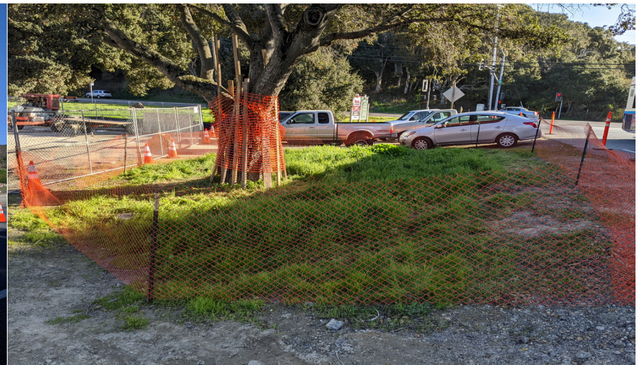
Photo 4. Completed ESA fencing protection around tree outside of staging area. (2-19-2020).
