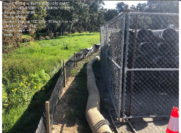
Photo 2. Silt fence surrounding staging area
