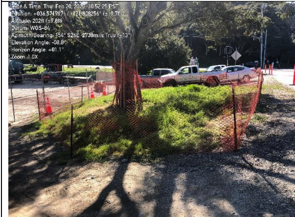
Photo 3. Tree protection installed around drip line of oak tree
