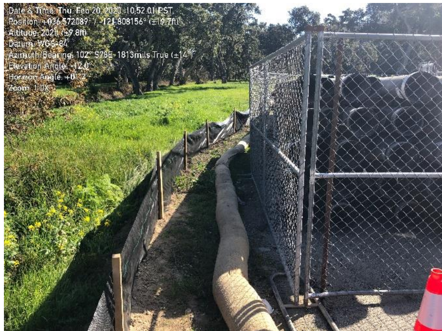
Photo 2. Silt fence installed around staging area off of York Road
