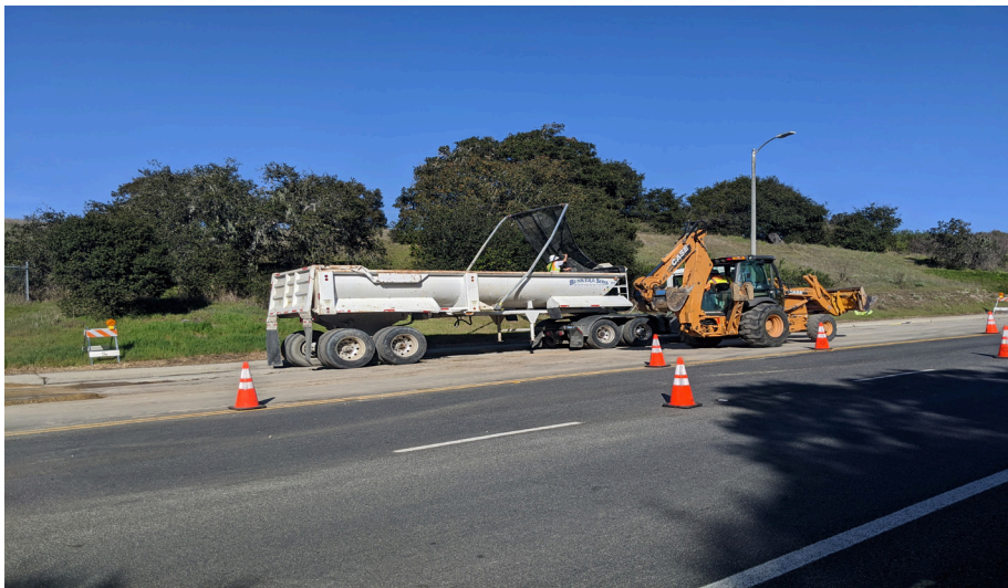
Photo 3. Dust control coverage over soil transportation vehicles. (2-19-2020).
