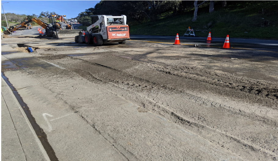
Photo 1. Dust abatement within minimal water usage. (2-18-2020).
