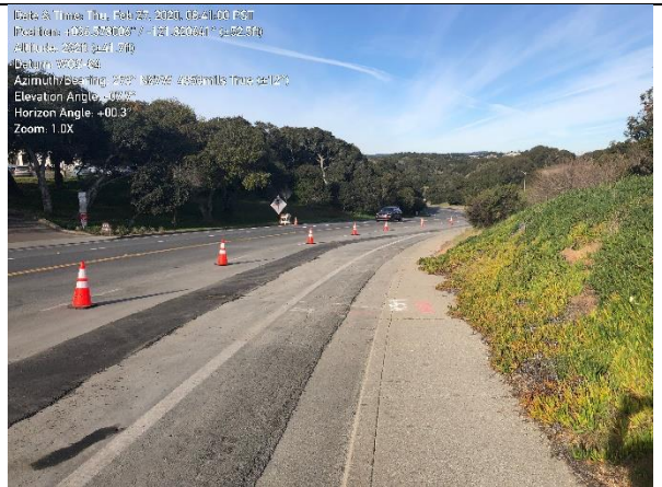
Photo 2. Completed pipeline installation on Ragsdale Drive
