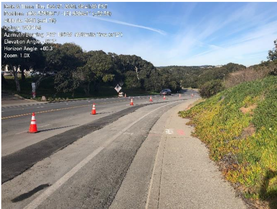
Photo 2. Completed pipeline installation on Ragsdale Drive
