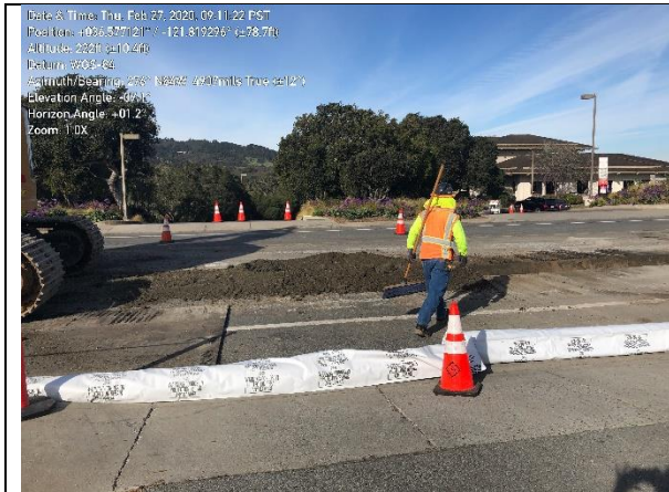
Photo 1. MPE excavation of pipeline trench
