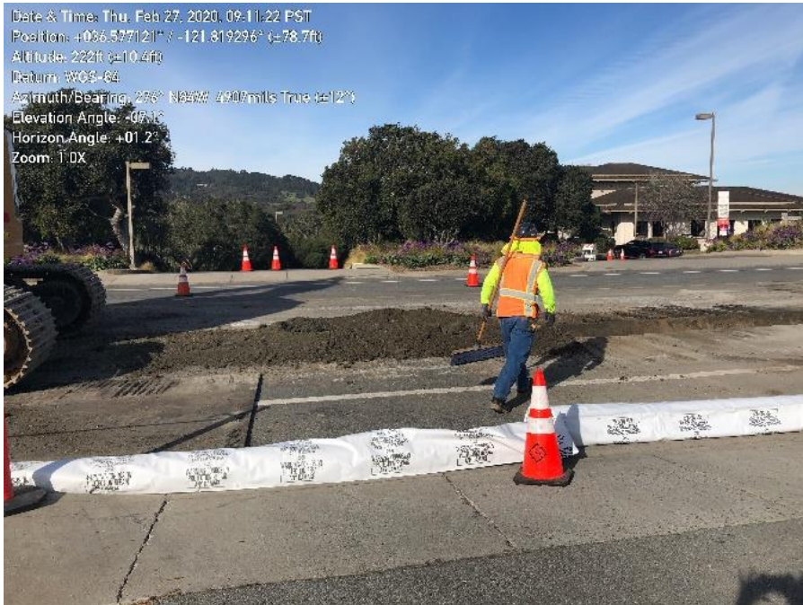
Photo 1. MPE excavation of pipeline trench on Ragsdale Drive.
