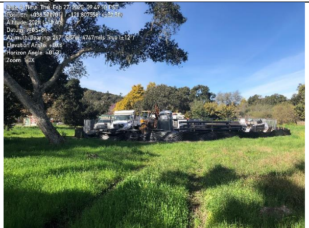
Photo 4. Silt fence around staging area
