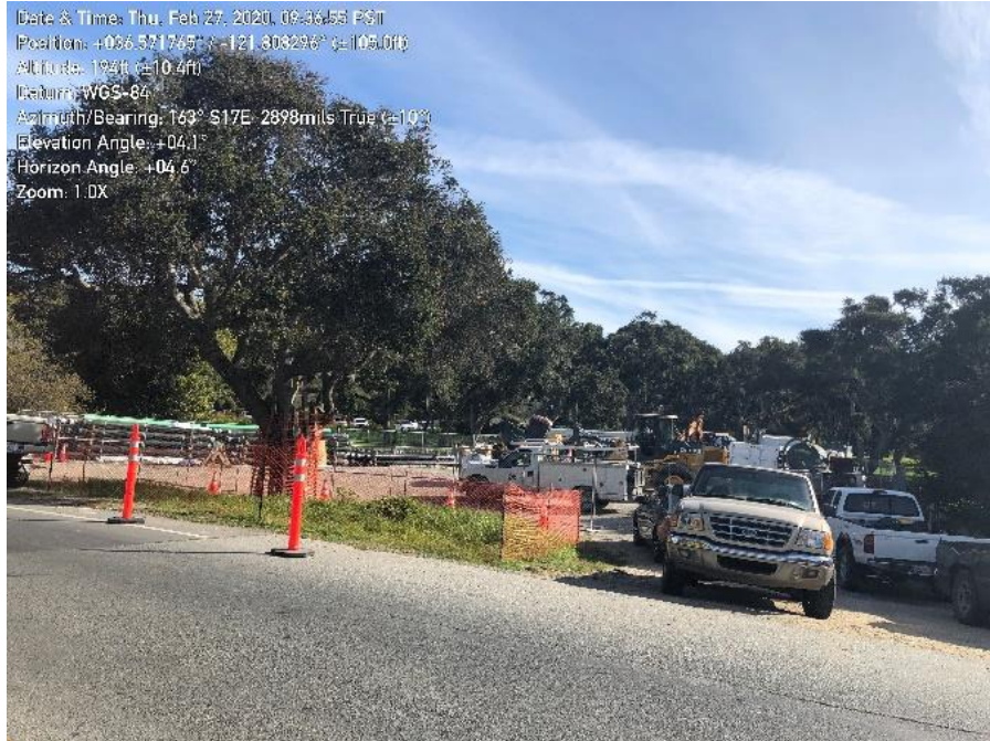
Photo 3. Tree protection around coast live oak tree in front of York Road staging area
