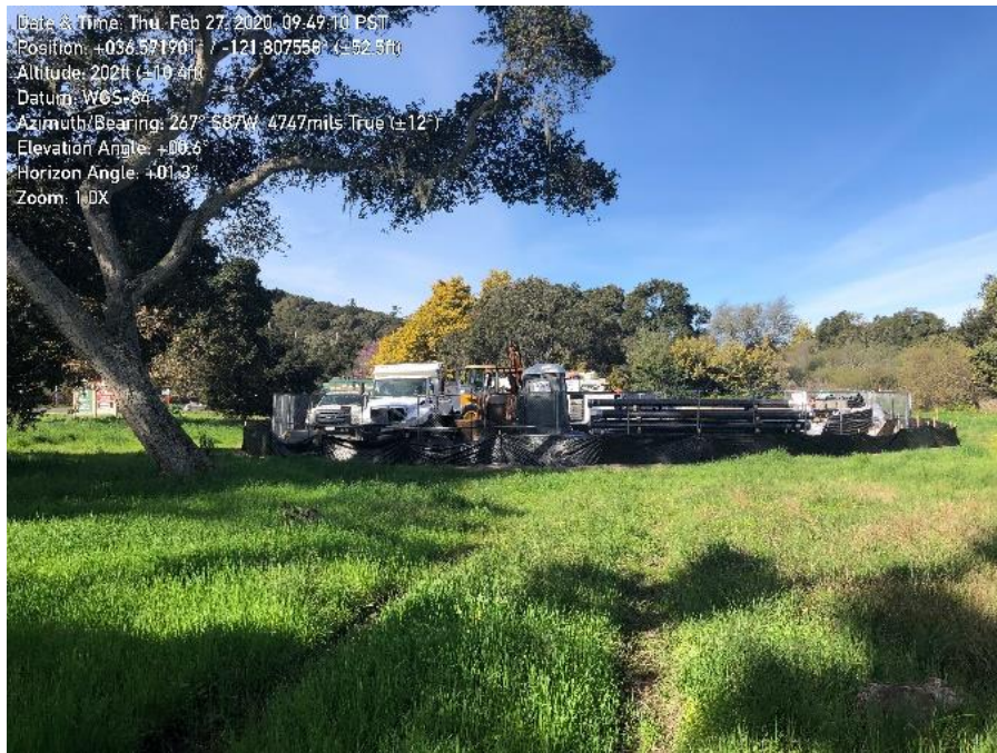
Photo 4. Silt fence installed around staging area off of York Road
