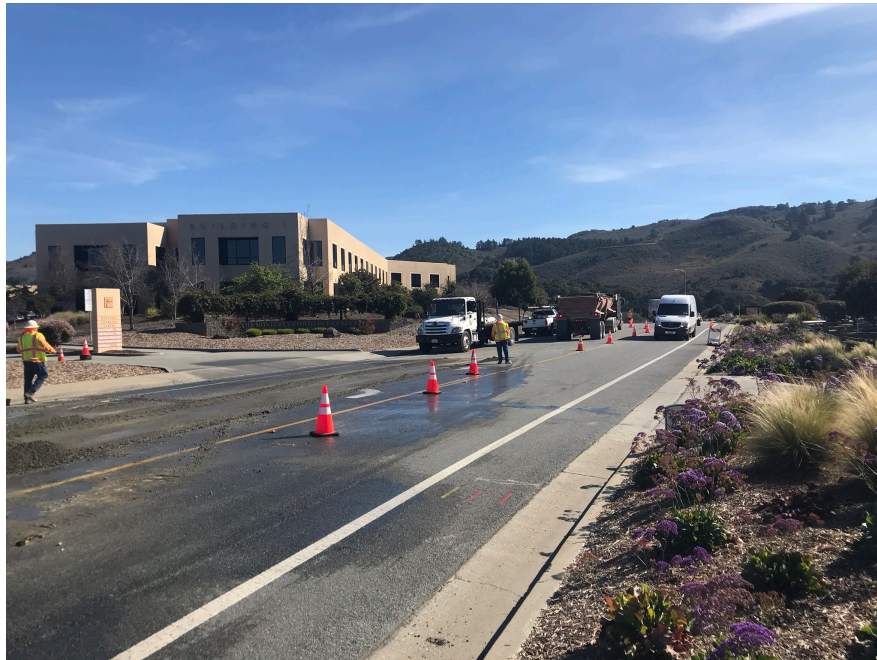
Photo 4. Minimal usage of water for dust mitigation along alignment. (02-26-2020)
