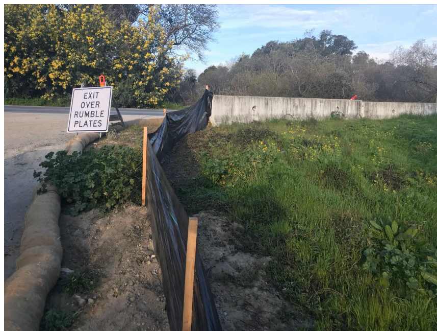
Photo 2. Protective silt fencing surrounding staging area. (02-21-2020)
