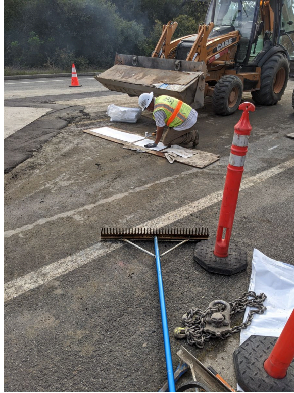
Photo 5. Preparation of hazardous spill protective mats for onsite vehicles and equipment stored overnight. (03-10-2020)
