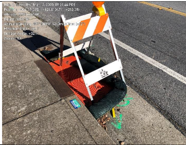
Photo 2. Storm drains protected
