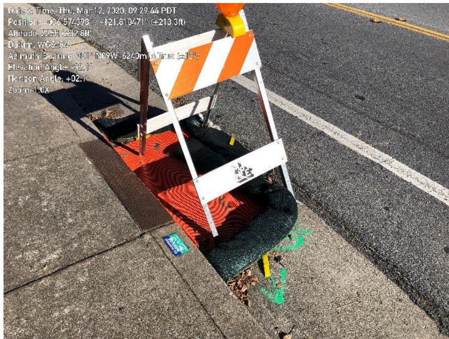
Photo 2. Protected storm drain on Lower Ragsdale Drive
