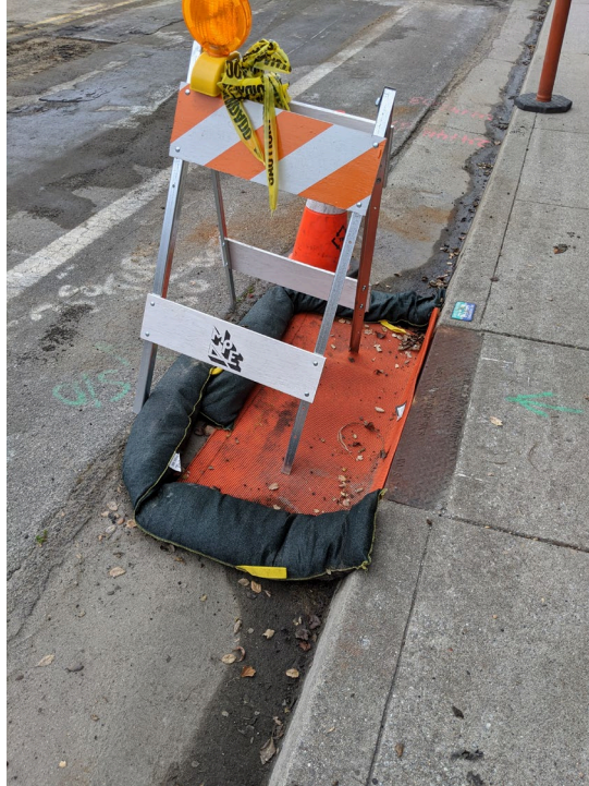
Photo 3. Stormwater drain protection post-maintenance. (3-9-2020)
