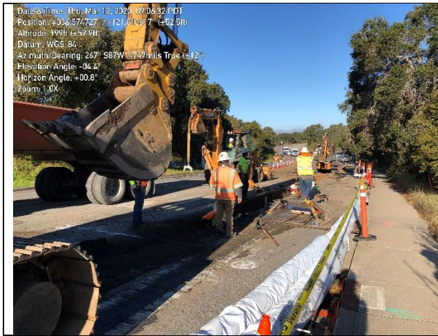
Photo 1. MPE excavation of pipeline trench on Lower Ragsdale Drive
