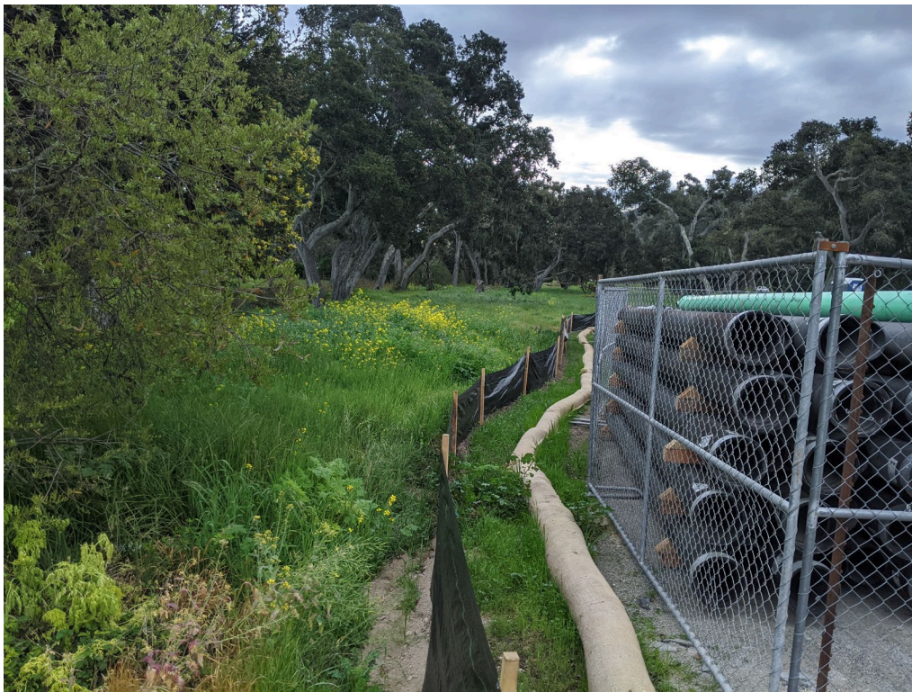
Photo 4. Intact silt fencing around staging area. (3-9-2020)
