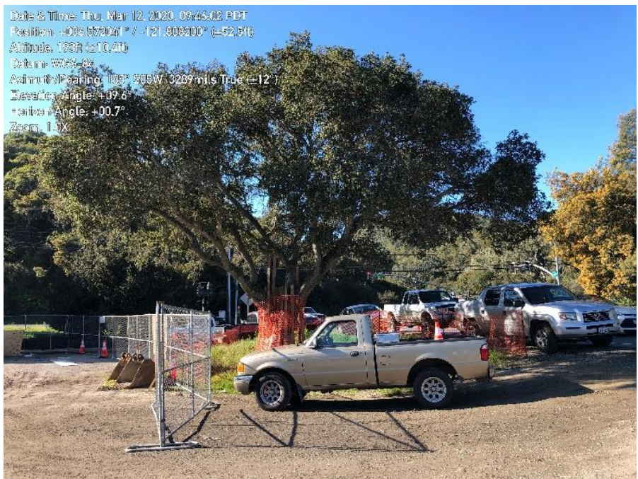
Photo 4. Tree protection and silt fence at staging area off of York Road
