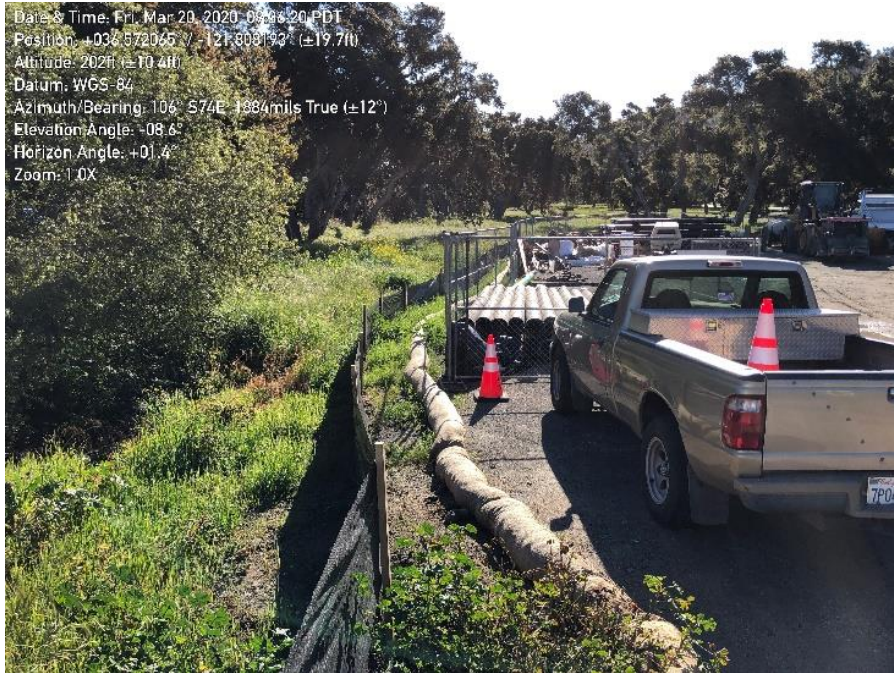
Photo 3. Silt fence surrounding staging area
