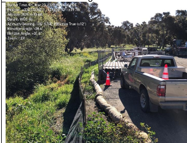
Photo 3. Silt fence surrounding staging area
