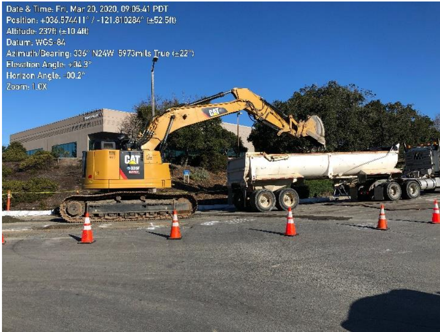
Photo 1. MPE excavation of pipeline trench on Lower Ragsdale Drive.
