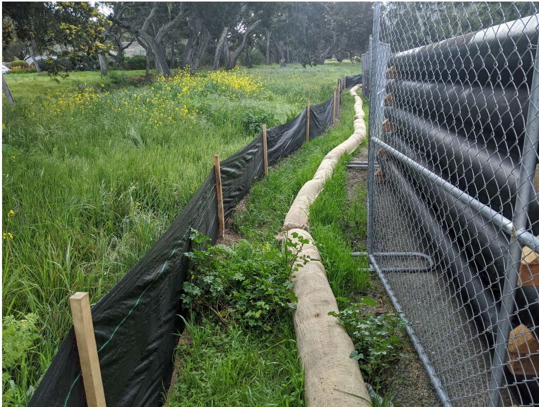
Photo 2. Intact silt fencing surrounding staging area. (3-13-2020)
