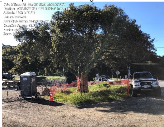
Photo 4. Tree protection at staging area
