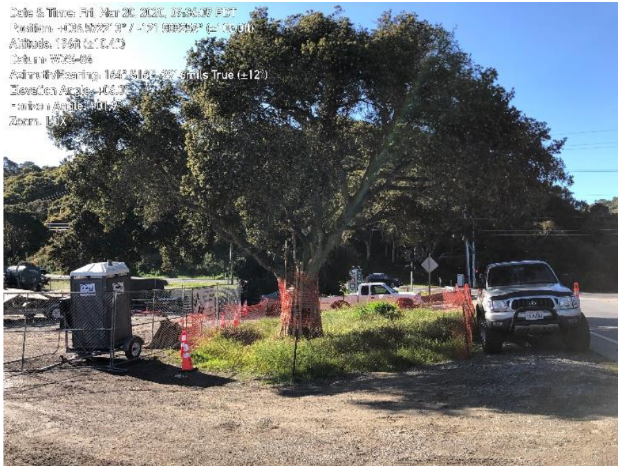
Photo 4. Tree protection at staging area
