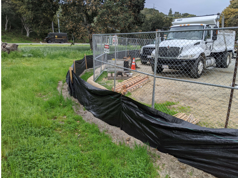
Photo 3. Secondary view of intact silt fencing surrounding staging area. (3-13-2020)
