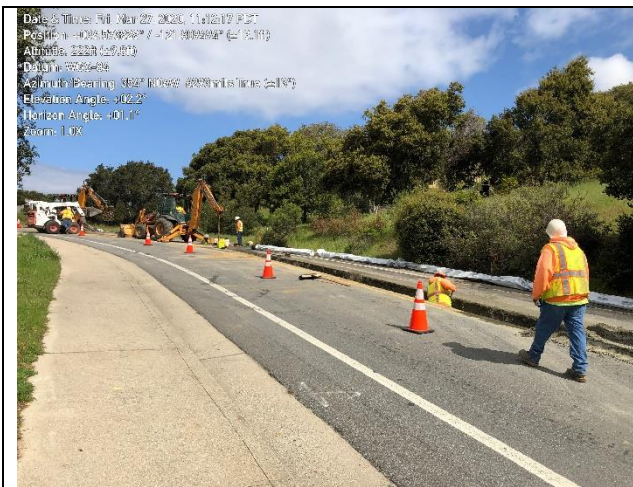
Photo 1. MPE excavation of pipeline trench on Wilson Road.
