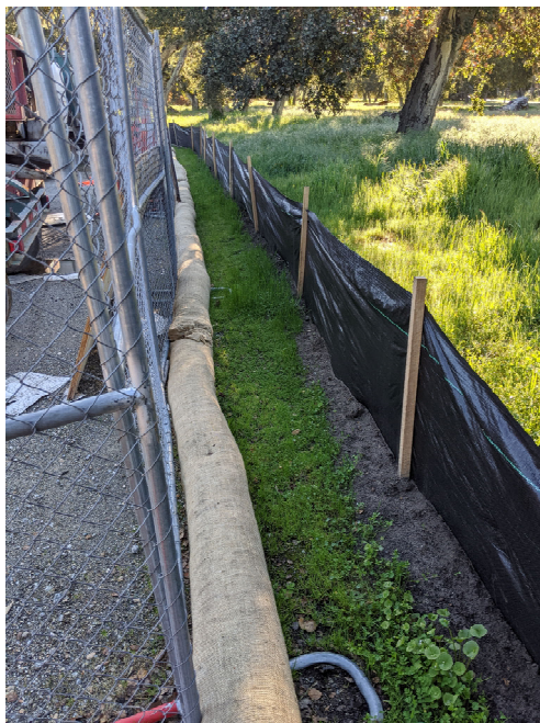
Photo 1. Intact silt fencing surrounding staging area. (3-20-2020)
