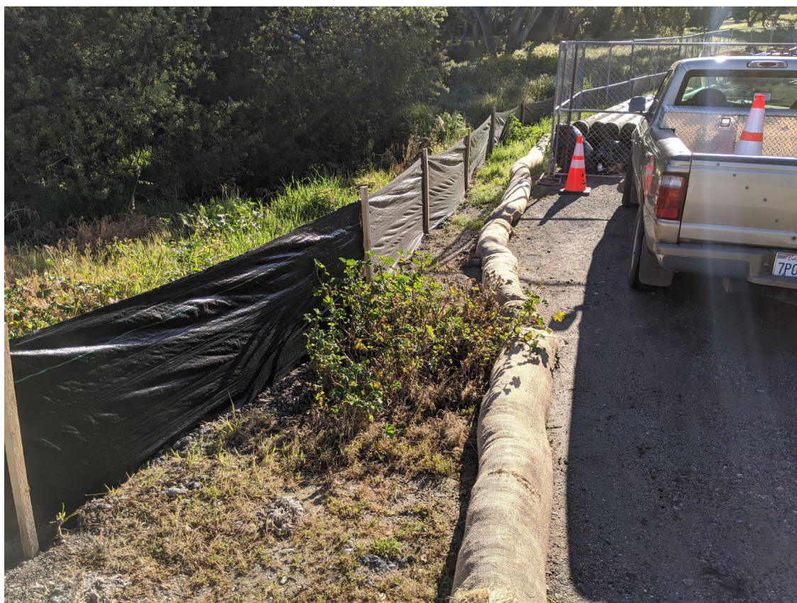
Photo 2. Secondary view of intact silt fencing surrounding staging area. (3-20-2020)
