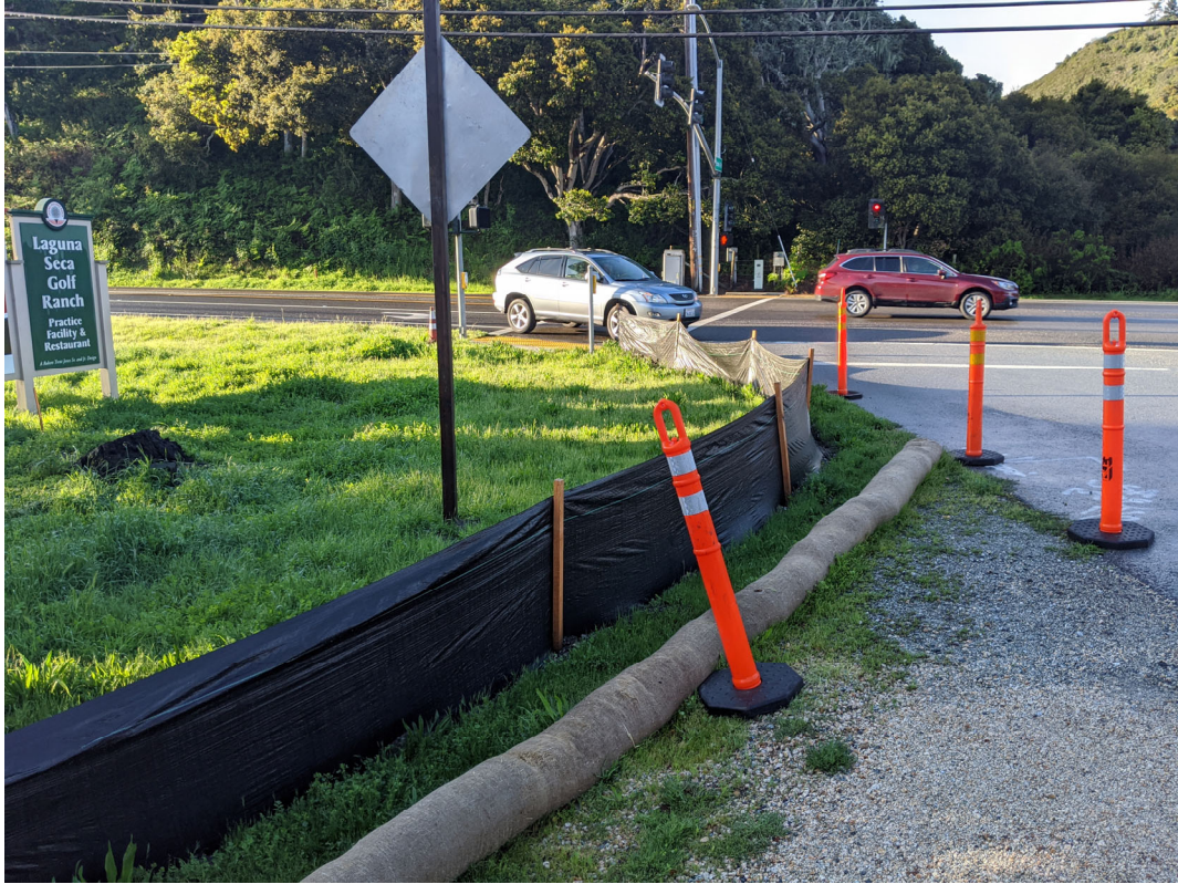
Photo 5. Intact silt fencing around staging area. (3-26-2020)
