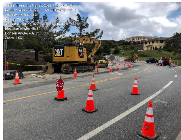
Photo 2. Temporary equipment staging on Lower Ragsdale Drive.
