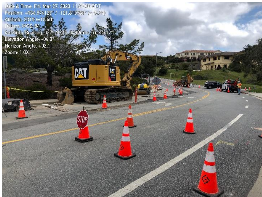
Photo 2. Temporary equipment staging on Lower Ragsdale Drive.
