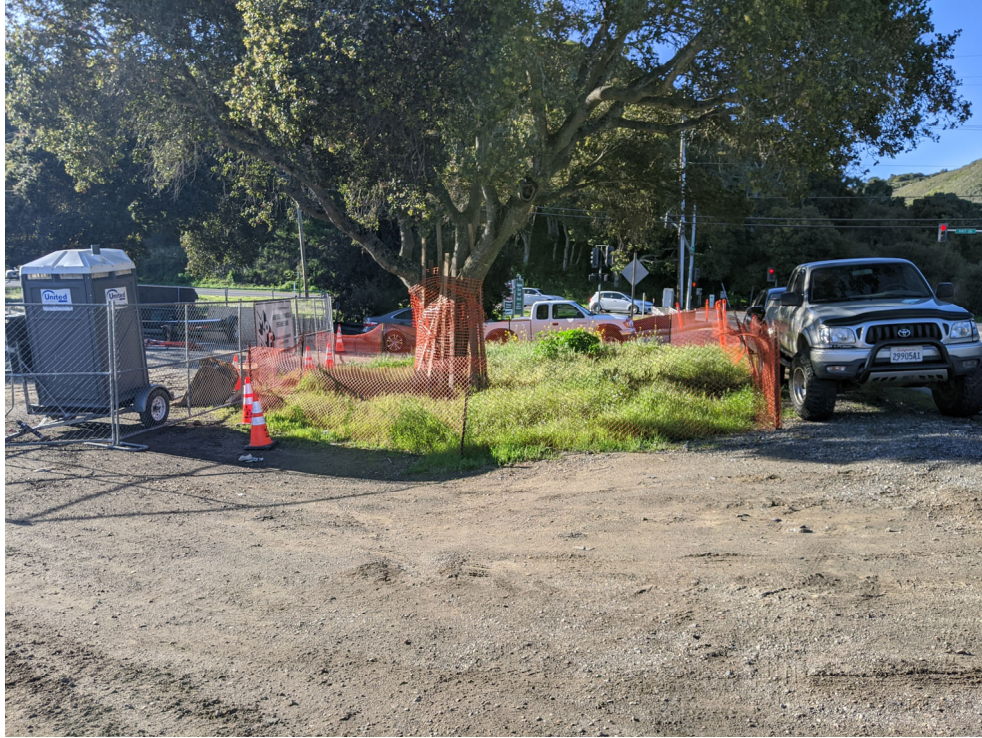
Photo 3. Intact ESA fencing around protected coast live oak tree adjacent to staging area. (3-20-2020)
