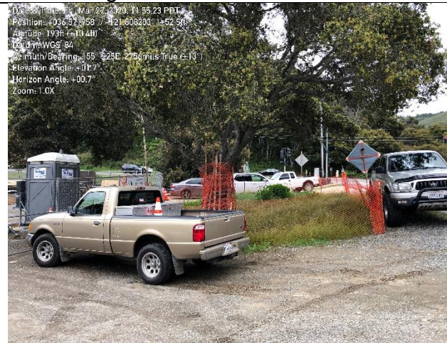
Photo 4. Tree protection and silt fence around staging area in good condition
