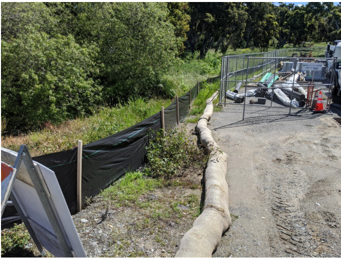
intact silt fencing surrounding staging area
