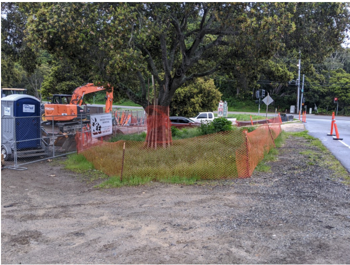
Intact ESA fencing around protected oak tree adjacent to staging area
