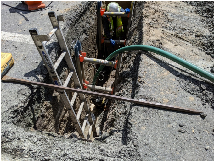
pumping of infiltrated groundwater out of alignment for blow-off valve installation
