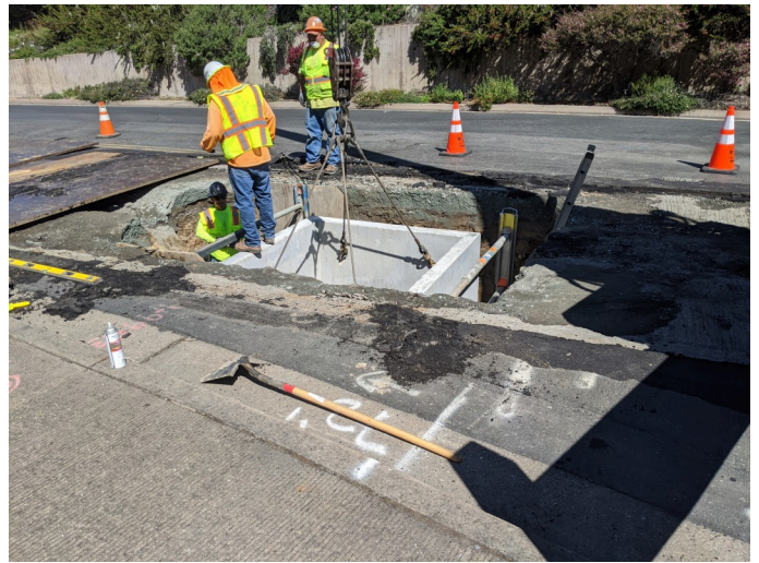
installation of vault along blue larkspur lane (end of alignment)
