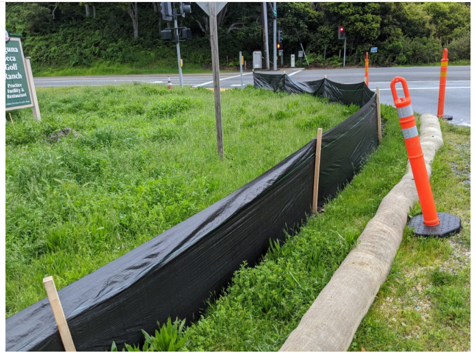
Intact silt fencing surrounding staging area
