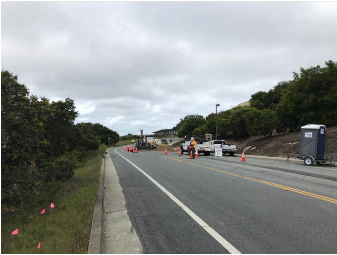
installation of blowoff along Lower Ragsdale Rd
