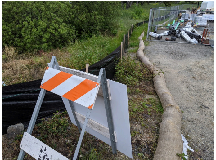
Intact silt fencing surrounding staging area
