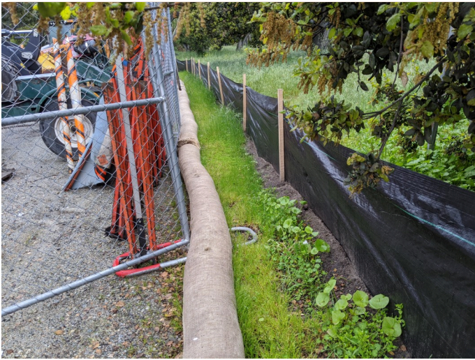
Intact silt fencing surrounding staging area
