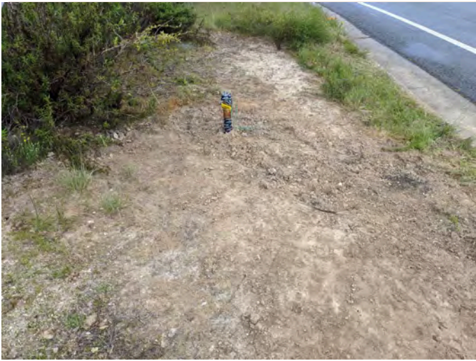
finished ARV on Lower Ragsdale
