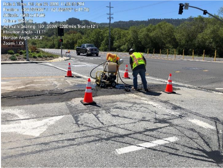
Photo 1. MPE pressure testing on Ragsdale Drive at Highway 68.
