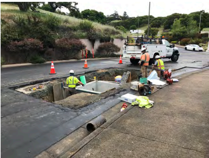
installation of PRV on Blue Larkspur Ln
