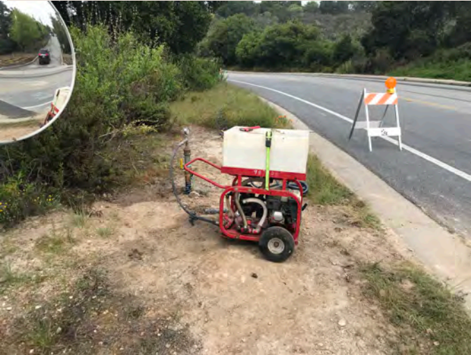
MPE conducting pressure testing of pipeline
