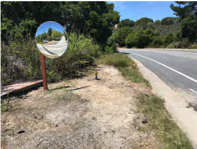
Air Release Valve (ARV) post construction activities.
