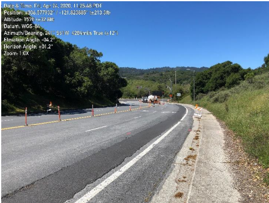
Photo 2. Conditions on Ragsdale Drive.
