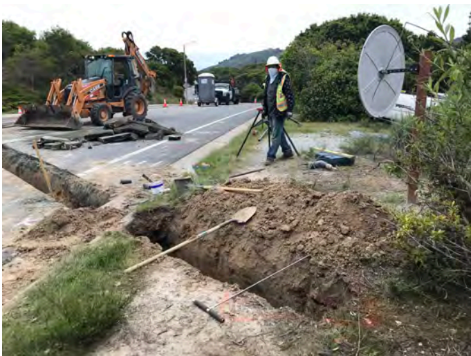
Air valve installation along Lower Ragsdale Rd
