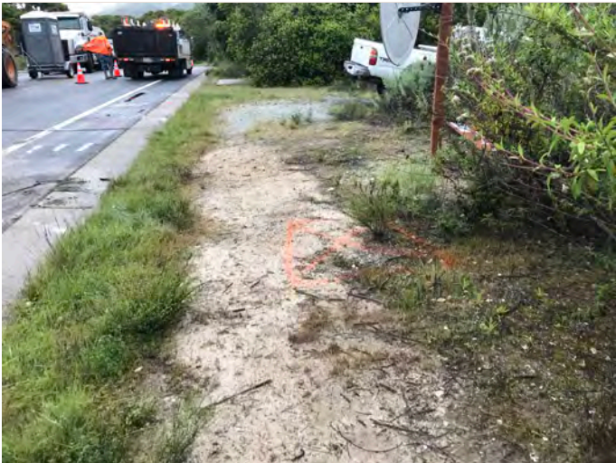
air valve location prior to installation
