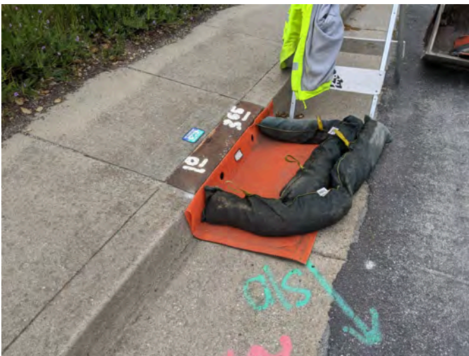
View of BMP usage adjacent to construction on Ragsdale Drive.
