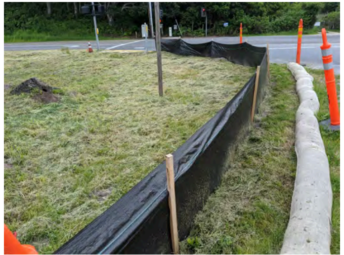
additional view of intact silt fencing surrounding staging area
