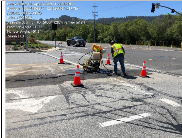
Photo 1. MPE pressure testing on Ragsdale Drive at Highway 68.
