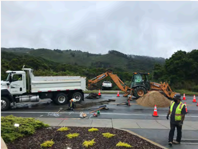
air valve installation on Lower Ragsdale Rd
