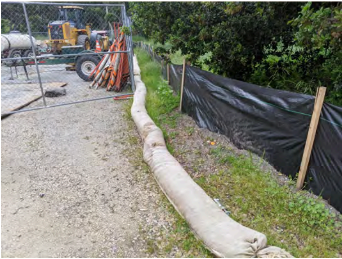
View of intact silt fencing surrounding the staging yard.
