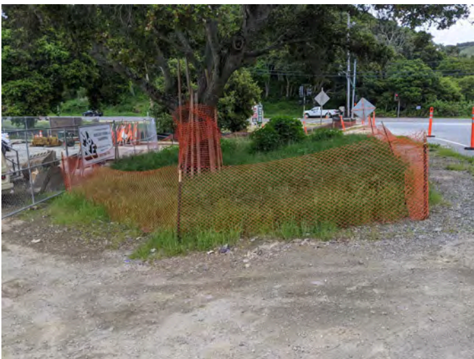
View of ESA fencing surrounding protected oak tree adjacent to staging yard
