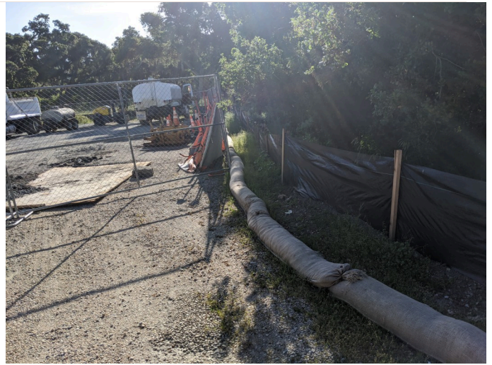
Intact silt fencing surrounding staging area.
