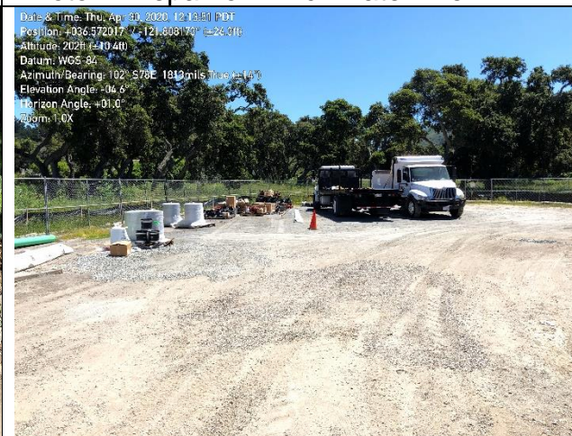
Photo 4. Silt fence around staging area in good condition
