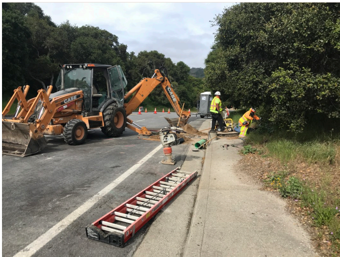
Installation of ARV along Ragsdale Rd at Station 18+00
