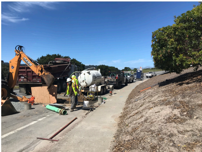
MPE repairing leak in pipeline along Lower Ragsdale Rd.
