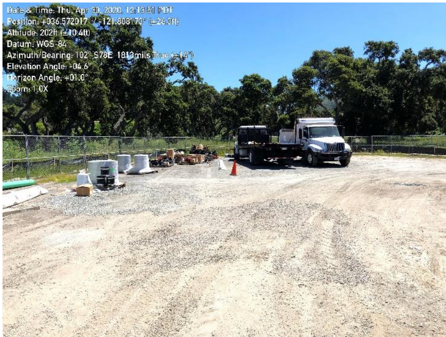
Photo 4. Silt fence around staging area in good condition.
