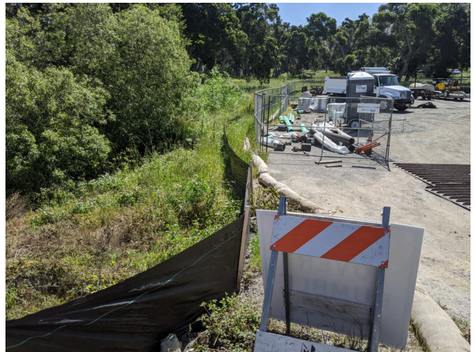
Intact silt fencing surrounding staging yard.
