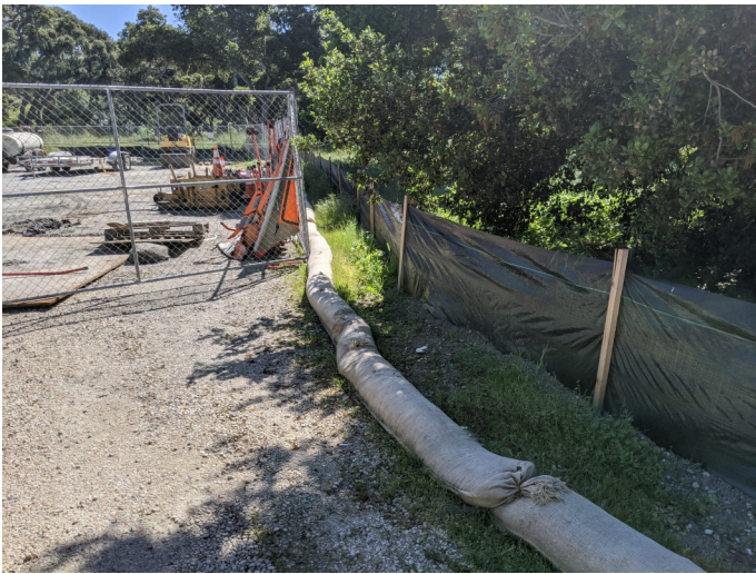
Intact silt fencing surrounding staging yard.
