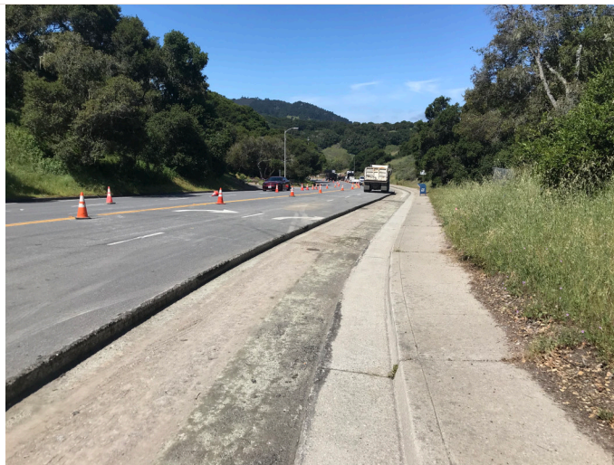
MPE repaving along Ragsdale Rd
