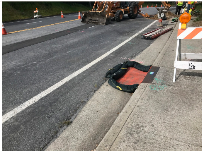
BMPs along Ragsdale Rd during the installation of ARV
