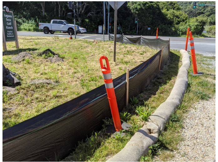
Intact silt fencing surrounding staging yard.
