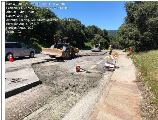
Photo 1. MPE paving on Ragsdale Drive
