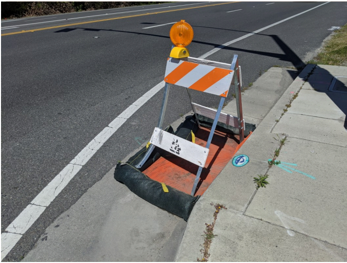
BMP in use adjacent to construction
