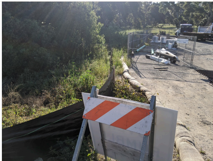
Intact silt fencing surrounding staging area.
