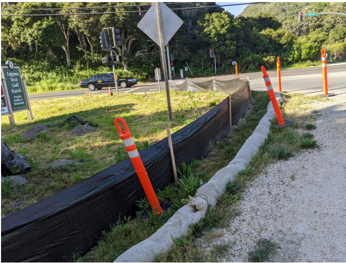
Intact silt fencing surrounding staging area.
