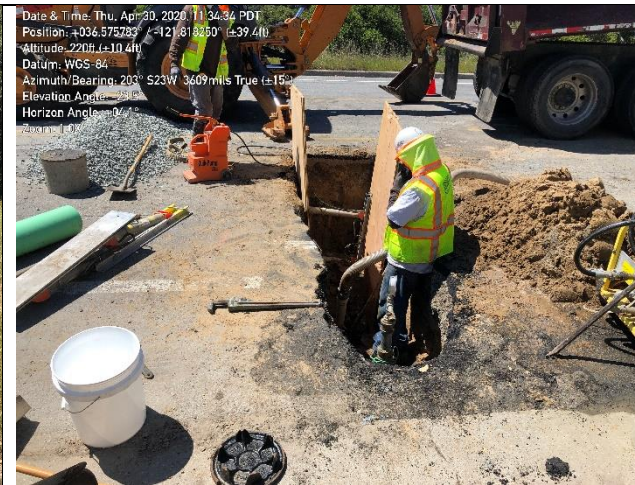
Photo 2. Repair of 2-inch water line
