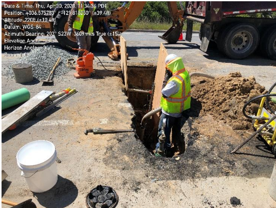
Photo 2. Repair of 2-inch water line.
