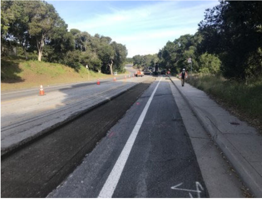
05/06/2020 - MPE grinding/paving along Lower Ragsdale Drive.
