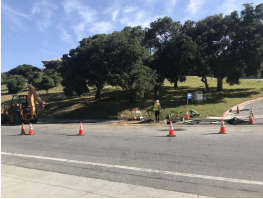
05/01/2020 - MPE repairing alignment leak along Wilson Road.
