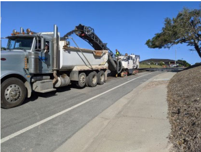
05/04/2020 - MPE grinding/paving along Lower Ragsdale Drive.
