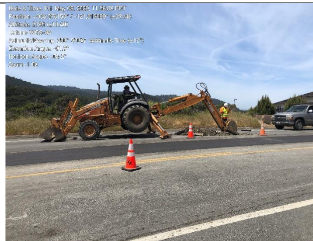
Photo 2. MPE paving repairs on Lower Ragsdale Drive
