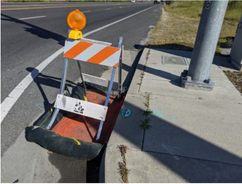
05/04/2020 - Intact stormwater BMPs in use adjacent to construction along Ragsdale Drive.
