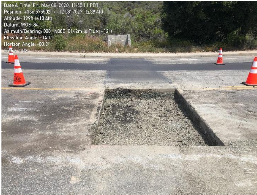
Photo 1. MPE paving repairs on Lower Ragsdale Drive.
