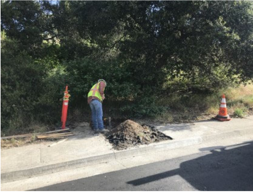
05/06/2020 - MPE installing ARV pad along Ragsdale Drive.
