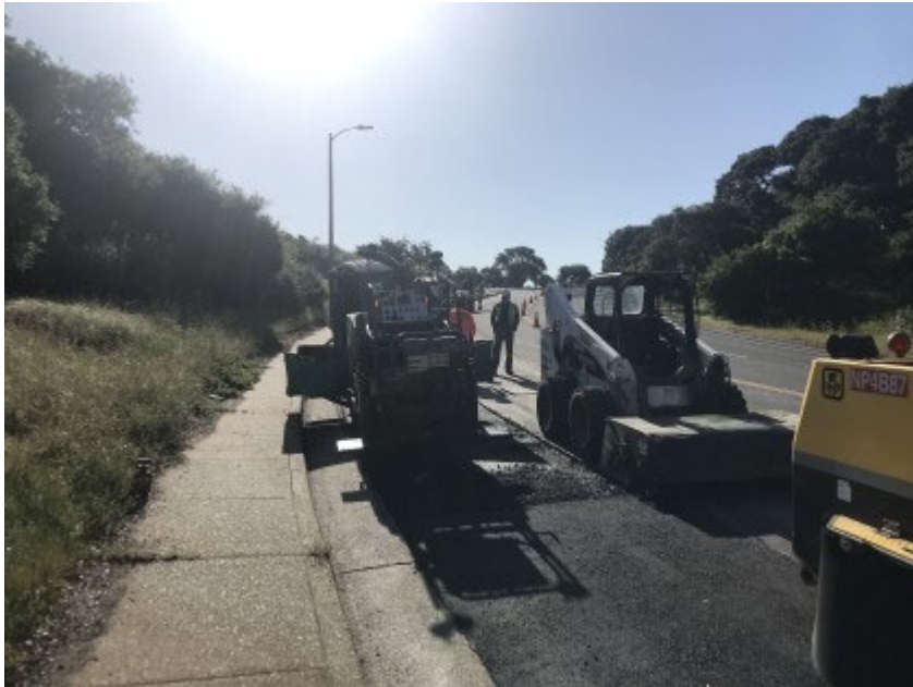
05/01/2020 - MPE grinding/paving along Ragsdale Drive.
