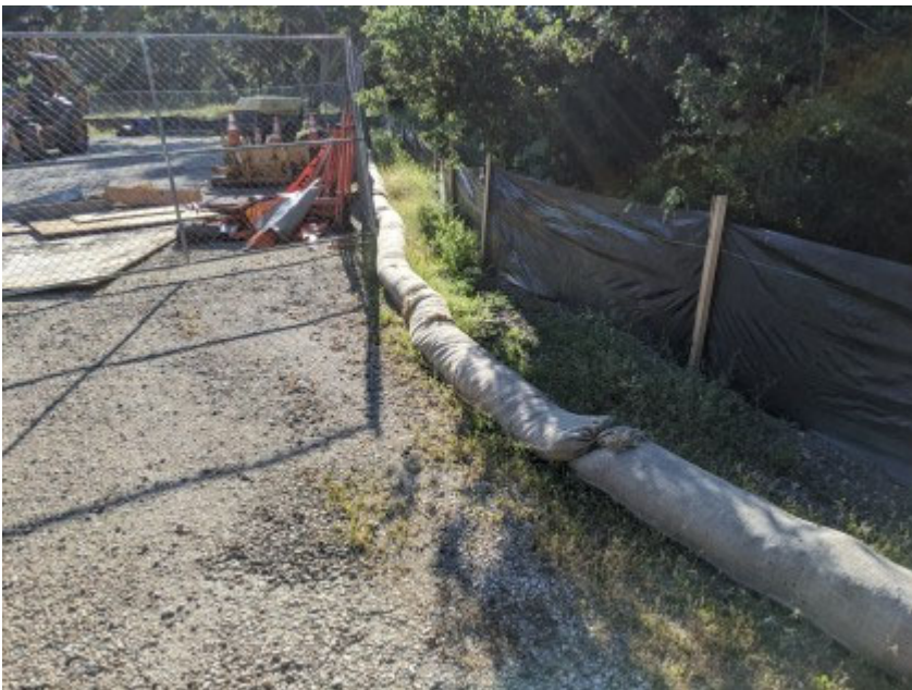
05/04/2020 - Intact silt fencing surrounding staging area.
