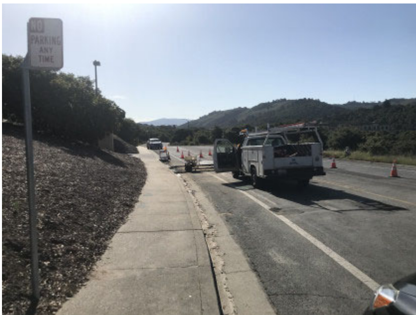
05/01/2020 - MPE repairing alignment leak along Lower Ragsdale Drive.
