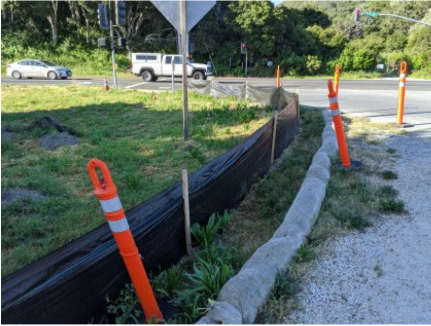
05/04/2020 - Intact silt fencing surrounding staging area.
