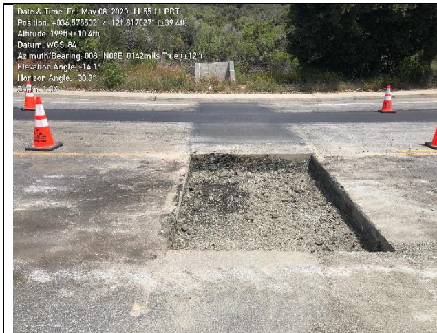
Photo 1. MPE paving repairs on Lower Ragsdale Drive
