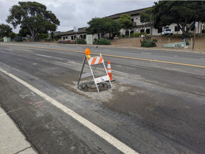
Excavation of AC along alignment in preparation for concrete pouring.
