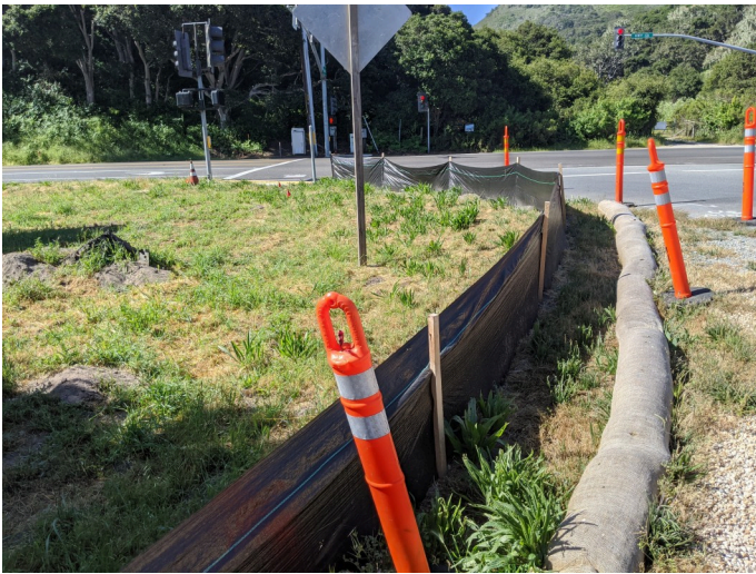
Intact silt fencing surrounding staging area.
