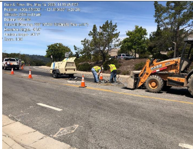
Photo 2. MPE paving repairs on Lower Ragsdale Drive
