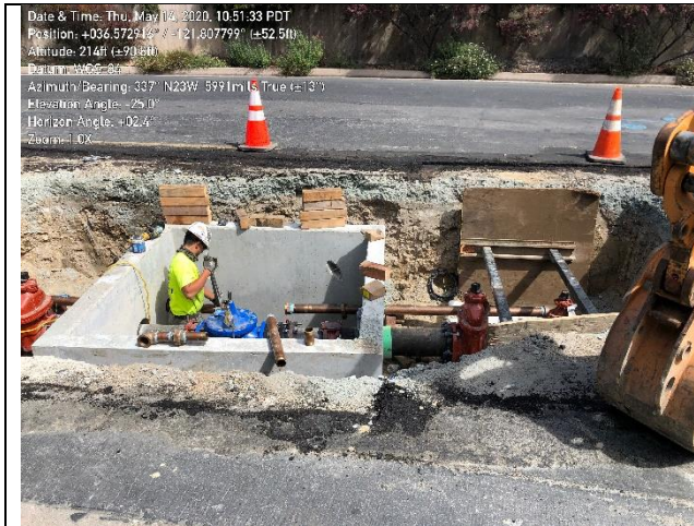
Photo 1. MPE excavation on Blue Larkspur Lane.
