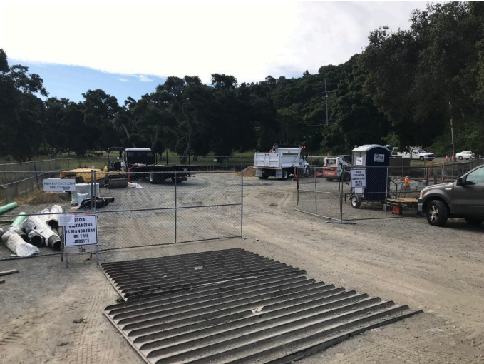
MPE staging area at the corner of Highway 68 and York Rd
