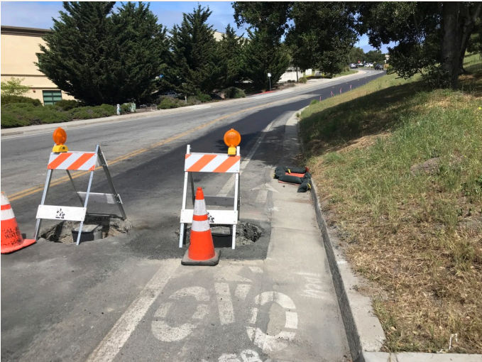
BMPs installed adjacent to work area along Wilson Rd
