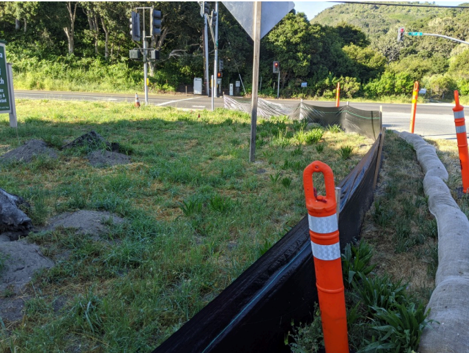
Intact silt fencing surrounding staging area.
