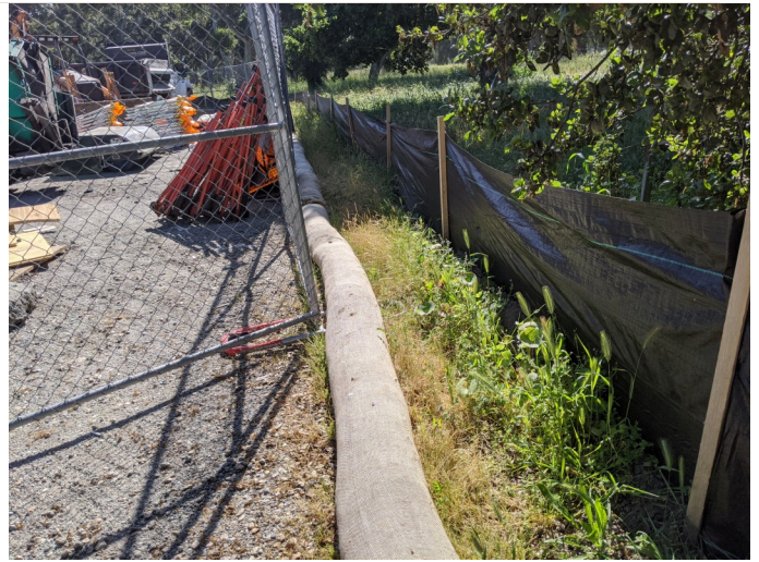
Intact silt fencing surrounding staging area.
