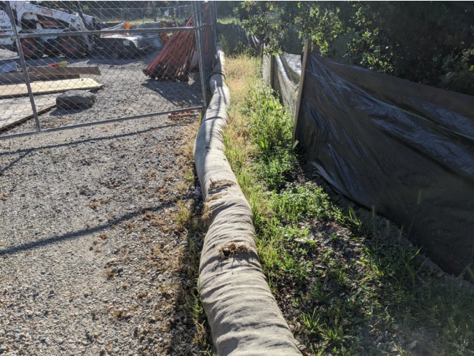
Intact silt fencing surrounding staging area.
