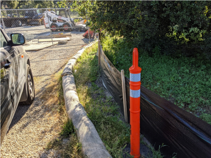
Intact silt fencing surrounding staging area.
