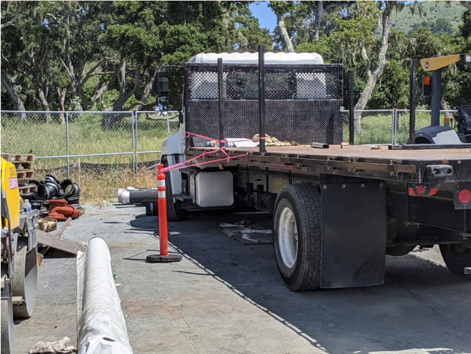
Intact exclusionary flagging around identified black phoebe nest in staging area.
