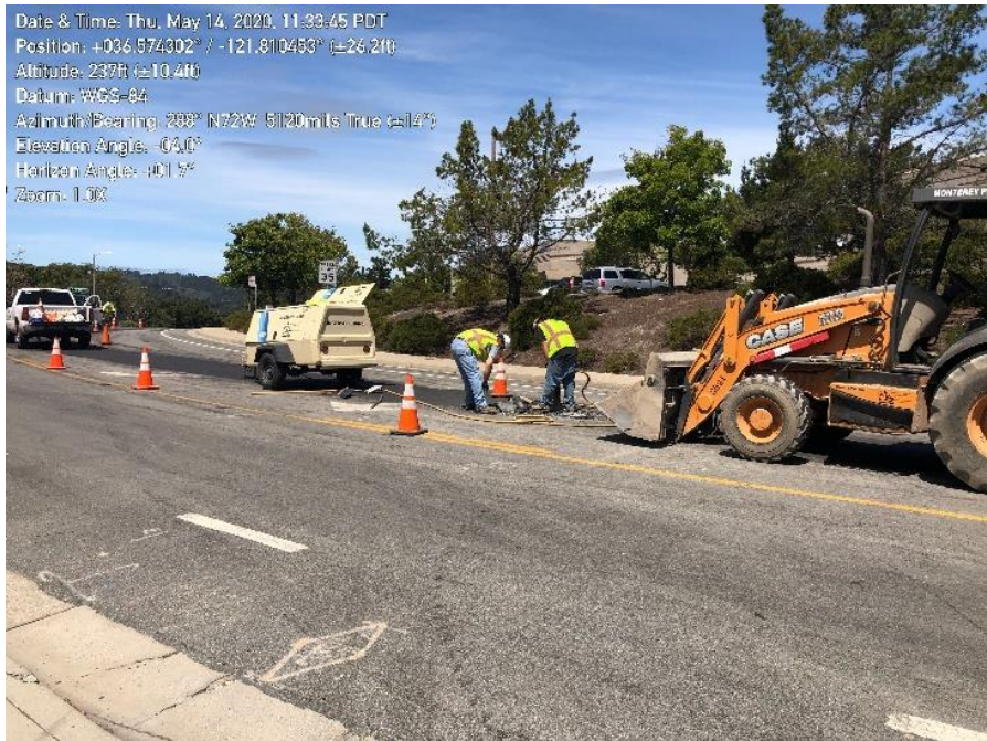
Photo 2. MPE paving repairs on Lower Ragsdale Drive.
