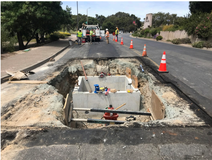
MPE installing connection on Blue Larkspur Ln
