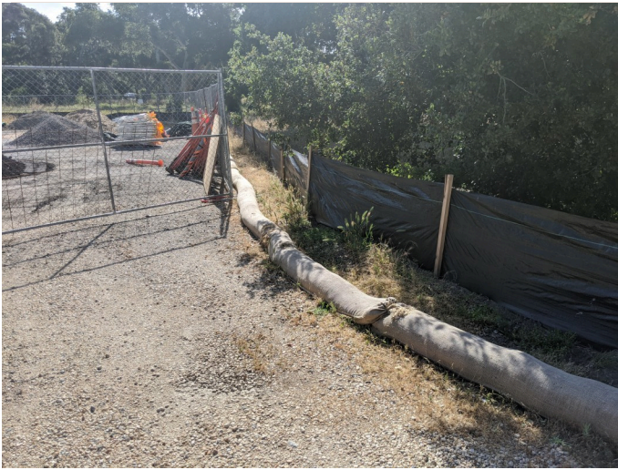
Intact silt fencing surrounding staging area.
