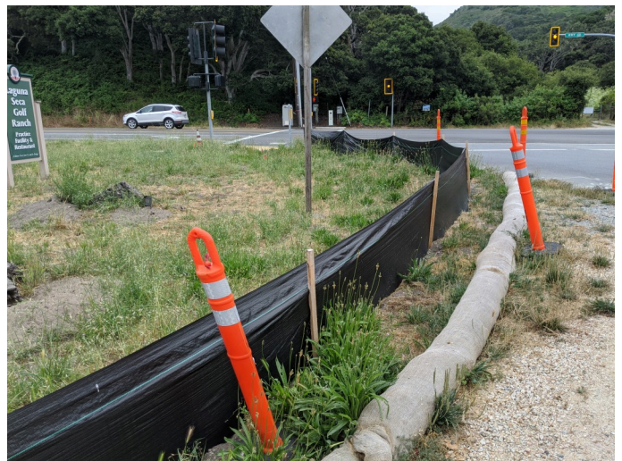
Intact silt fencing surrounding staging area.
