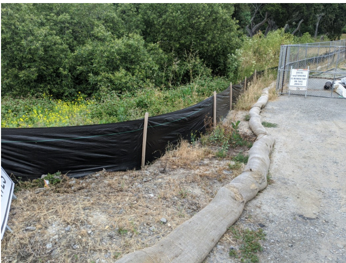
Intact silt fencing surrounding staging area.
