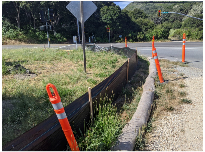
Intact silt fencing surrounding staging area.
