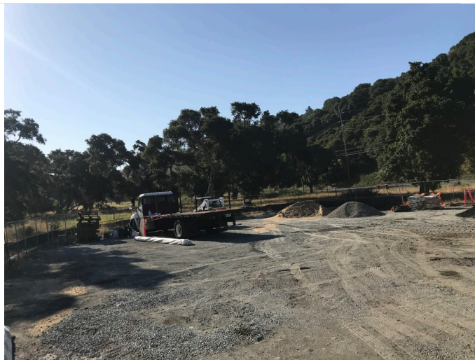
MPE staging area at the corner of Highway 68 and York Road
