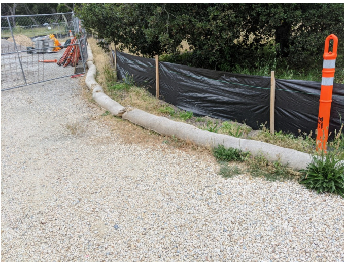
Intact silt fencing surrounding staging area.
