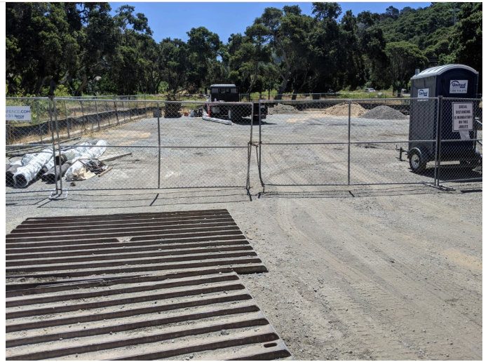
Gate locked, confirmed no work during monitoring period.
