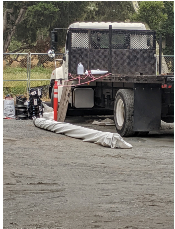
Intact exclusionary flagging surrounding protected black phoebe nest within staging area.
