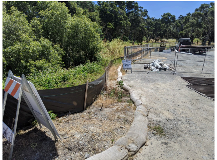
Intact silt fencing surrounding staging area.
