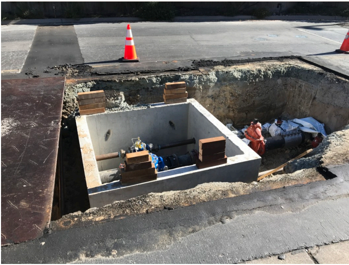
MPE installing pipe supports along Blue Larkspur Ln
