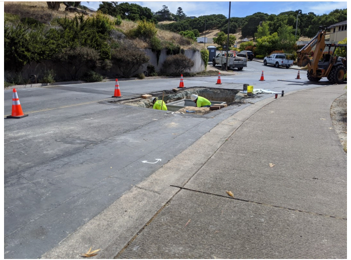
Vault installation on Blue Larkspur Lane.
