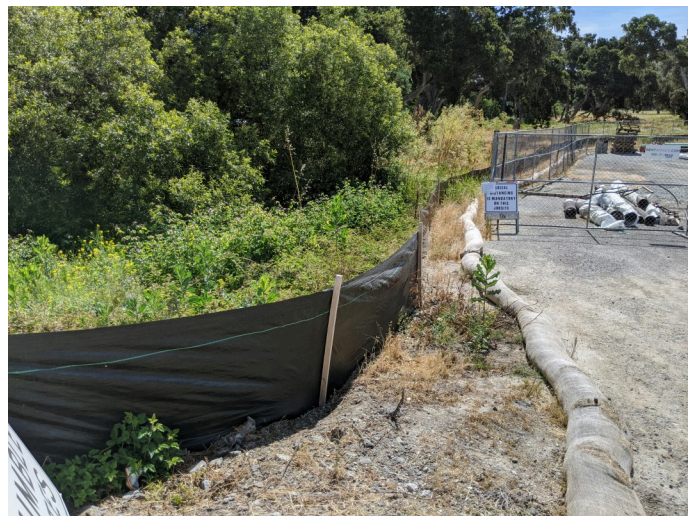
Intact silt fencing surrounding staging area.
