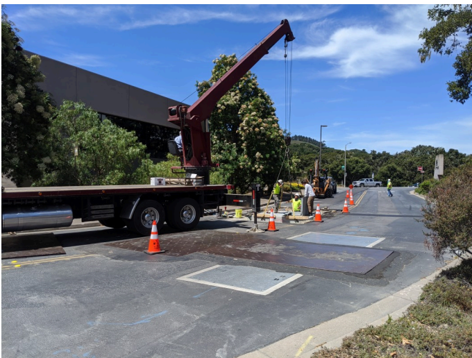
Vault installation on Blue Larkspur Lane.
