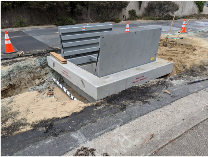
Vault installation on Blue Larkspur Lane.
