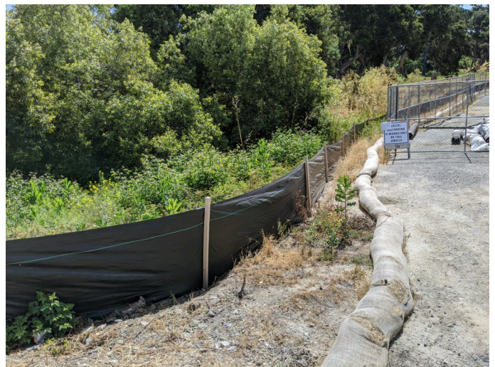
Intact silt fencing surrounding staging area.
