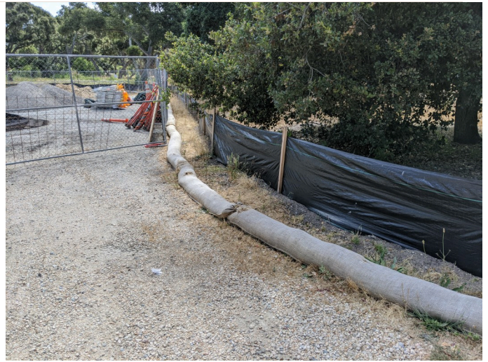
Intact silt fencing surrounding staging area.
