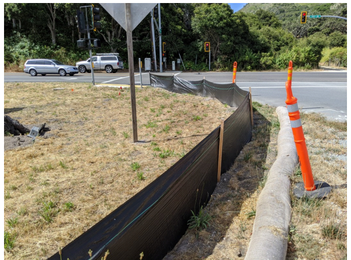
Intact silt fencing surrounding staging area.
