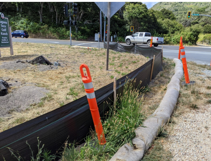
Intact silt fencing surrounding staging area.
