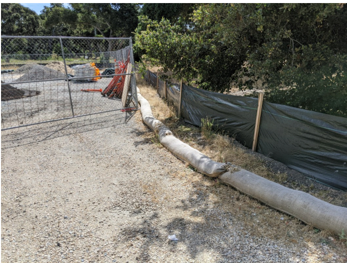
Intact silt fencing surrounding staging area.
