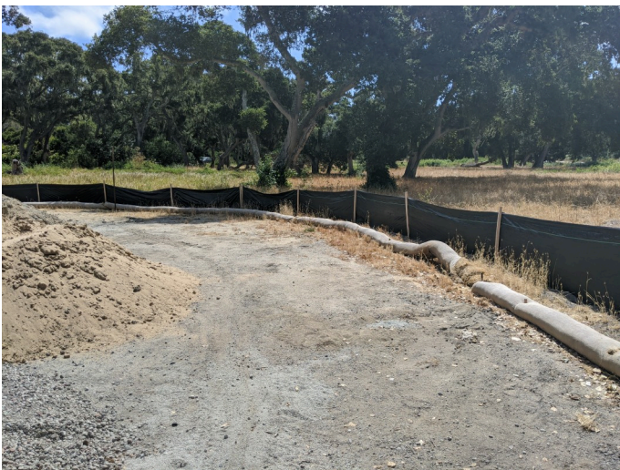
Intact silt fencing surrounding staging area.
