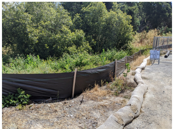
Intact silt fencing surrounding staging area.
