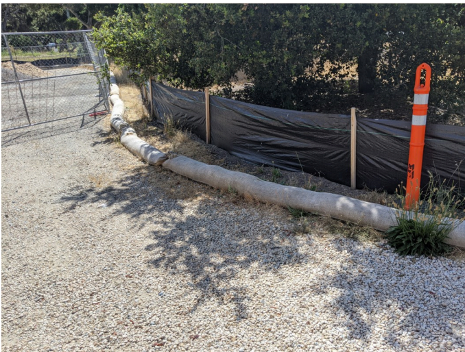
Intact silt fencing surrounding staging area.
