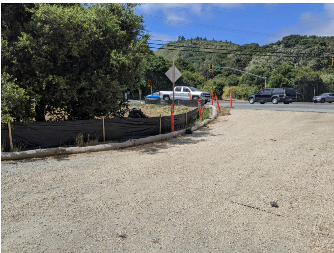
Intact silt fencing surrounding staging area.
