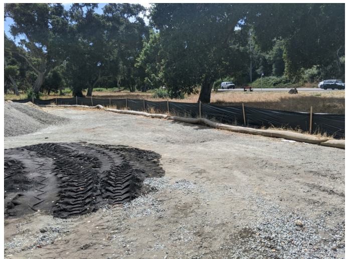
Intact silt fencing surrounding staging area.
