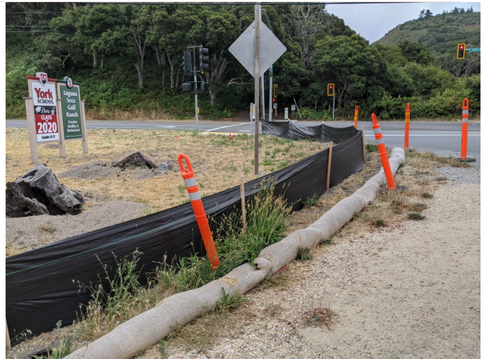
Intact silt fencing surrounding staging area.
