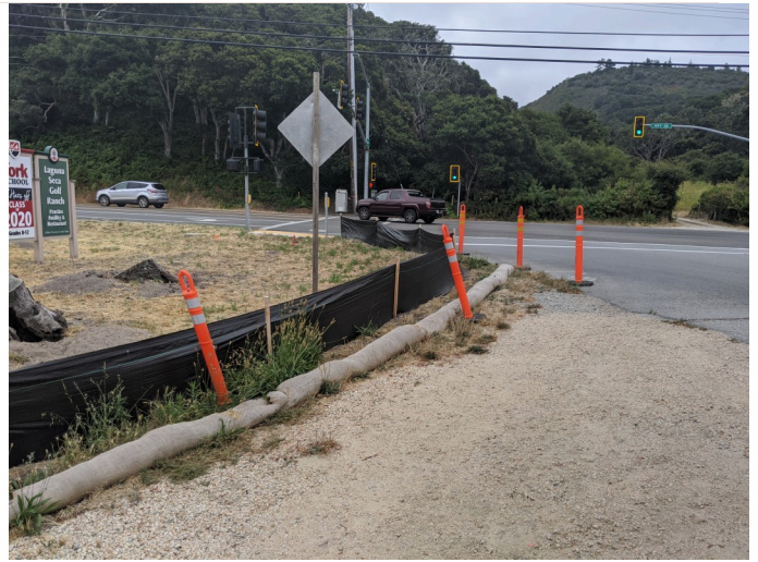
Intact silt fencing surrounding staging area.
