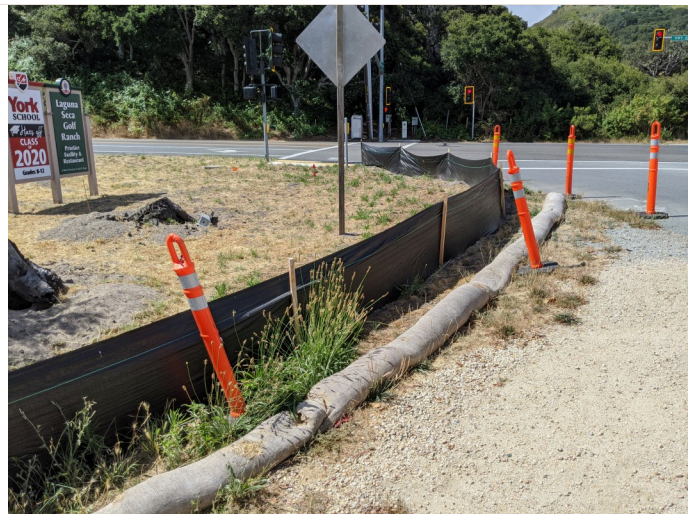
Intact silt fencing surrounding staging area.
