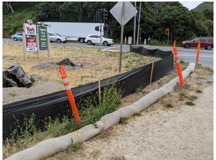
Intact silt fencing surrounding staging area.
