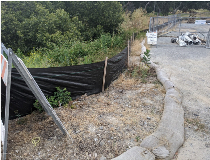
Intact silt fencing surrounding staging area.
