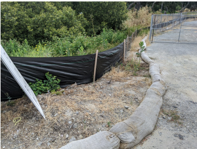
Intact silt fencing surrounding staging area.
