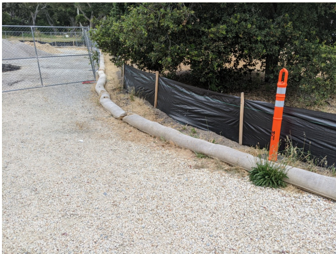
Intact silt fencing surrounding staging area.
