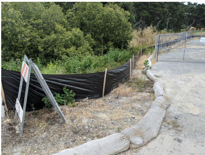
Intact silt fencing surrounding staging area.
