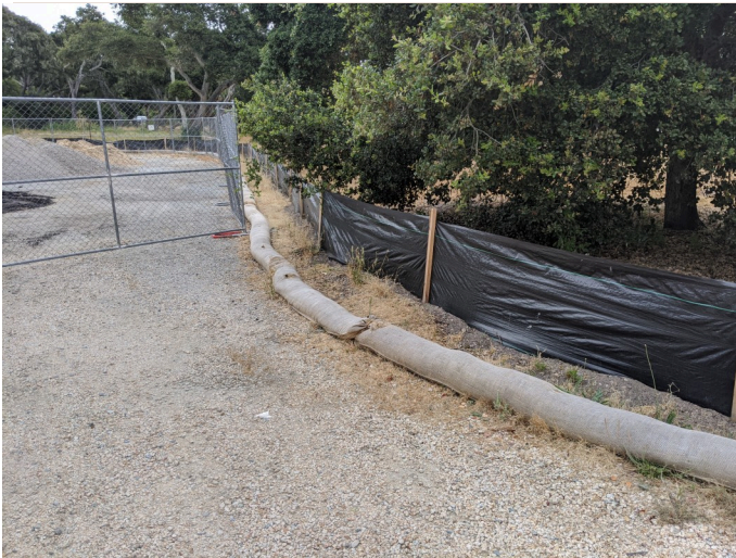
Intact silt fencing surrounding staging area.
