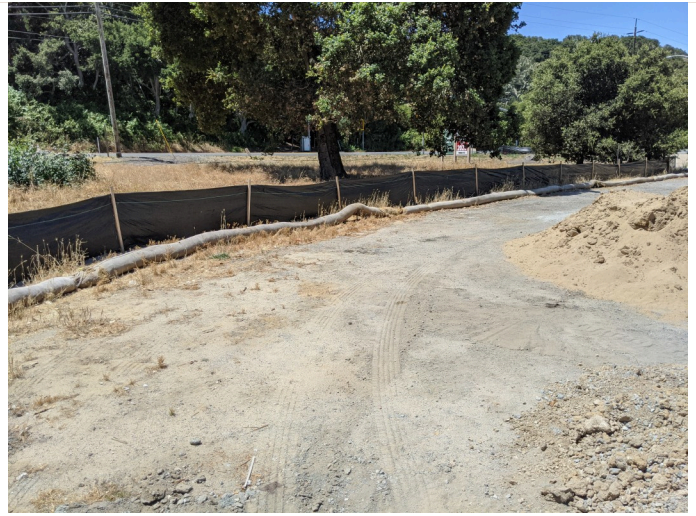
Intact silt fencing surrounding staging area.
