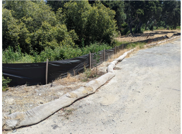
Intact silt fence surrounding staging area.
