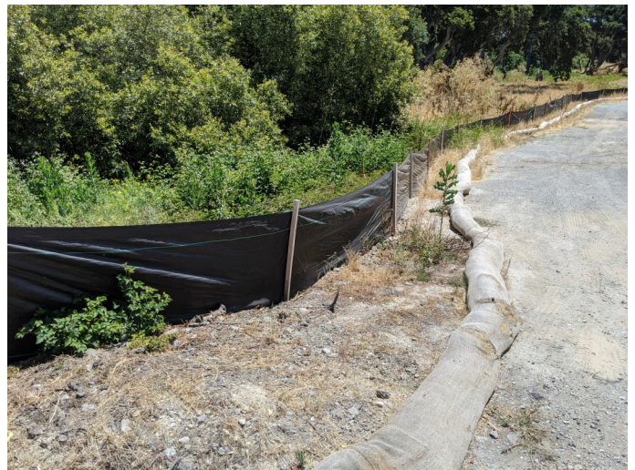
Intact silt fencing surrounding staging area.
