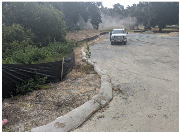
Intact silt fence surrounding staging area.
