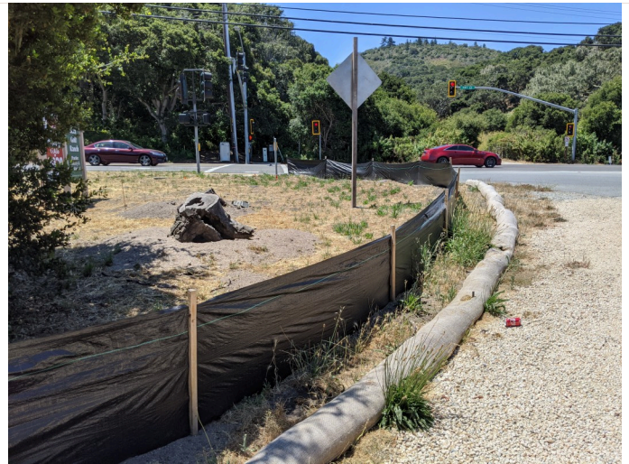
Intact silt fencing surrounding staging area.
