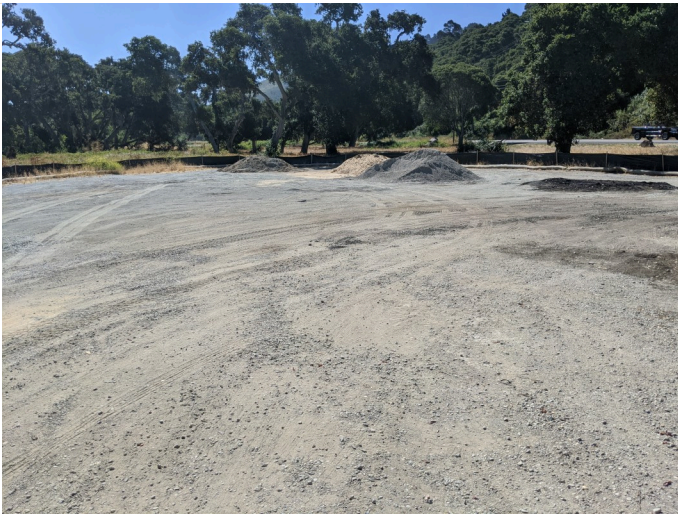
Intact silt fencing surrounding staging area.
