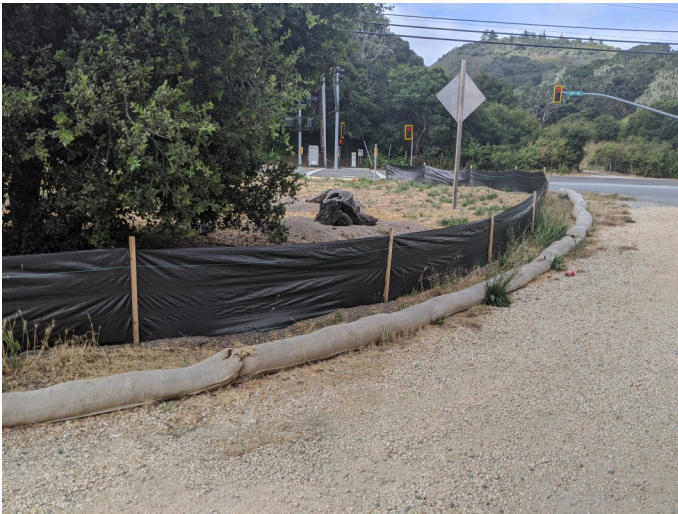
Intact silt fence surrounding staging area.
