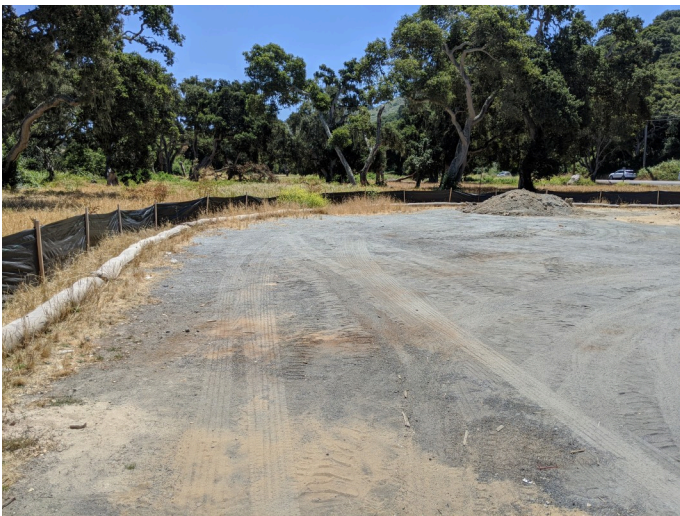
Intact silt fencing surrounding staging area.
