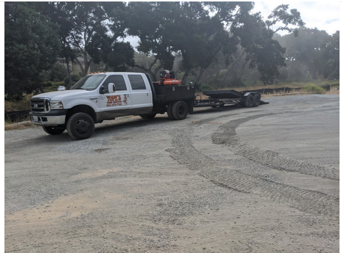
Topes tree service on site performing vegetation clearance around staging area.
