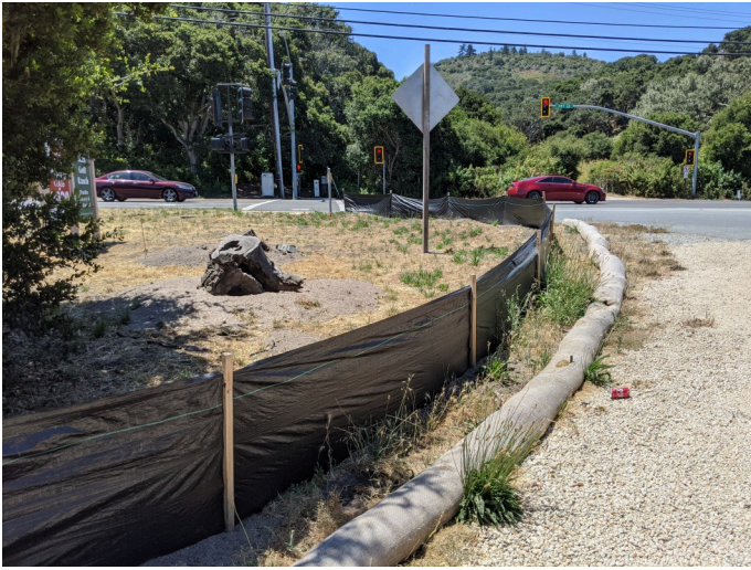
Intact silt fencing surrounding staging area.
