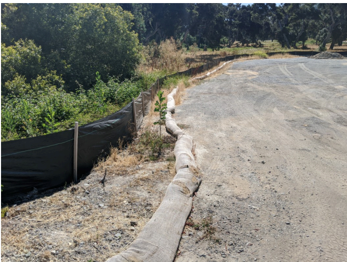
Intact silt fence surrounding staging area.
