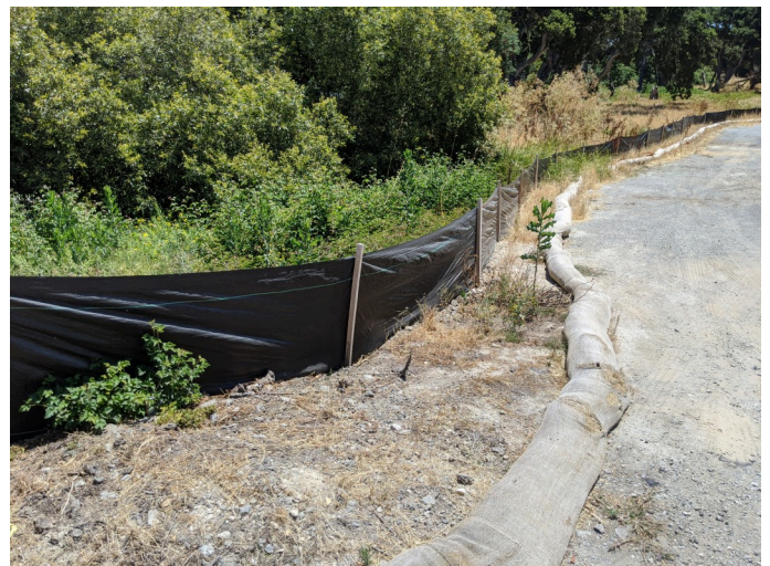
Intact silt fencing surrounding staging area.
