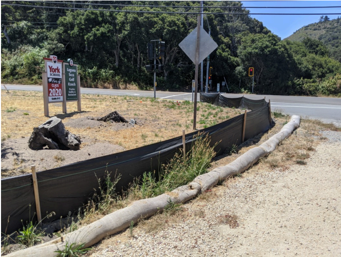
Intact silt fence surrounding staging area.
