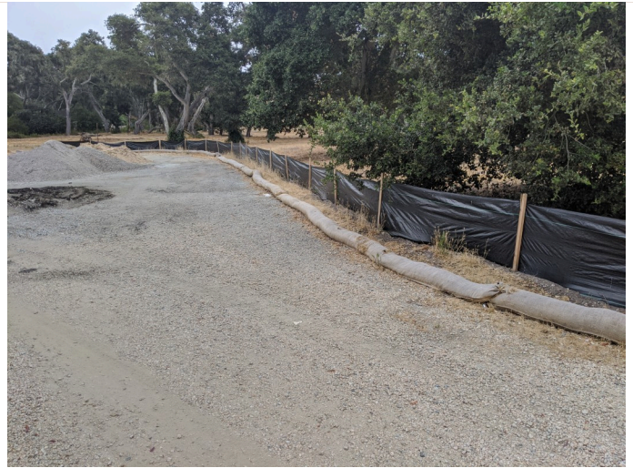
Intact silt fencing surrounding staging area.
