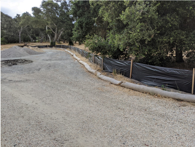
Intact silt fencing surrounding staging area.
