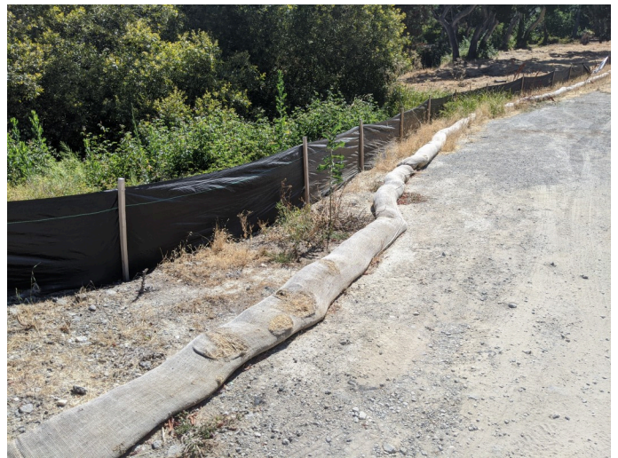
Intact silt fencing surrounding staging area.
