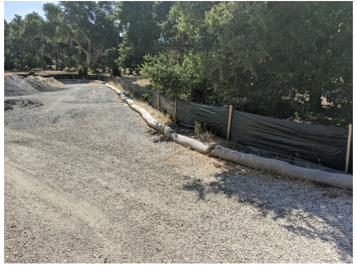
Intact silt fence surrounding staging area.
