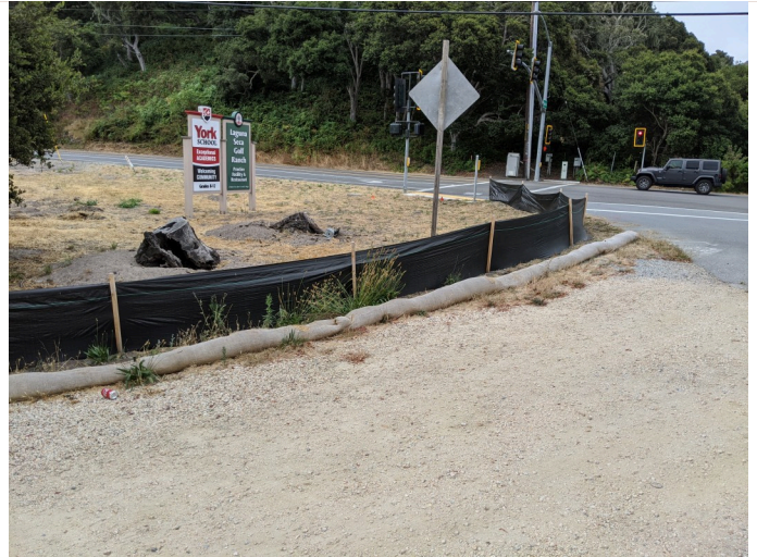
Intact silt fencing surrounding staging area.
