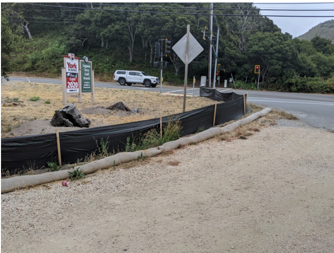
Intact silt fencing surrounding staging area.
