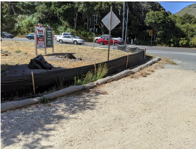
Intact silt fence surrounding staging area.
