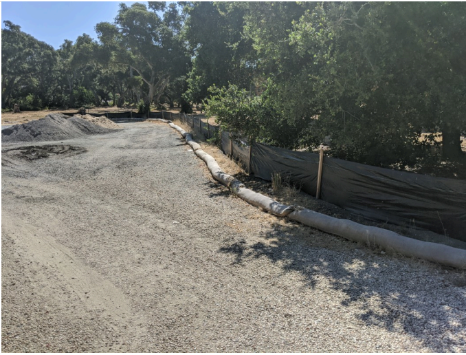
Intact silt fencing surrounding staging area.
