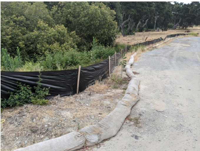
Intact silt fencing surrounding staging area.
