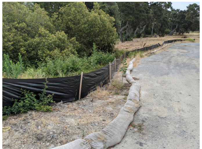
Intact silt fencing surrounding staging area.
