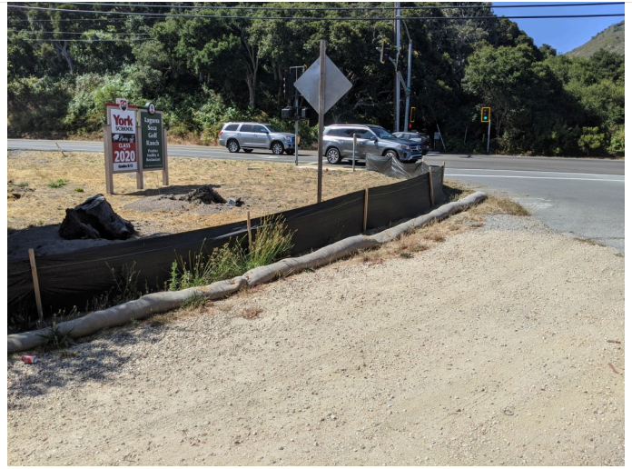
Intact silt fencing surrounding staging area.
