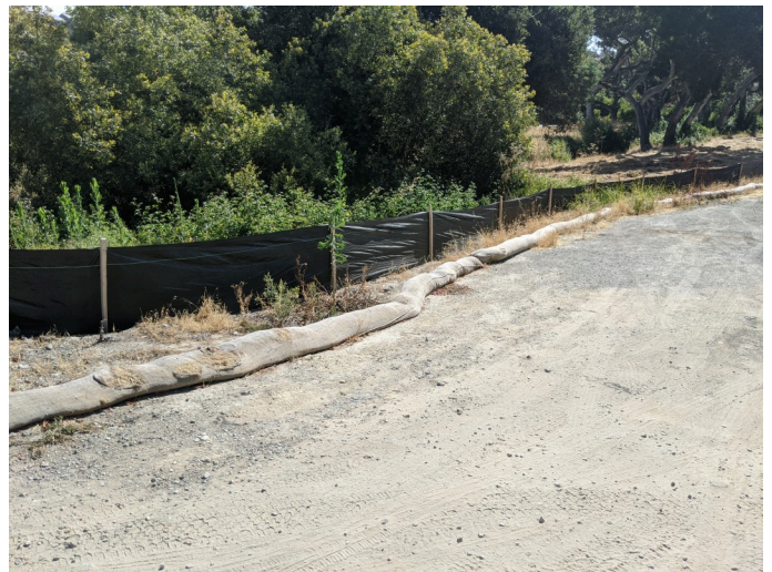
Intact silt fence surrounding staging area.
