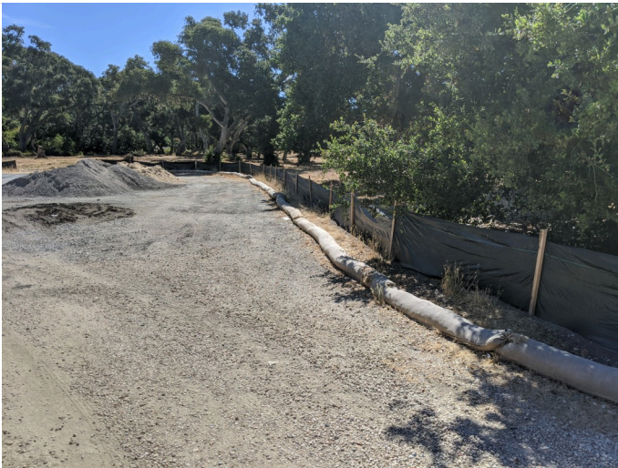
Intact silt fencing surrounding staging area.
