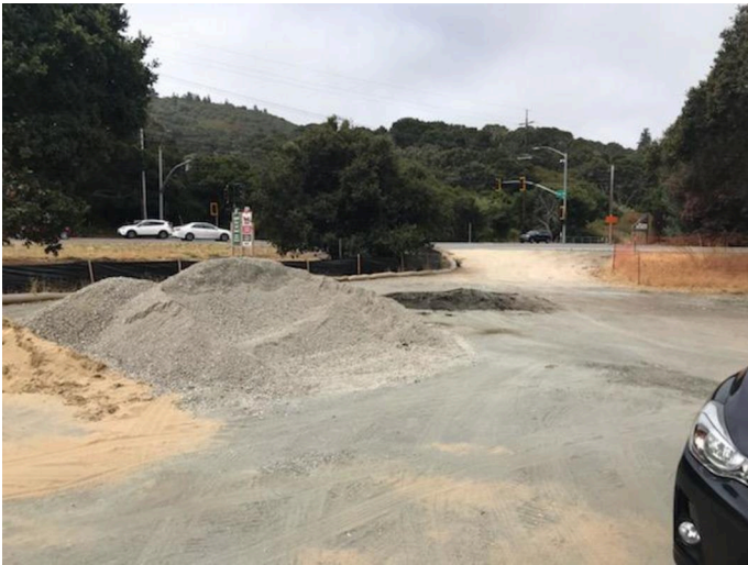
Inactive staging area.
