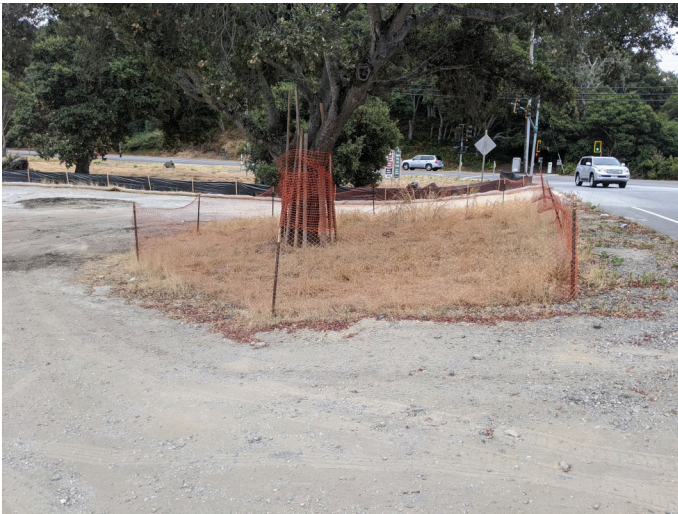
Intact ESA fencing surrounding protected oak tree adjacent to staging area.
