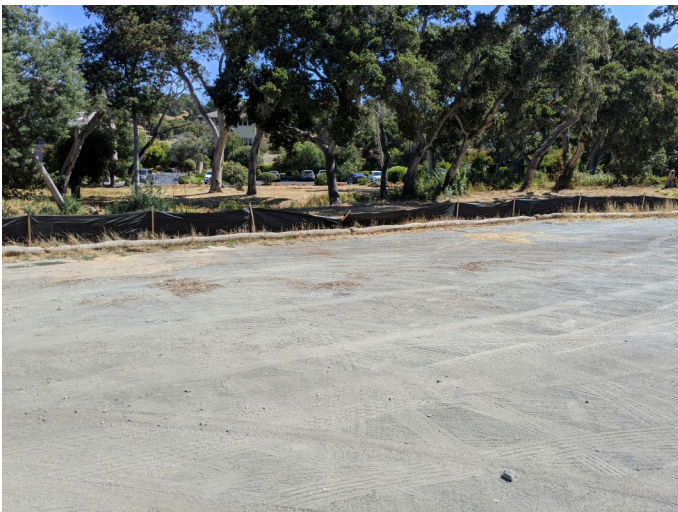
View of repaired silt fencing surrounding staging area.
