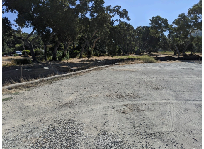
Intact silt fencing surrounding staging area.
