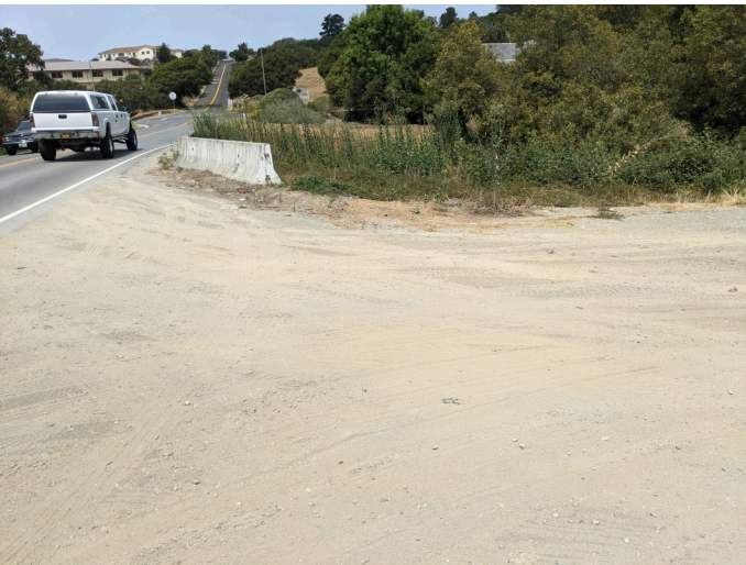
Silt fencing surrounding staging area removed.
