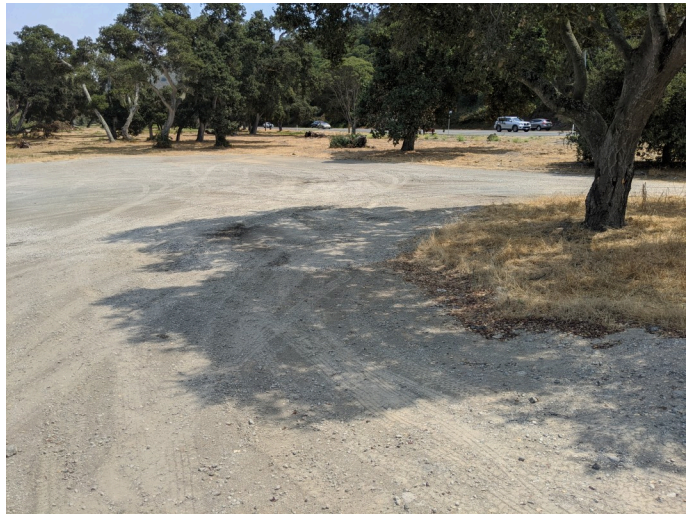
Silt fencing surrounding staging area removed.
