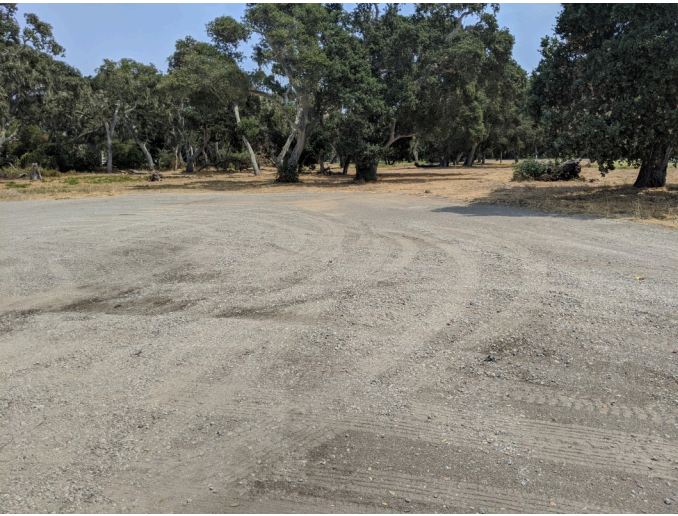
Stored materials removed from staging area.
