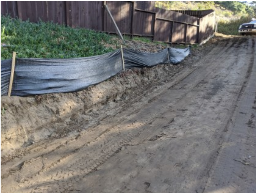
09/25/2020 - Repaired exclusionary fencing surrounding construction area.
