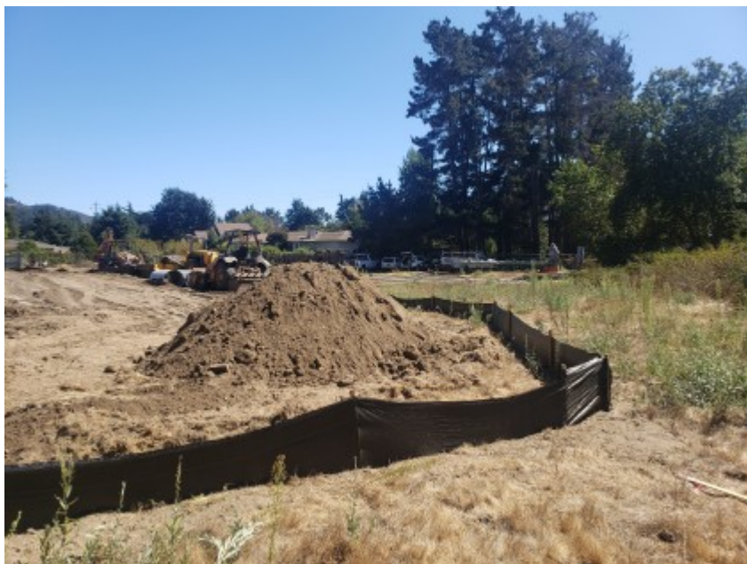
09/24/2020 - View of exclusionary fencing.
