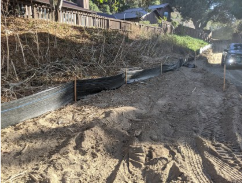
09/25/2020 - Repaired exclusionary fencing surrounding construction area.
