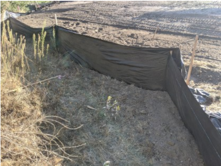
09/25/2020 - Repaired exclusionary fencing surrounding construction area.
