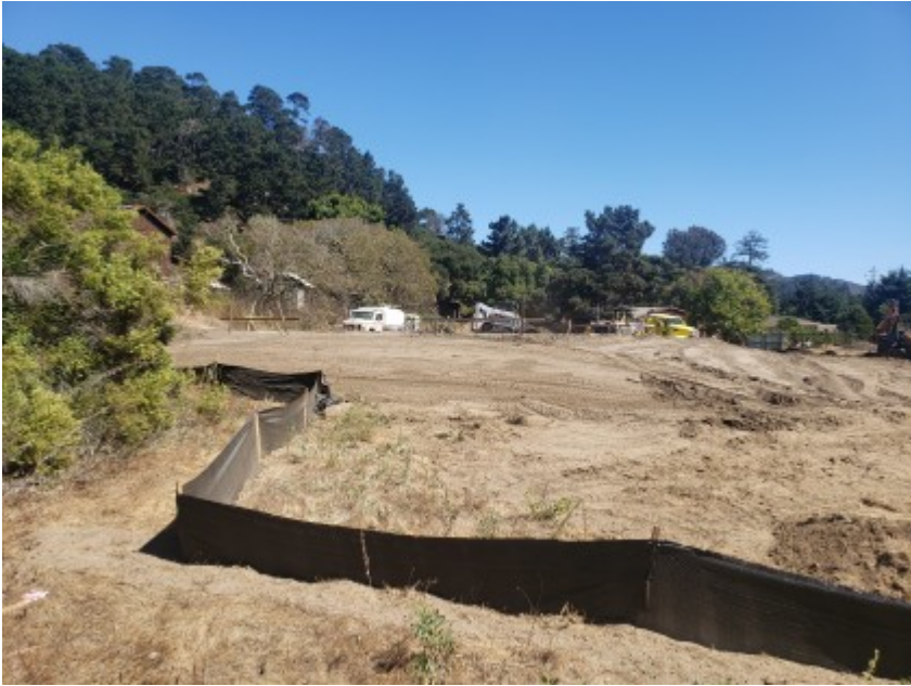
09/24/2020 - View of exclusionary fencing.
