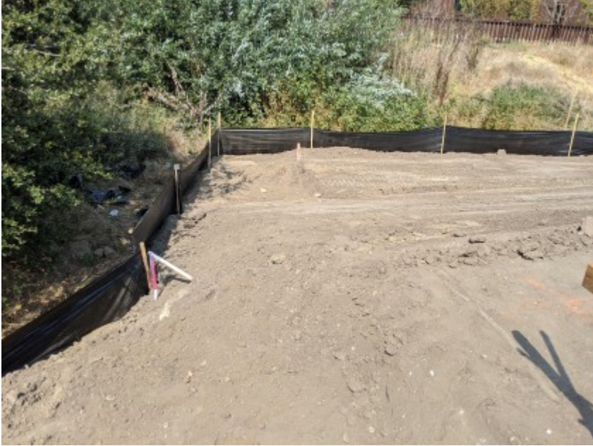
09/28/2020 - Intact exclusionary fencing surrounding construction area.
