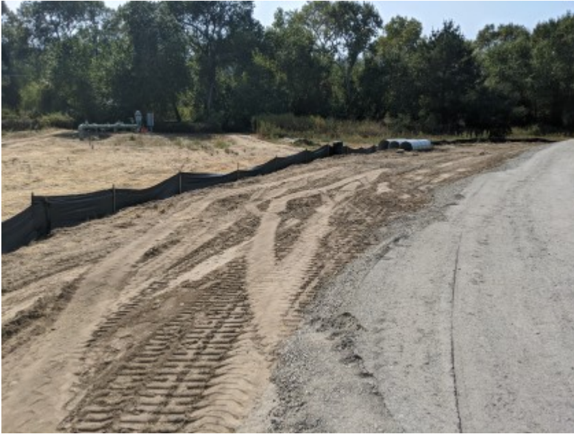
09/28/2020 - Intact exclusionary fencing surrounding construction area.
