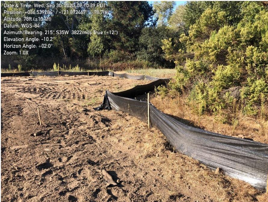
Photo 1. Silt fence repaired and in good condition.
