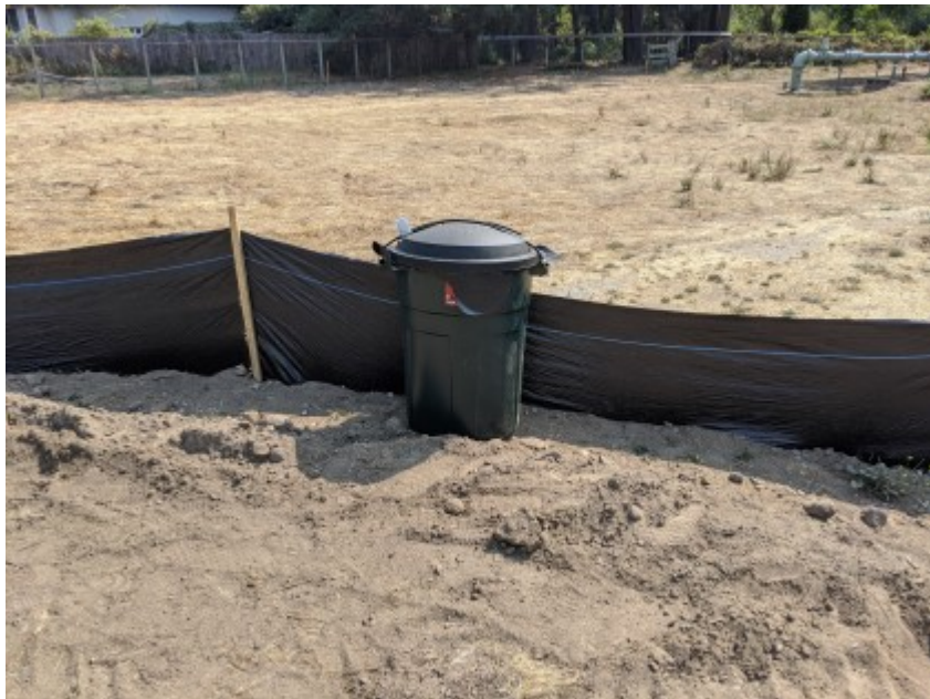
09/28/2020 - Confirmed trash receptacle on-site.
