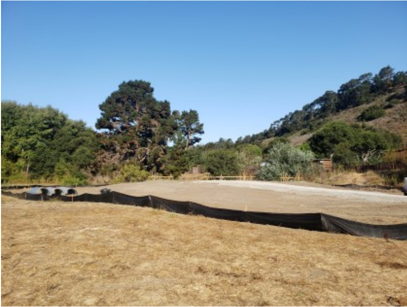
09/30/2020 - Overall site conditions.
