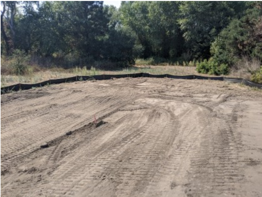
09/28/2020 - Intact exclusionary fencing surrounding construction area.
