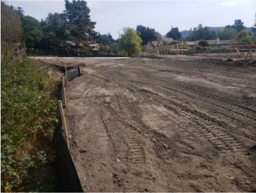
10/08/2020 - Typical site conditions
