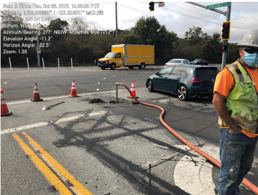
Photo 3. Ryan Ranch – Bishop Interconnection Improvements: MPE cleaning installed pipeline.
