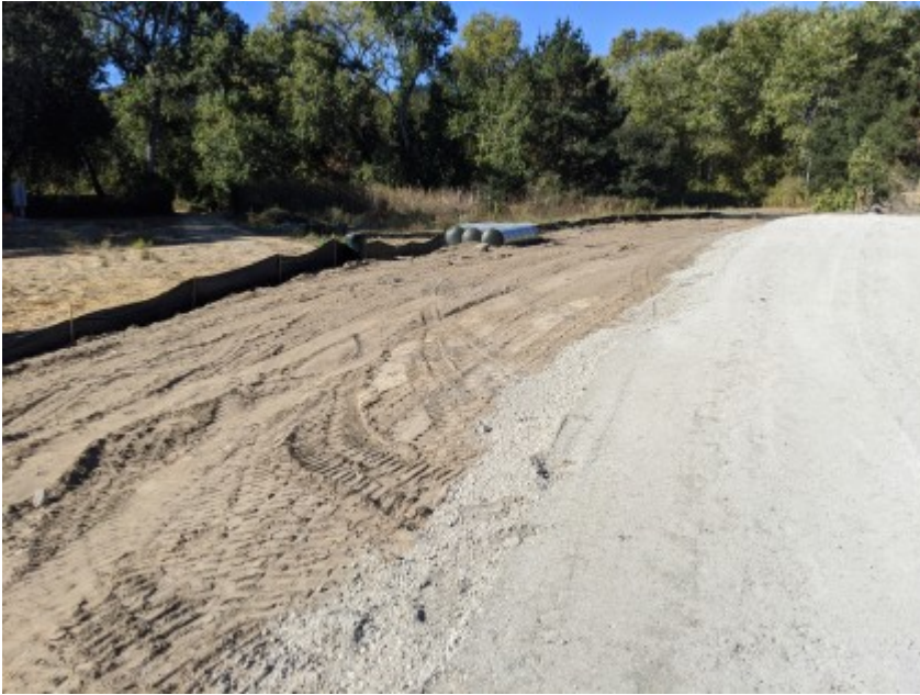
10/12/2020 - Intact exclusionary fencing surrounding construction area.
