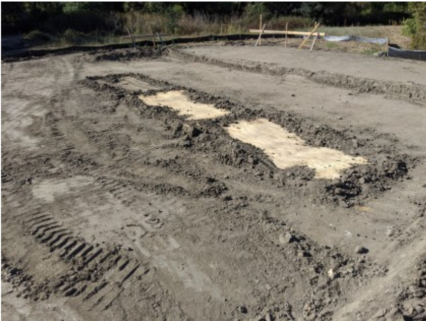
10/12/2020 - Properly installed pit coverings
