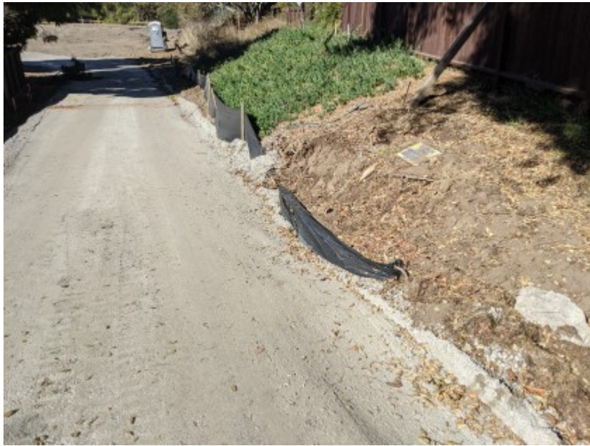
10/12/2020 - Exclusionary fencing by site entrance in need of repair.
