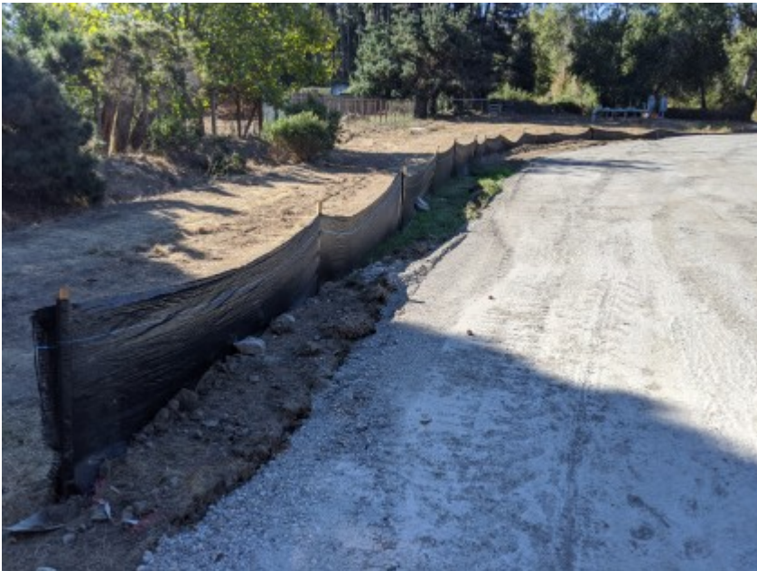
10/12/2020 - Intact exclusionary fencing surrounding construction area.
