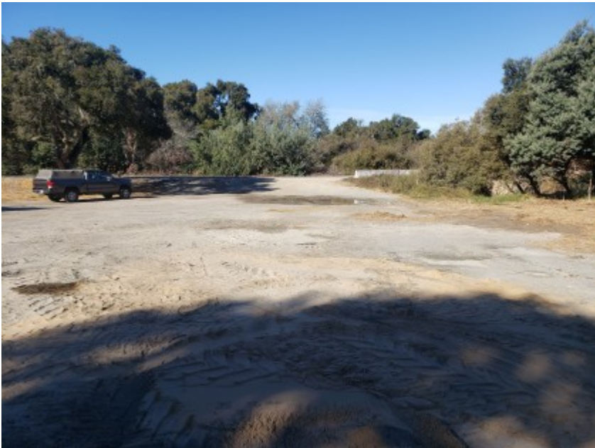
11/10/2020 - Staging area cleared.
