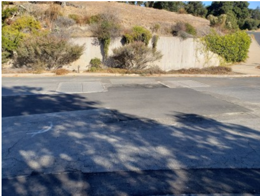
11/10/2020 - Tie in location at Blue Larkspur.
