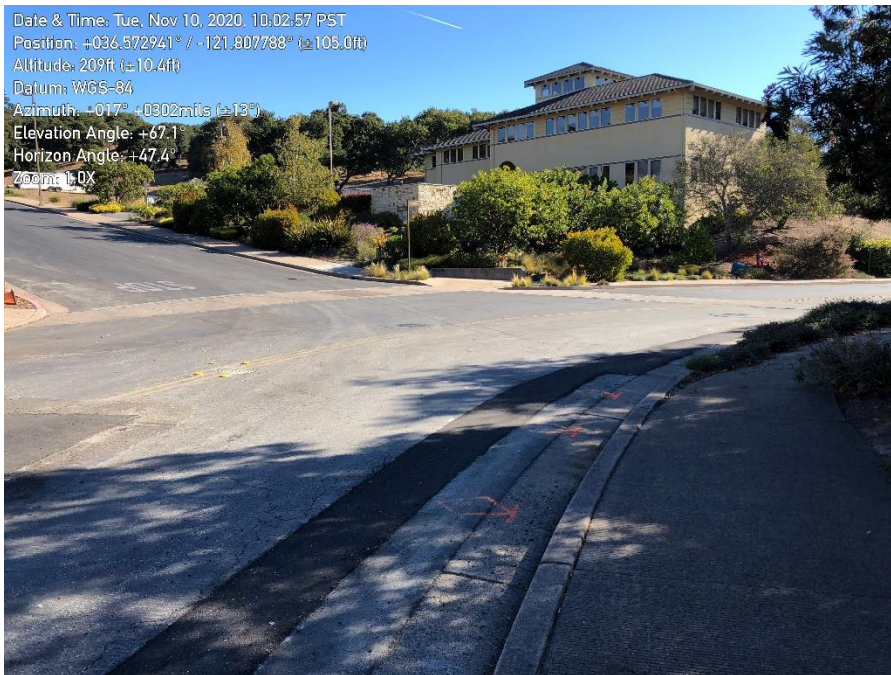
Photo 4. Ryan Ranch – Bishop Interconnection Improvements: Trenching along Blue Larkspur Lane complete.
