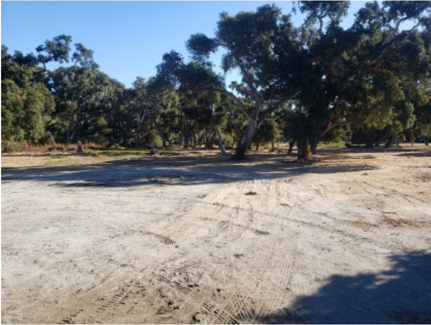
11/10/2020 - Staging area cleared.
