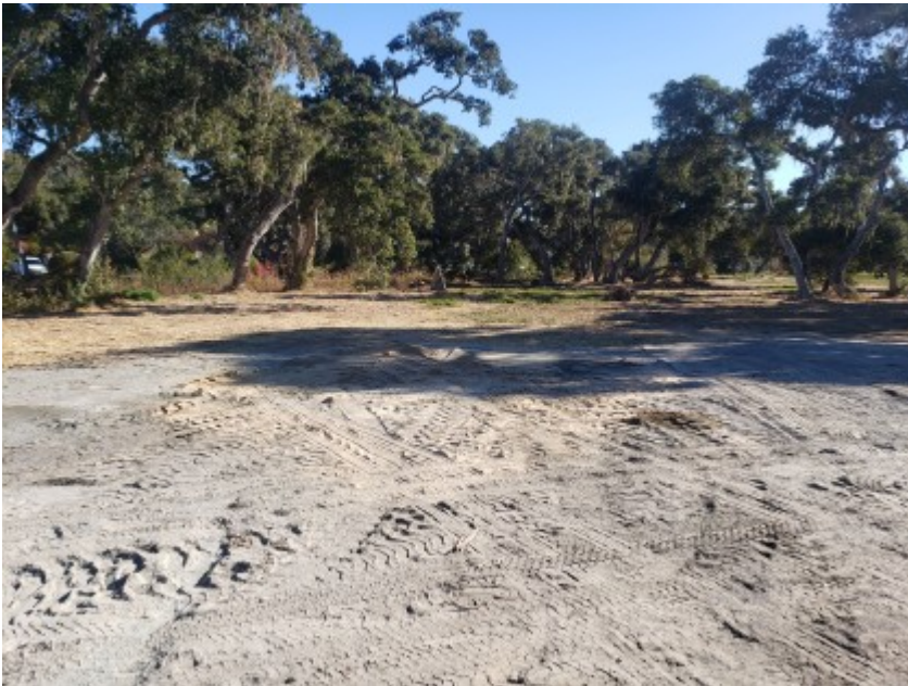
11/10/2020 - Staging area cleared.
