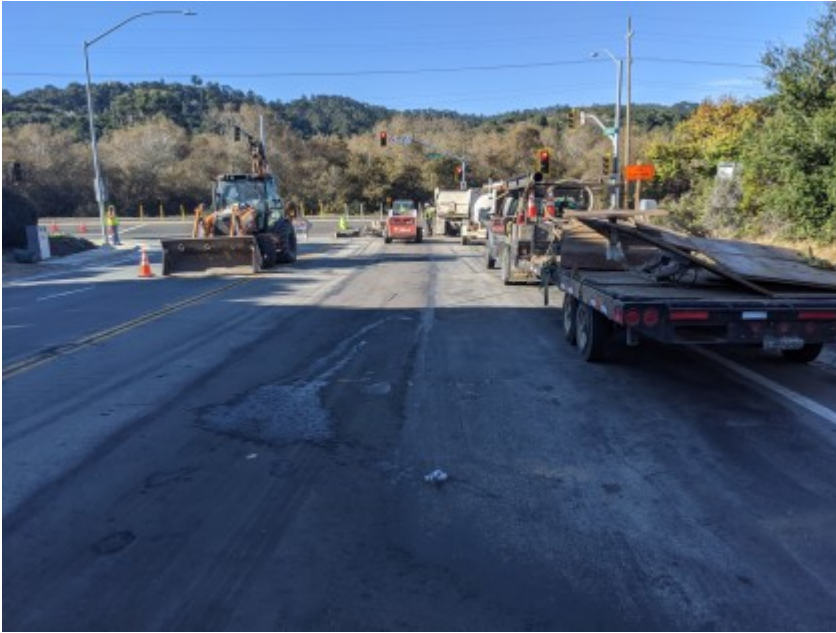
11/09/2020 - Tie-in work at Ragsdale Drive and Hwy 68.
