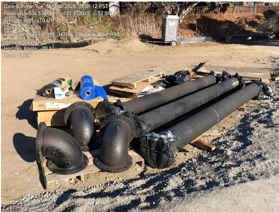
Photo 2. Carmel Valley Pump Station: ends of pipes covered.
