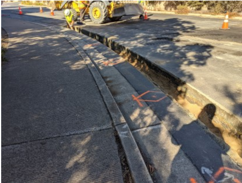
11/09/2020 - Installation of electrical conduit along Blue Larkspur Lane.
