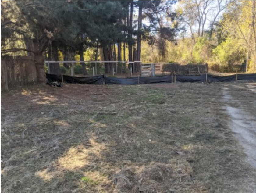
12/07/2020 - Intact silt fencing surrounding work area.
