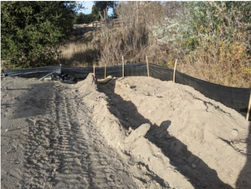
12/10/2020 - Intact silt fencing surrounding work area.
