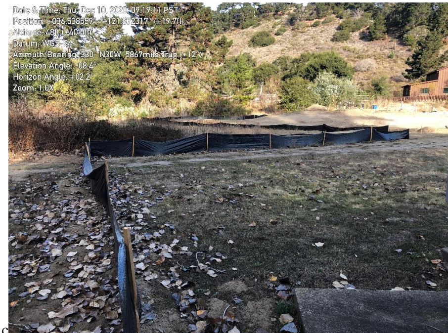
Photo 2. Silt fence in adequate condition.
