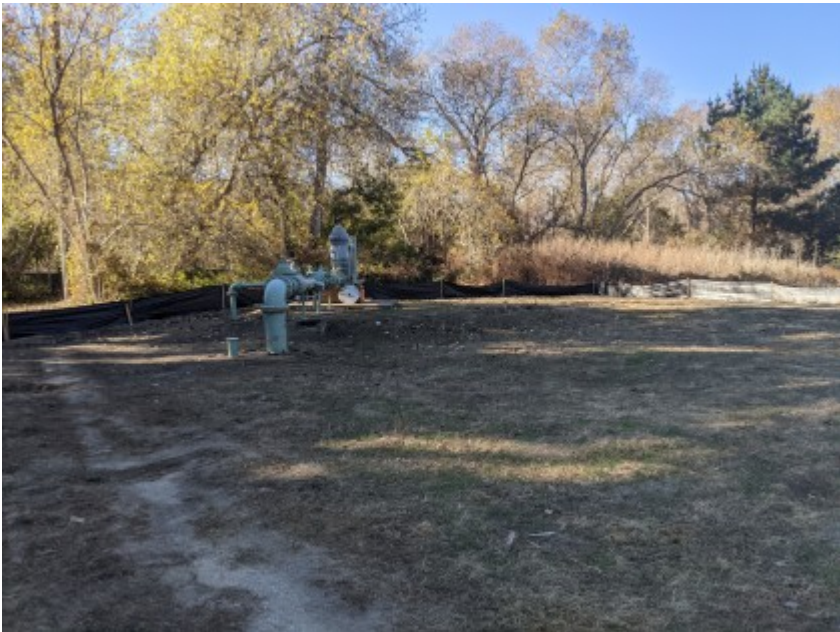
12/07/2020 - Intact silt fencing surrounding work area.
