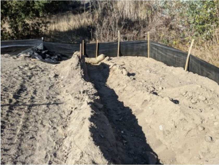
12/07/2020 - Intact silt fencing surrounding work area.
