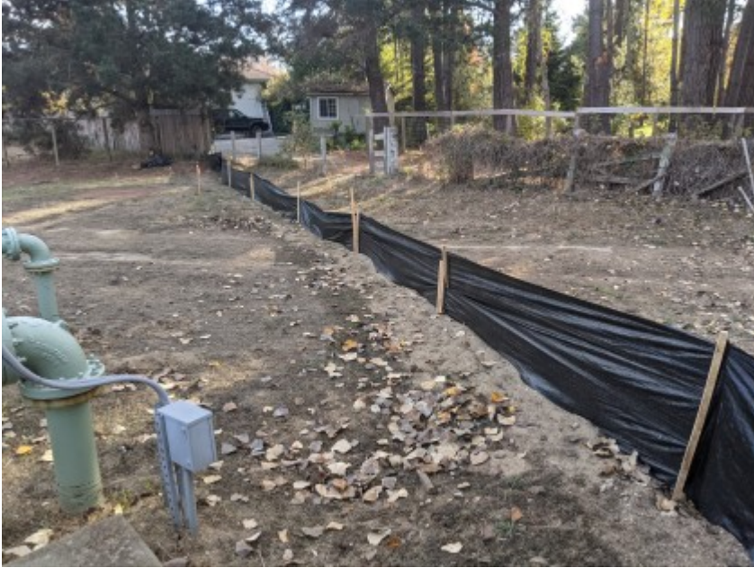
12/10/2020 - Intact silt fencing surrounding work area.
