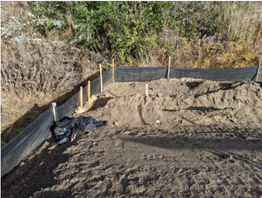
12/14/2020 - Intact exclusionary fencing surrounding work area.
