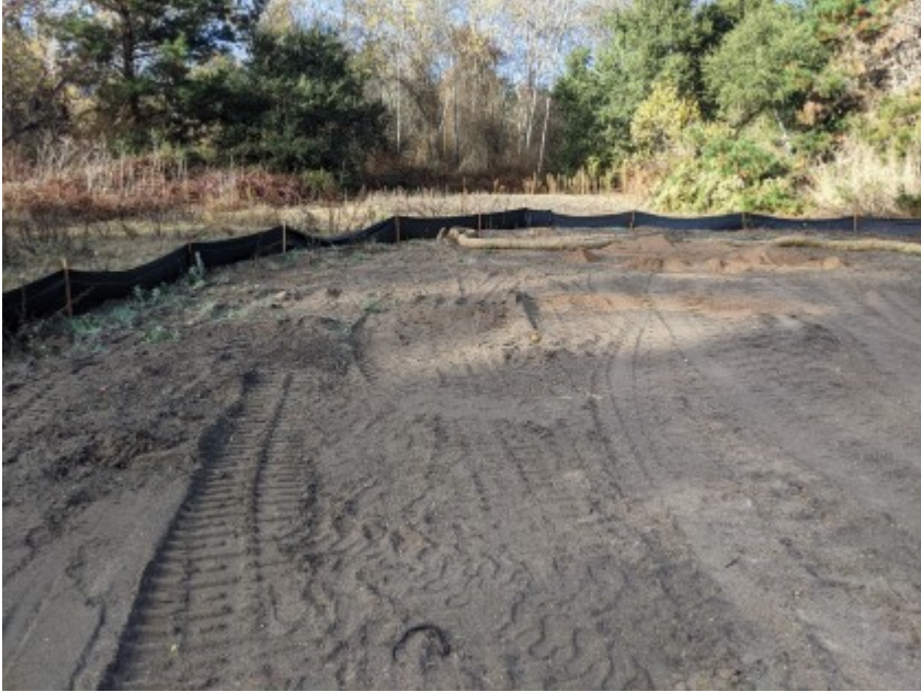
12/14/2020 - Intact exclusionary fencing surrounding work area.
