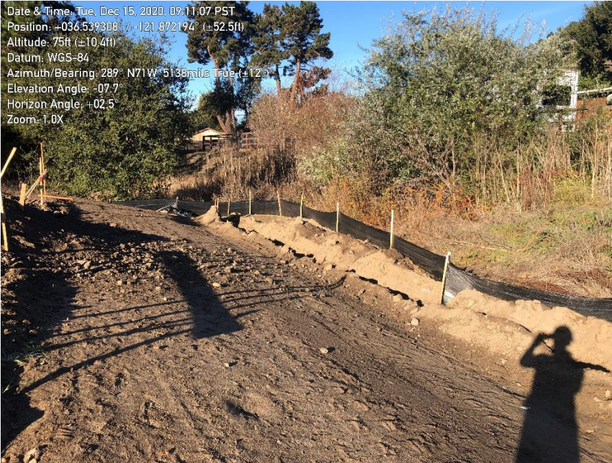
Photo 1. Silt fence near pad.
