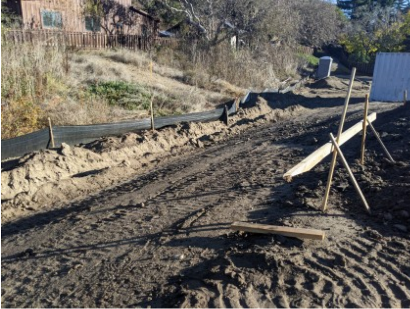
12/15/2020 - Intact exclusionary fencing surrounding work area.
