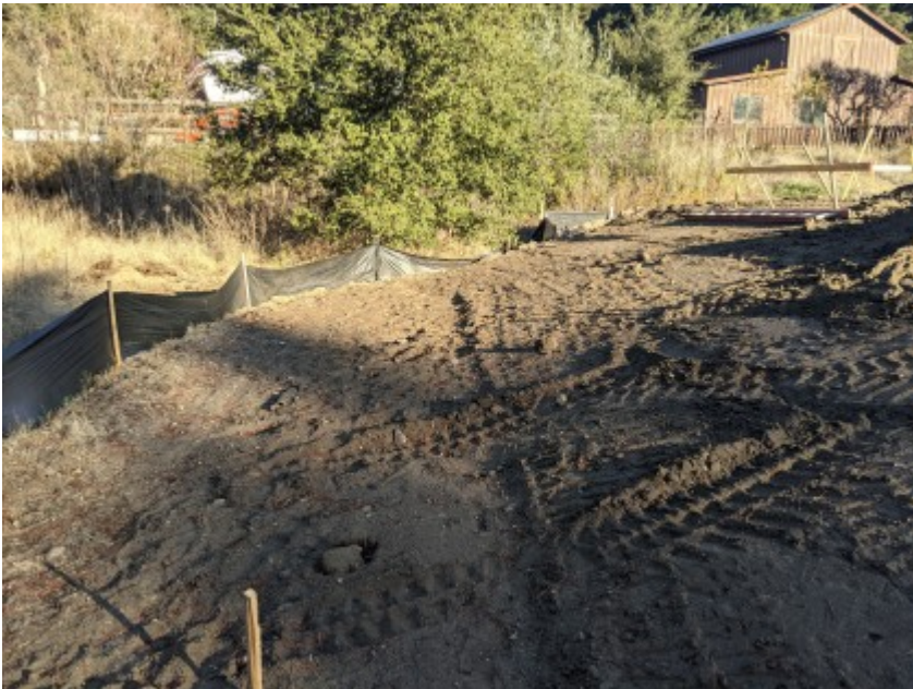
12/15/2020 - Intact exclusionary fencing surrounding work area.
