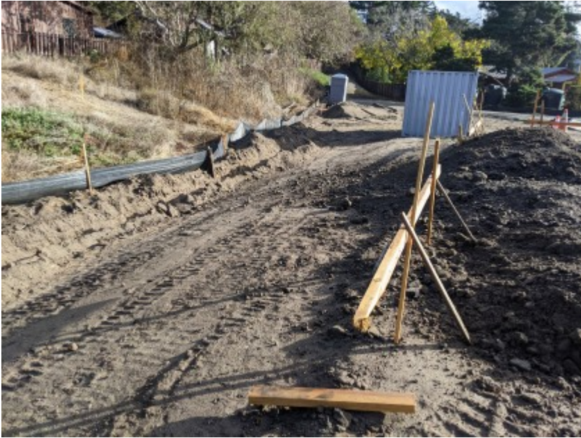
12/14/2020 - Intact exclusionary fencing surrounding work area.
