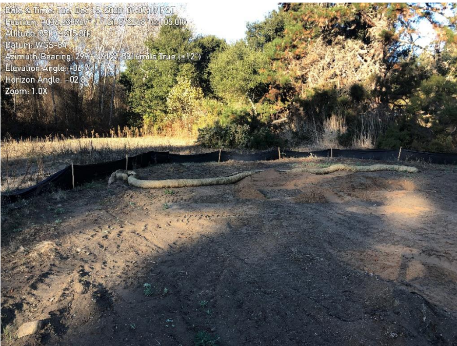
Photo 2. Silt fence at south end of side.
