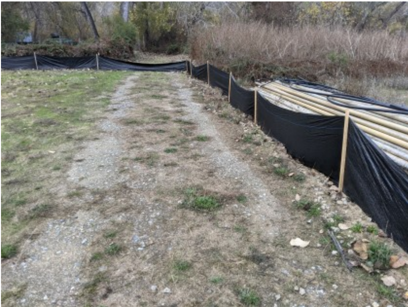
12/22/2020 - 10. Repaired exclusionary fencing surrounding work area.
