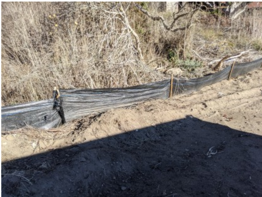
12/21/2020 - 2. Repaired exclusionary fencing surrounding work area.
