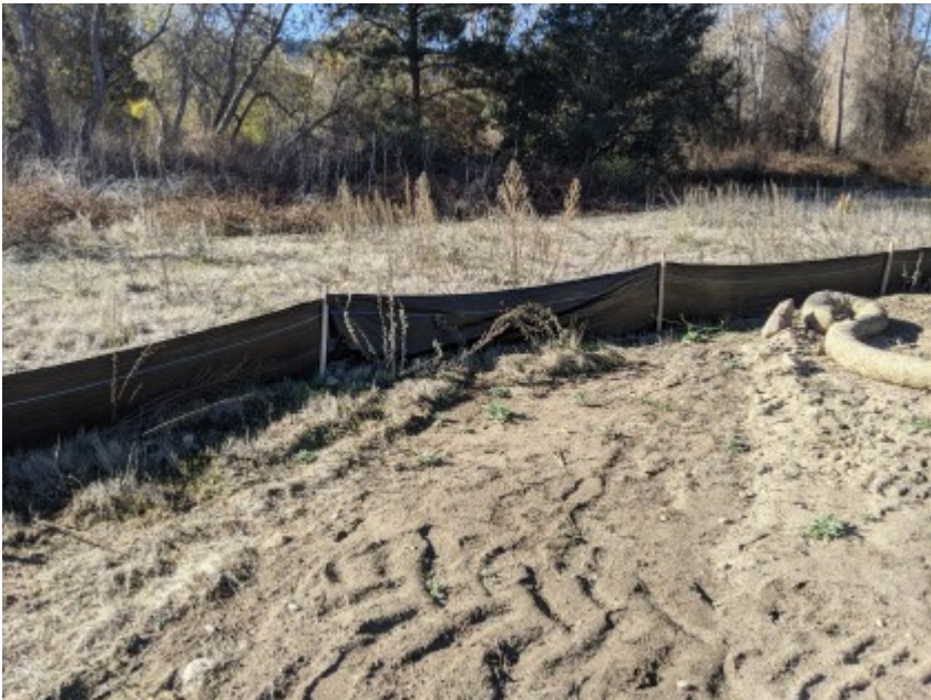
12/21/2020 - 4. Repaired exclusionary fencing surrounding work area.
