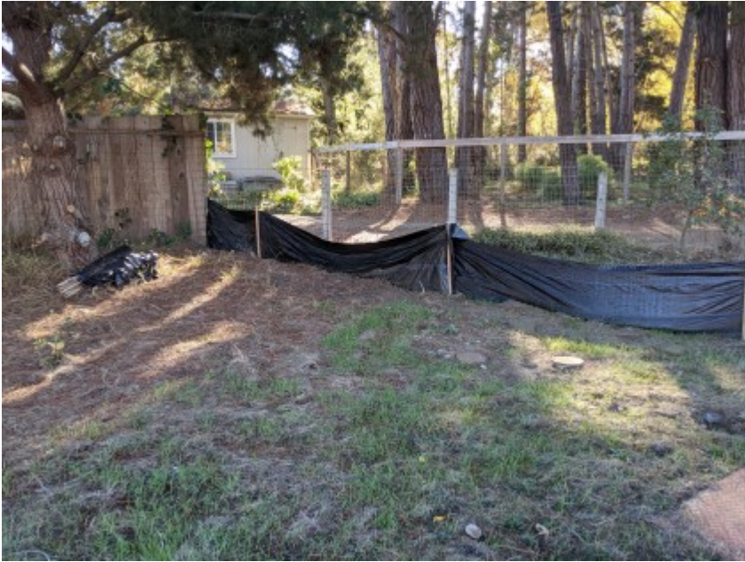
12/21/2020 - 5. Exclusionary fencing in need of repair.
