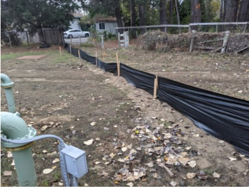
12/22/2020 - 9. Repaired exclusionary fencing surrounding work area.
