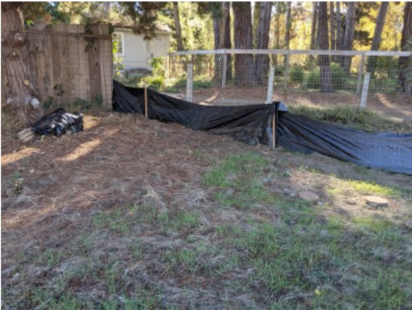
12/21/2020 - 6. Repaired exclusionary fencing surrounding work area.
