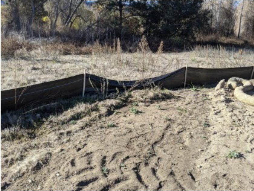
12/21/2020 - 3. Exclusionary fencing in need of repair.
