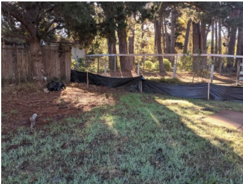
12/29/2020 - Intact exclusionary fencing surrounding work area.
