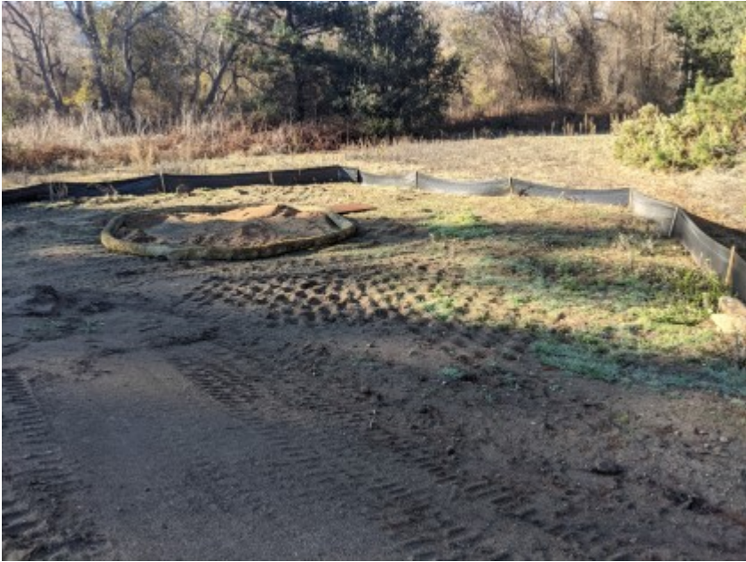
12/29/2020 - Intact exclusionary fencing surrounding work area.
