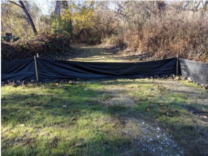
12/29/2020 - Intact exclusionary fencing surrounding work area.
