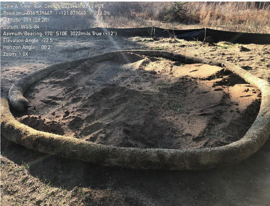
Photo 3. BMPs in place around fill stored onsite.
