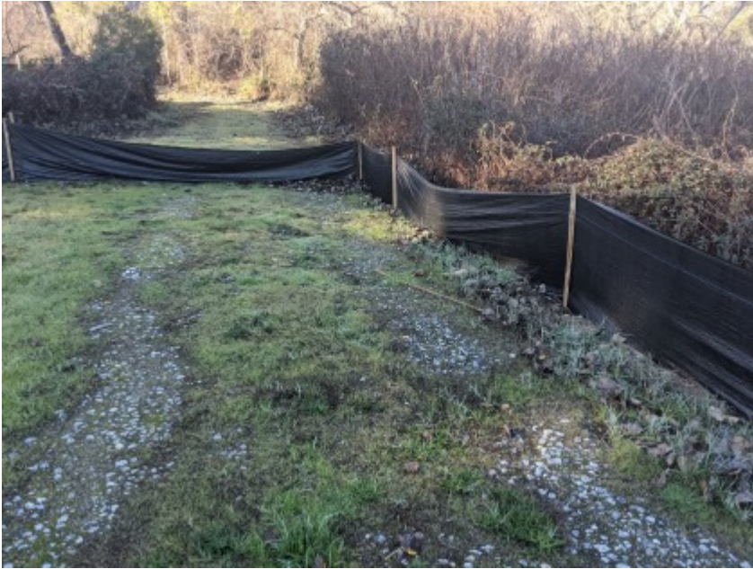
02/03/2021 - Intact exclusionary fencing surrounding work area.
