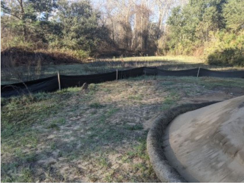
02/03/2021 - Intact exclusionary fencing surrounding work area.
