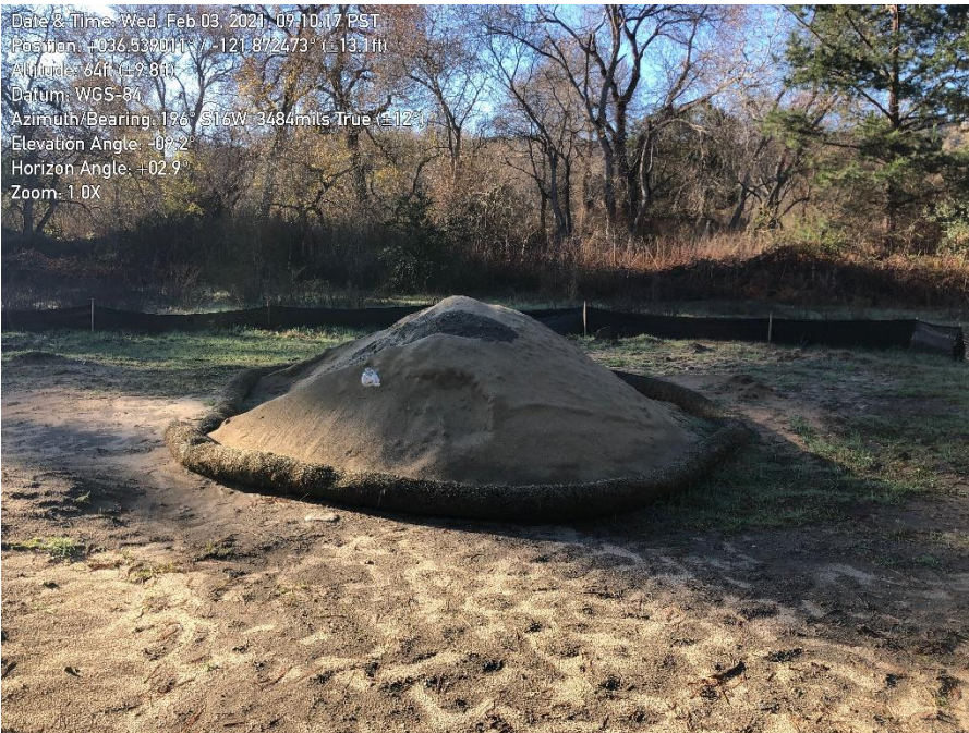
Photo 4. BMPs in place around stock pile.
