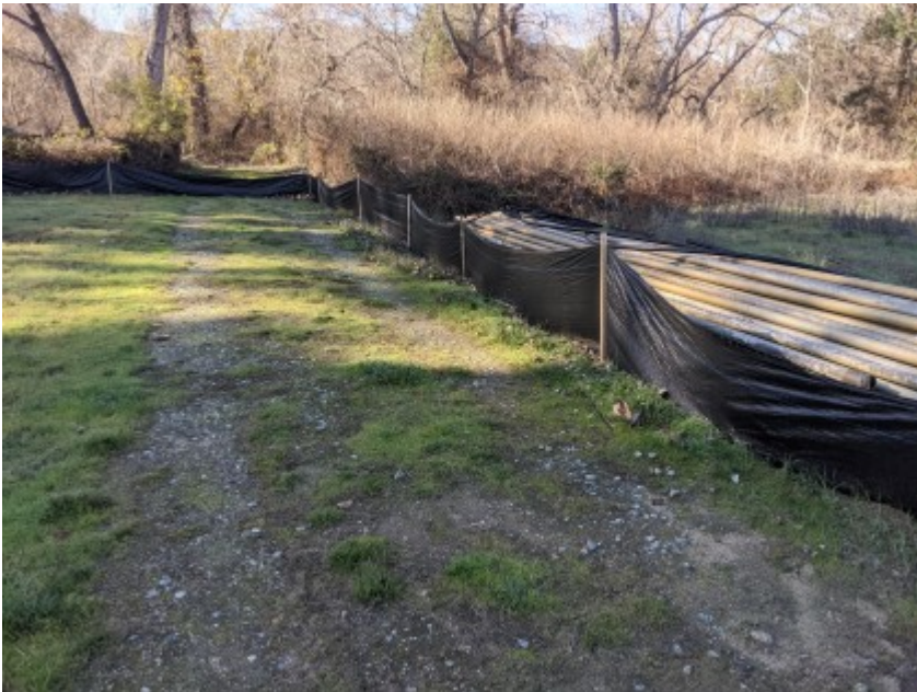
02/01/2021 - Intact exclusionary fencing surrounding work area.
