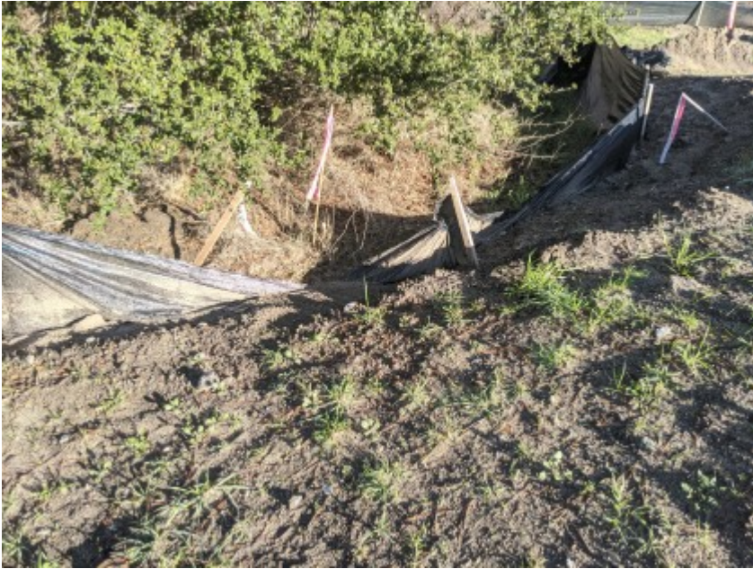
02/03/2021 - Section of exclusionary fencing damaged by erosional feature.
