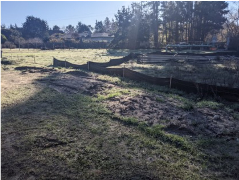
02/03/2021 - Intact exclusionary fencing surrounding work area.
