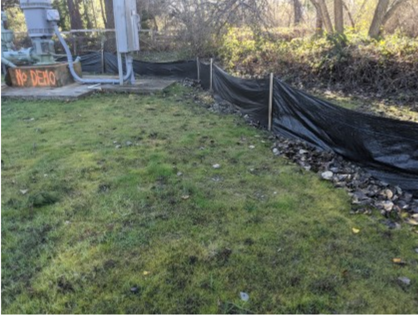
02/01/2021 - Intact exclusionary fencing surrounding work area.
