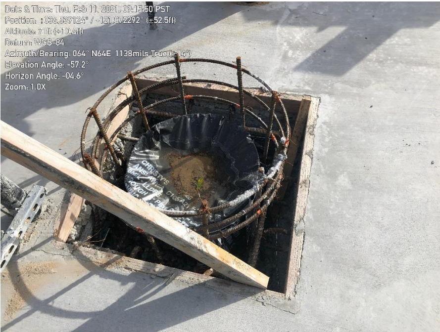
Photo 4. Wooden stakes placed in openings on slab.
