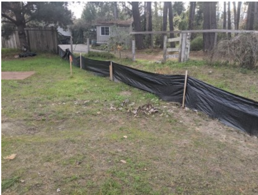
02/09/2021 - Intact exclusionary fencing surrounding work area.
