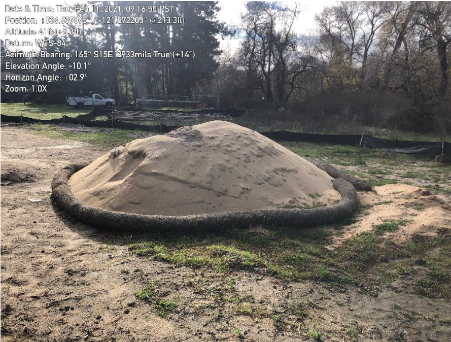
Photo 4. BMPs in place around stock pile.
