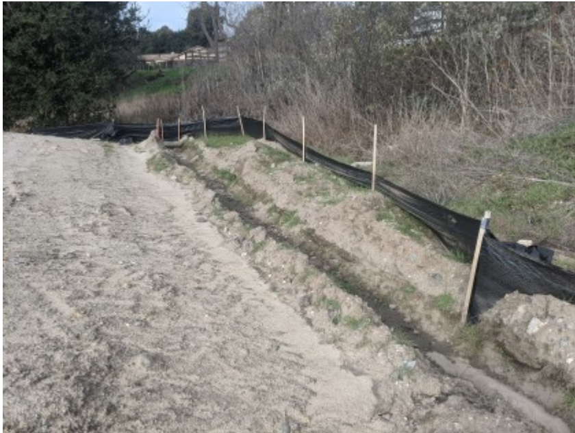
02/09/2021 - Intact exclusionary fencing surrounding work area.
