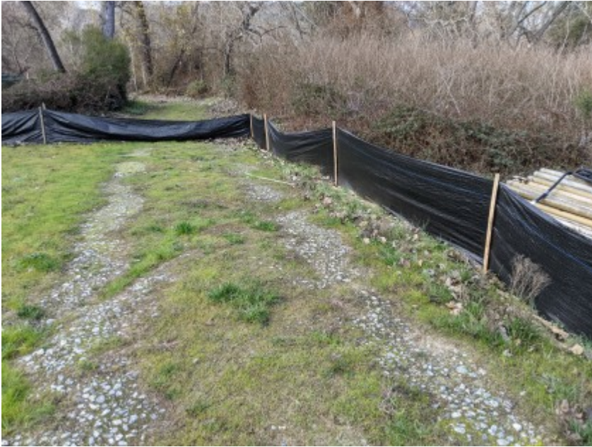
02/11/2021 - Intact exclusionary fencing surrounding work area.
