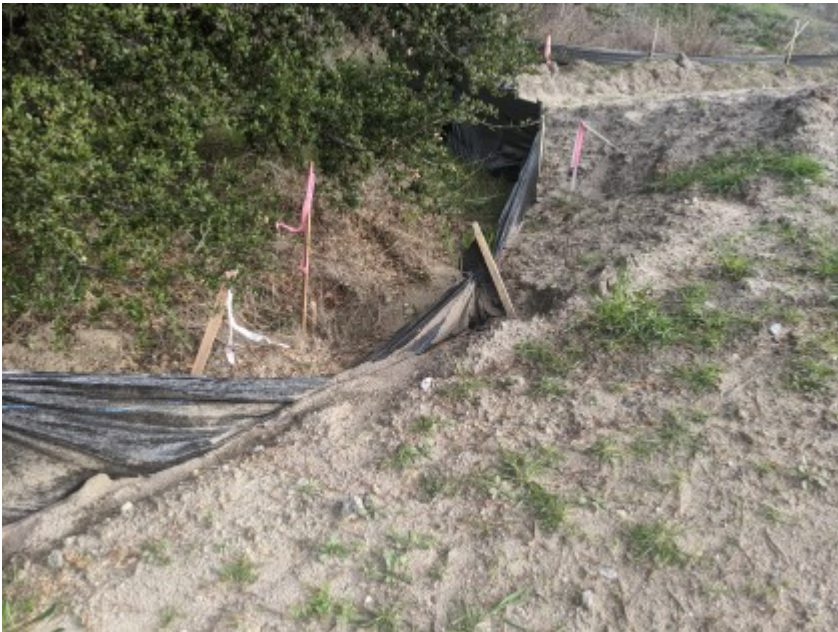
02/09/2021 - Section of exclusionary fencing damaged by erosional feature.
