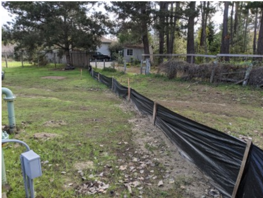
02/11/2021 - Intact exclusionary fencing surrounding work area.
