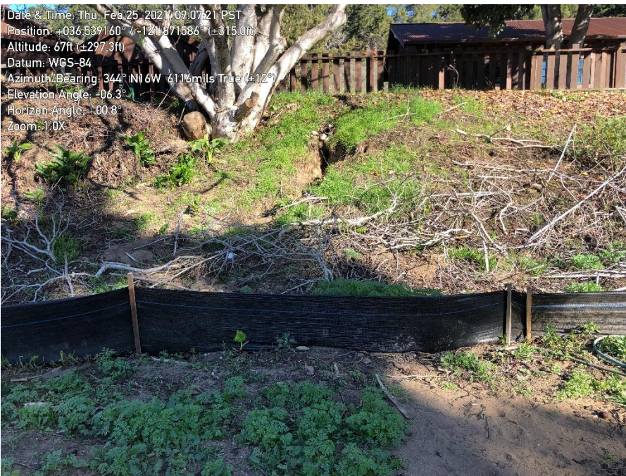
Photo 2. Silt fence repaired after being compromised due to erosion.
