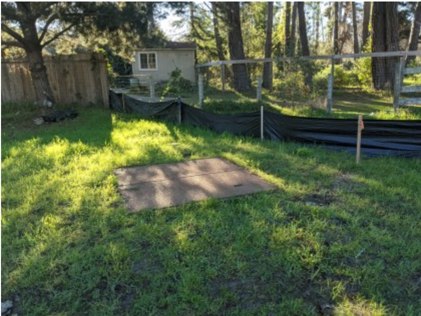
02/22/2021 - Intact exclusionary fencing surrounding work area.
