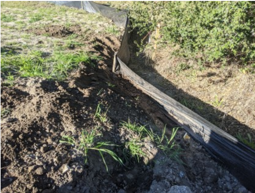
02/22/2021 - Eroded soil cleared from exclusionary fencing surrounding work area.
