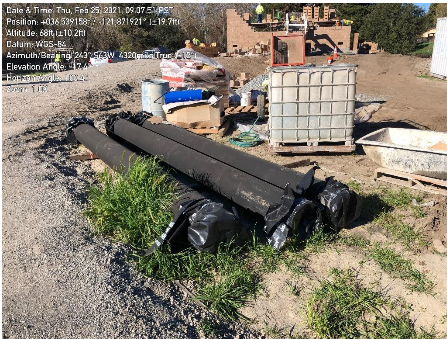
Photo 3. Pipes capped.
