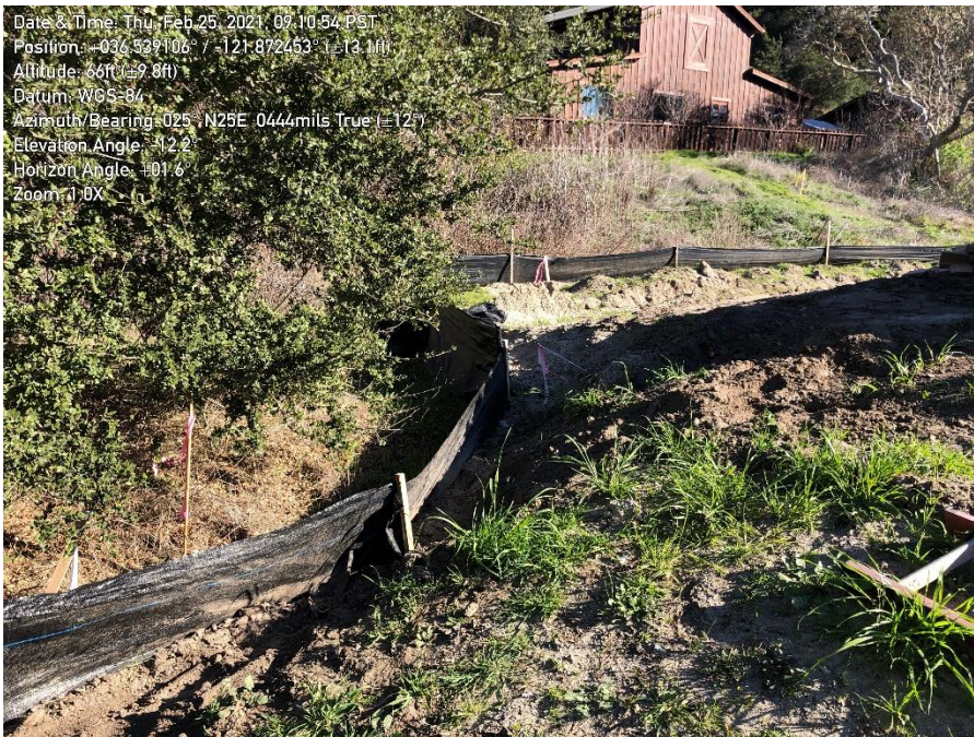
Photo 4. Silt fence along west border repaired.
