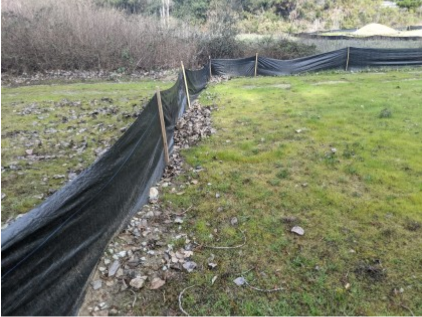
02/23/2021 - Intact exclusionary fencing surrounding work area.
