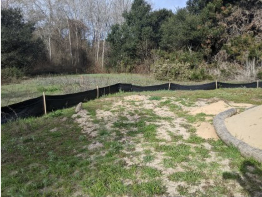
02/23/2021 - Intact exclusionary fencing surrounding work area.
