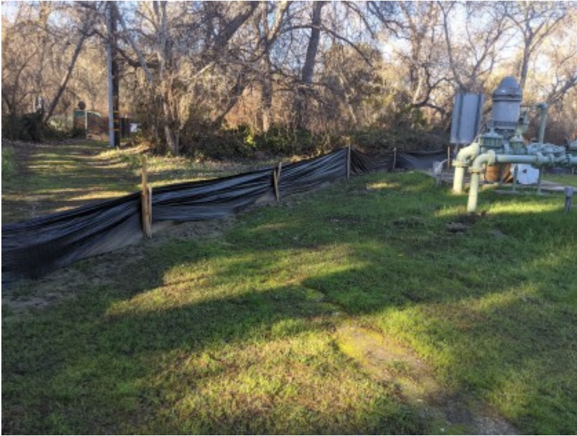
02/22/2021 - Intact exclusionary fencing surrounding work area.
