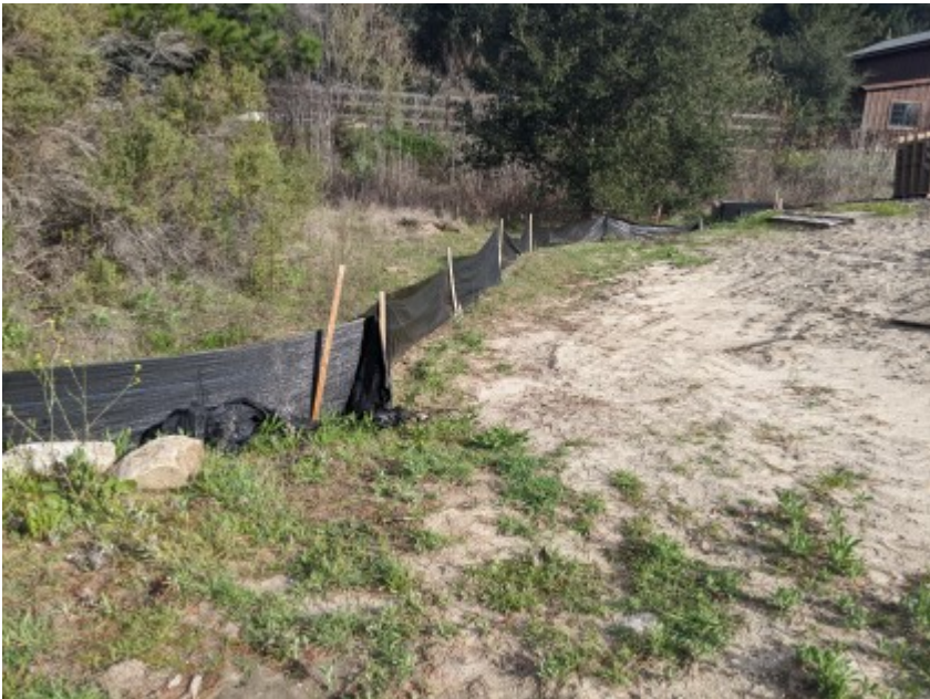
02/23/2021 - Intact exclusionary fencing surrounding work area.
