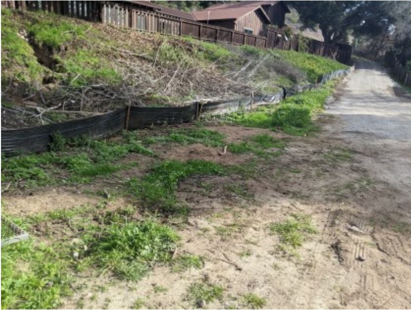
02/25/2021 - Confirmed repair of damaged exclusionary fencing surrounding work area.
