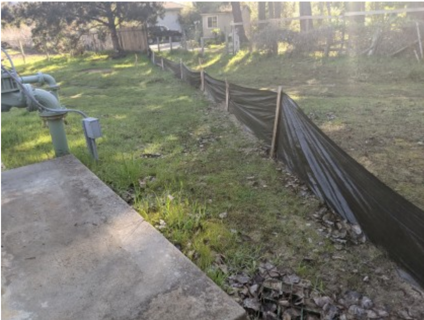
03/04/2021 - Intact exclusionary fencing surrounding work area.
