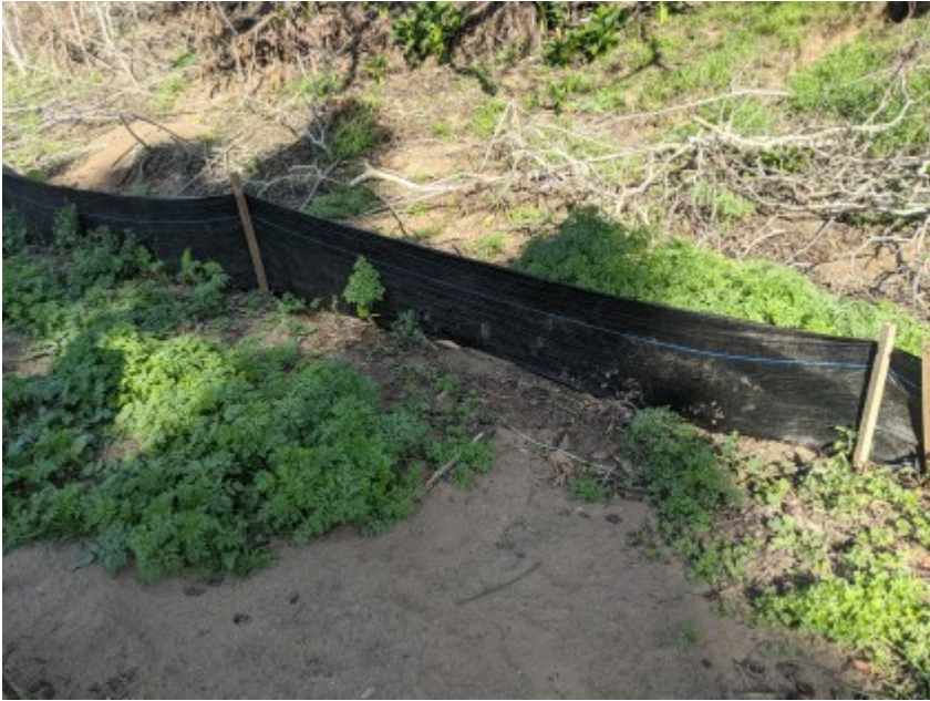
03/04/2021 - Intact exclusionary fencing surrounding work area.
