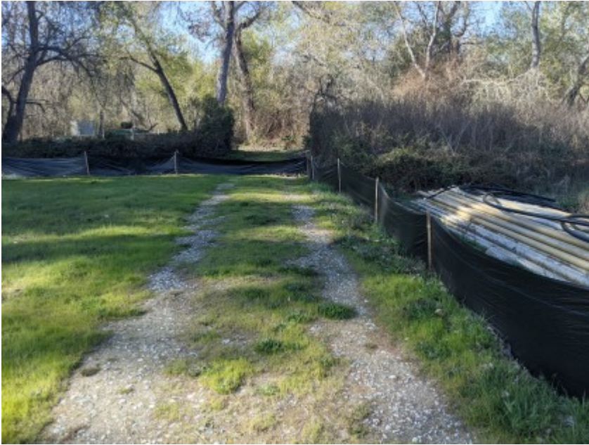
03/04/2021 - Intact exclusionary fencing surrounding work area.
