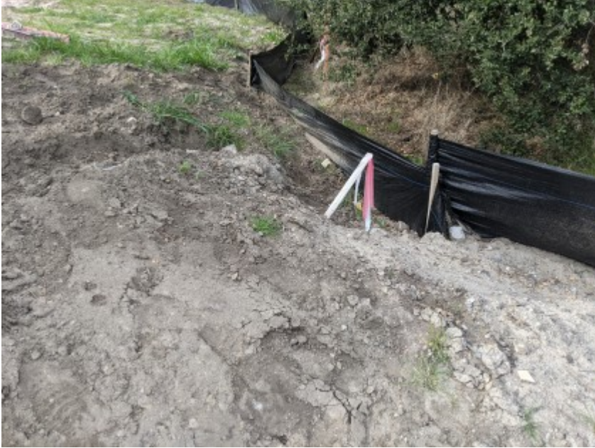
03/03/2021 - Intact exclusionary fencing surrounding work area.
