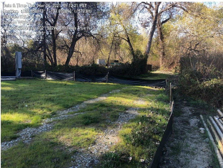
Photo 2. Exclusionary silt fence in acceptable condition.
