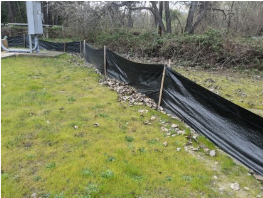
03/03/2021 - Intact exclusionary fencing surrounding work area.
