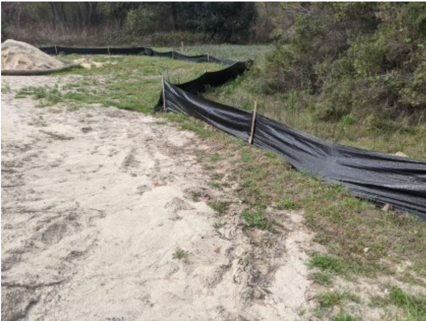
03/03/2021 - Intact exclusionary fencing surrounding work area.
