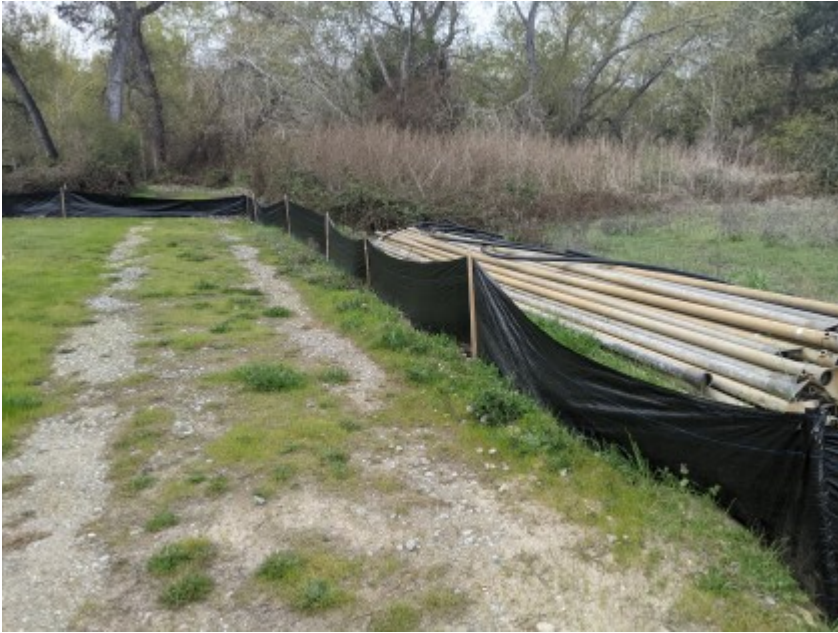
03/03/2021 - Intact exclusionary fencing surrounding work area.
