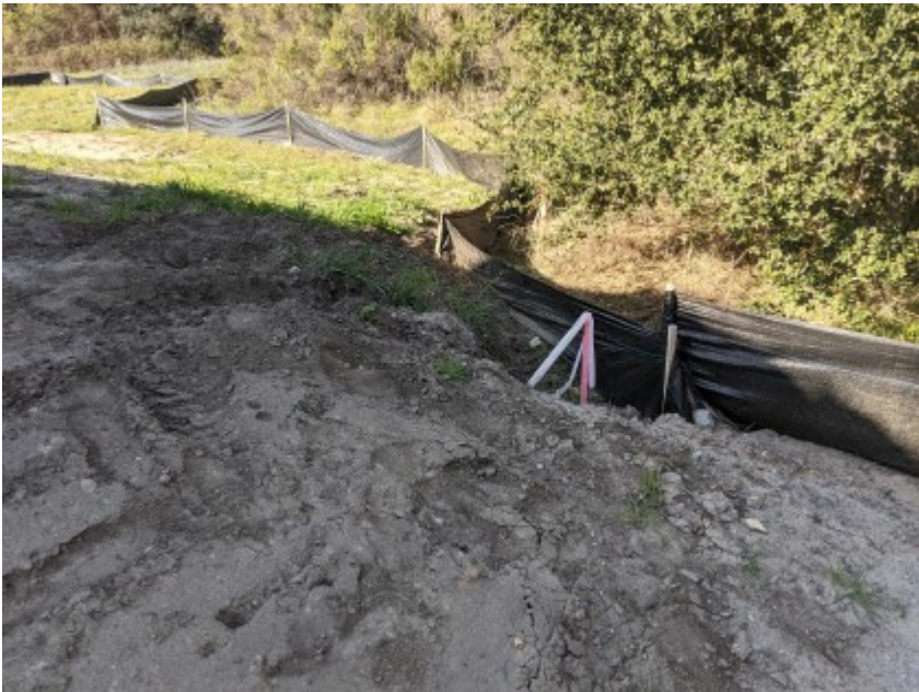
03/04/2021 - Intact exclusionary fencing surrounding work area.
